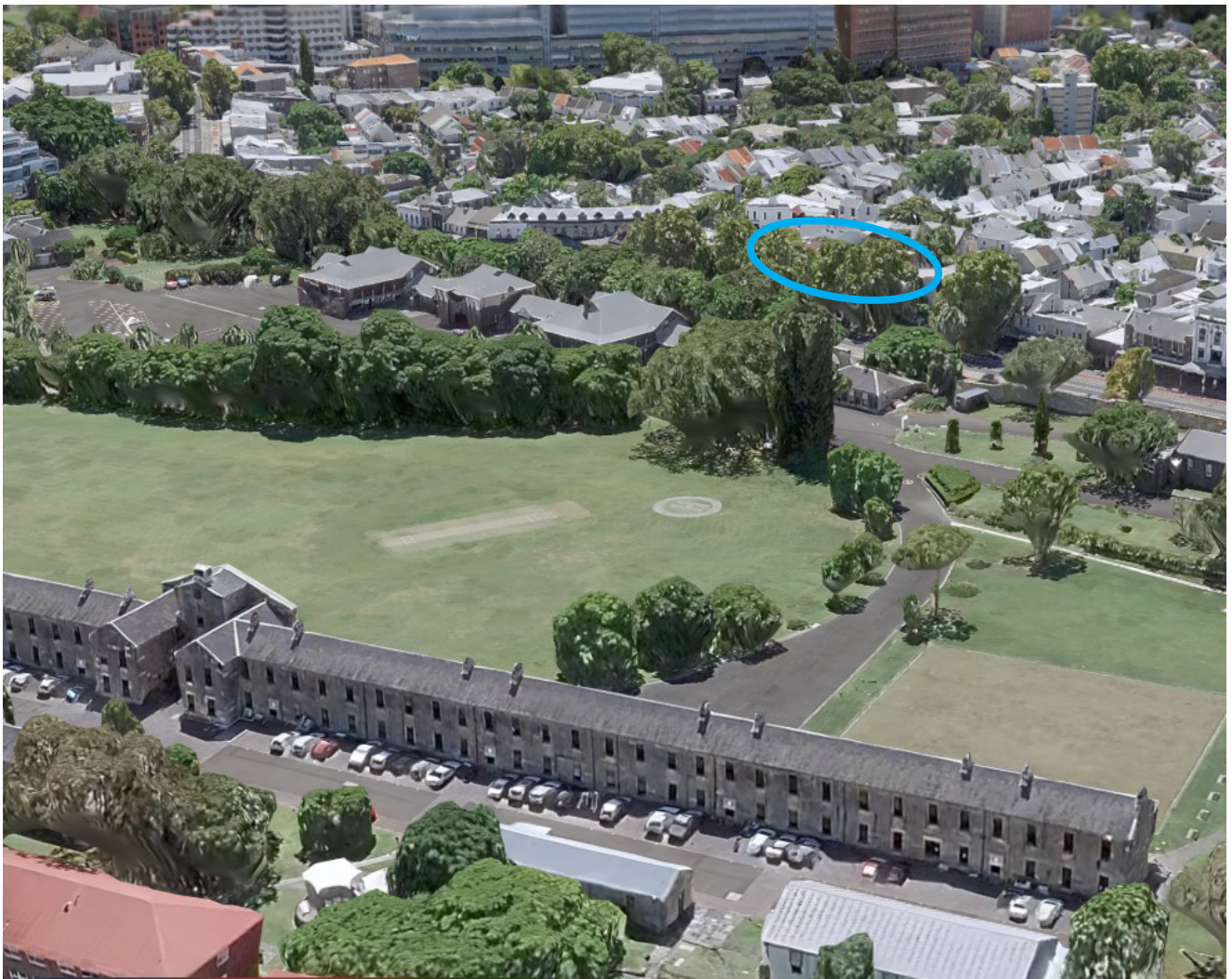
Figure 4.12 Oblique aerial photograph north-west over the Victoria Barracks towards the subject site, circled in blue. Note the multiple layers of trees between the parade ground and the subject site Source: Apple Maps
