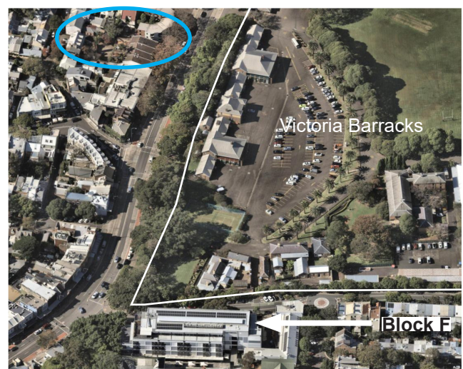
Figure 4.11 Oblique aerial photograph showing the relationship of the 5-storey Block F and the Victoria Barracks. The approximate extent of the perimeter wall is drawn in white Source: Nearmap website
