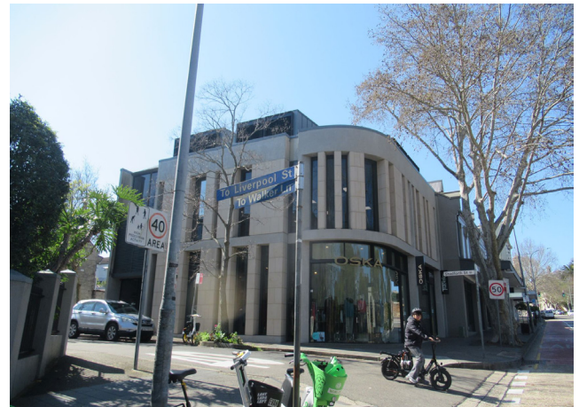
Figure 1.7 The three-storey retail building at 168 Oxford Street has a contemporary design and was constructed in recent decades
