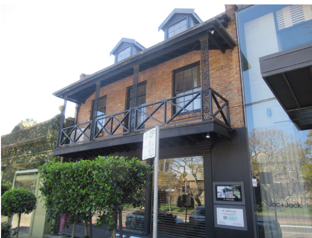
Figure 1.5 The commercial building at 124 Oxford Street, west of the subject site, emulated a historic residence but was constructed in recent decades
