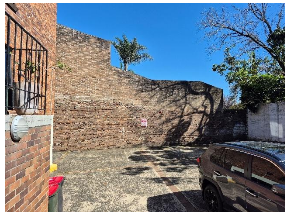
Figure 23. Carpark view west from the ramp.
