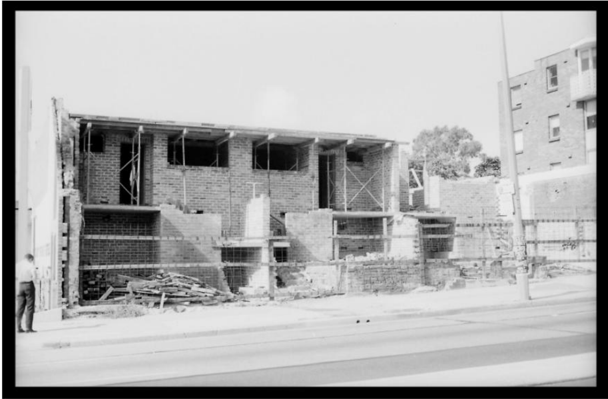
Figure 14. Construction of 142-148 Oxford Street in 1982 (National Trust).
