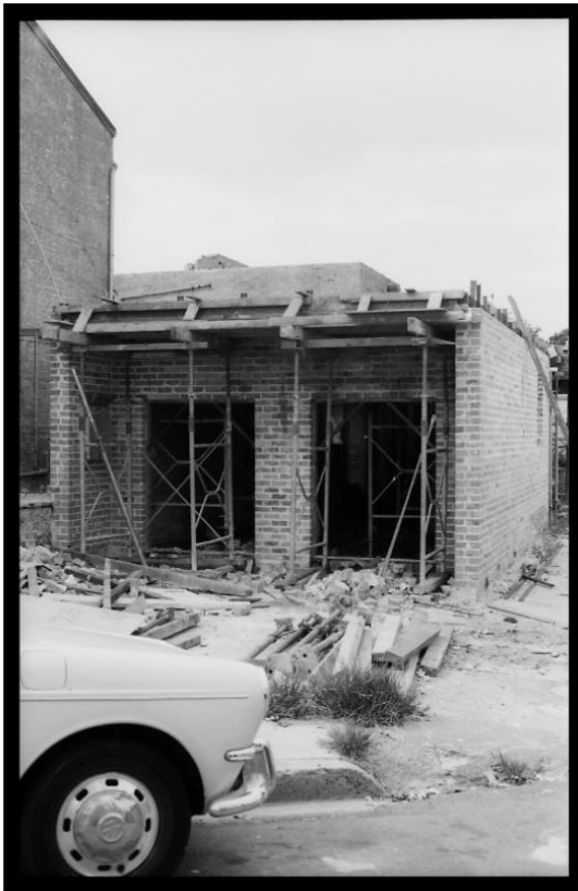
Figure 15. Construction of 13 Gipps Street in 1982 (National Trust).
