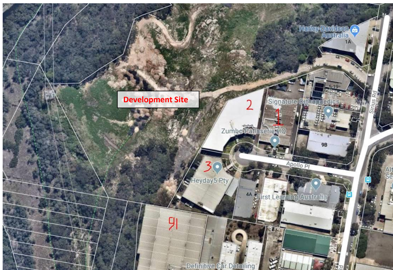
Figure 3 Neighbouring properties to 1 Sirius Rd Lane Cove
