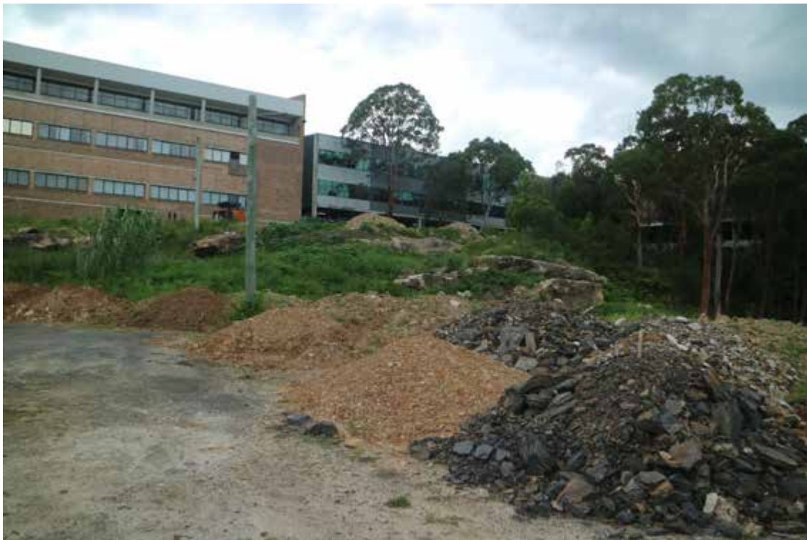
Plate 9 Contaminated fill dumped on site, view south-east
