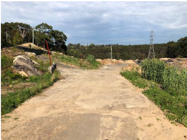
Photo 4. Tarred section of the access road.
