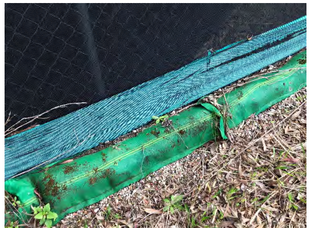
Photo 8. Sediment controls on the western boundary.
