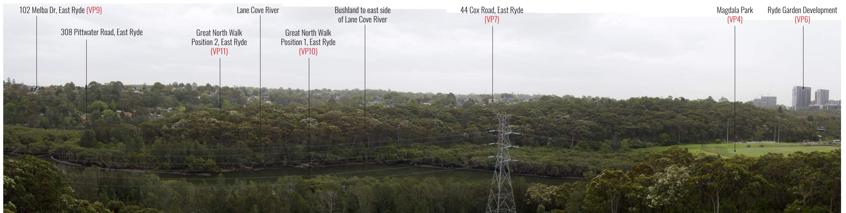
Figure 13: Drone at 40m RL Position 1 - Looking West
