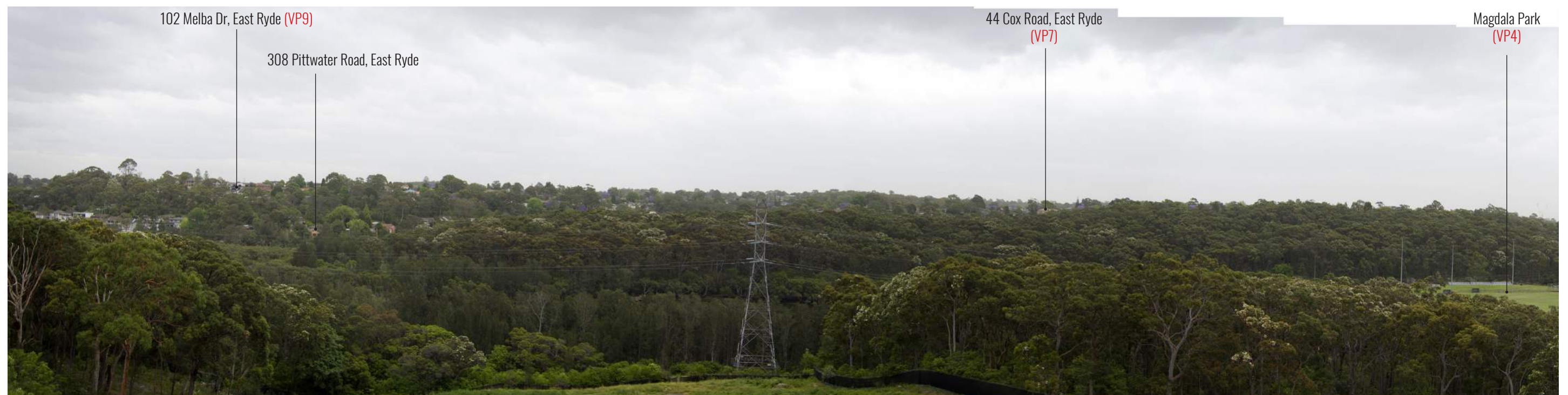
Figure 17: Drone at 40m RL Position 2 looking West
