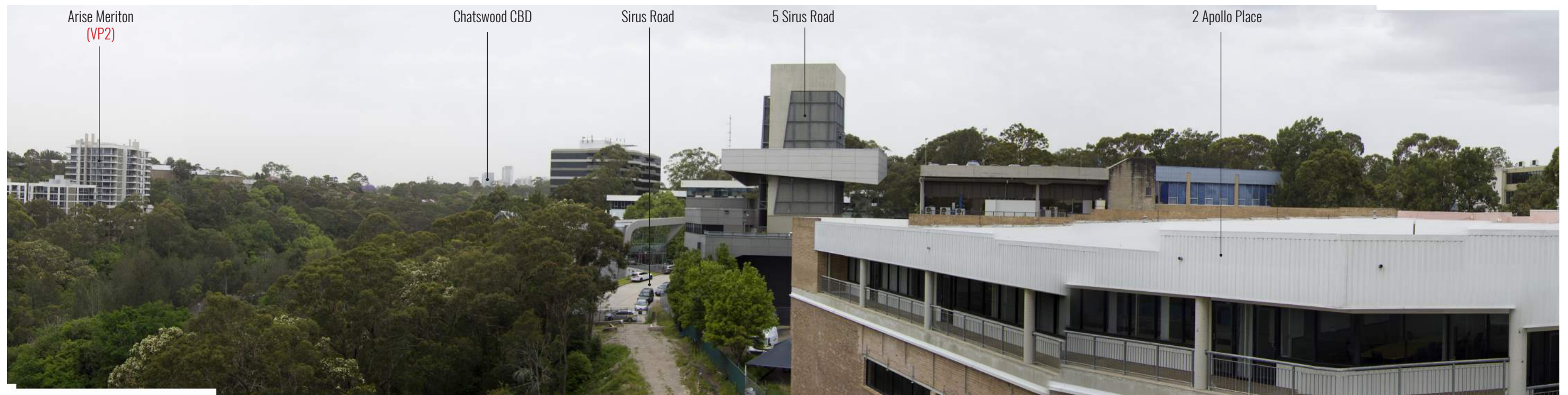
Figure 15: Drone at 40m RL Position 2 Looking - East
