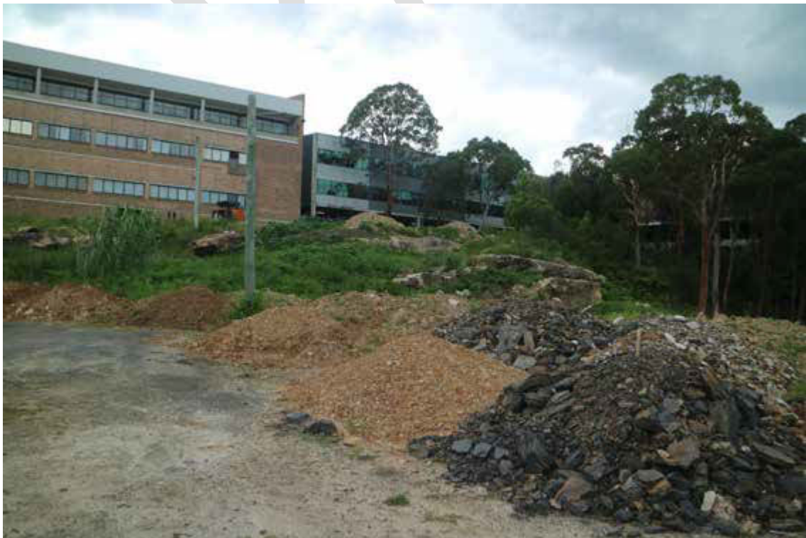
Plate 9 Contaminated fill dumped on site, view south-east
