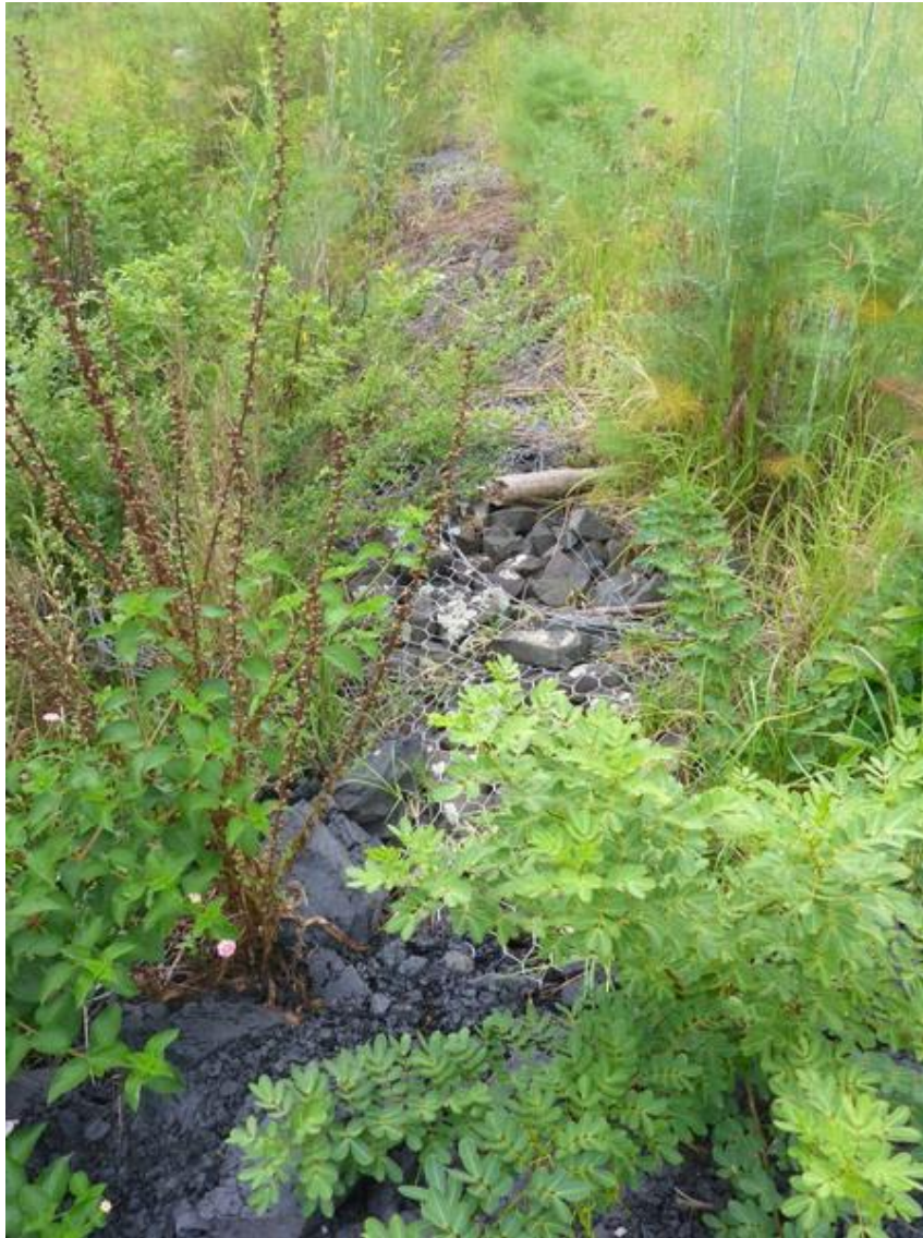
Plate 14 Loose rubble with wire netting running towards the north end of the site, facing north
