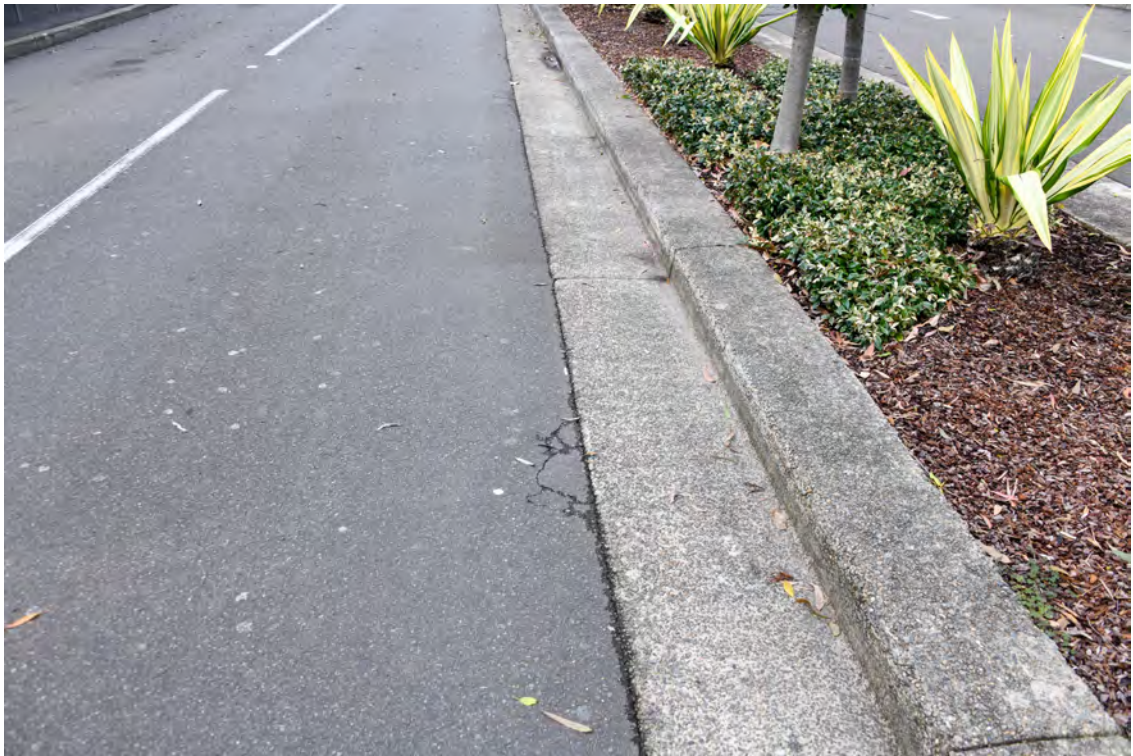
Eastern side of the Boulevard. Area opposite 'The Hordern Pavilion'. Area approaching the intersection with Park Road. Heading south. Cracked paving adjacent to the gutter.
