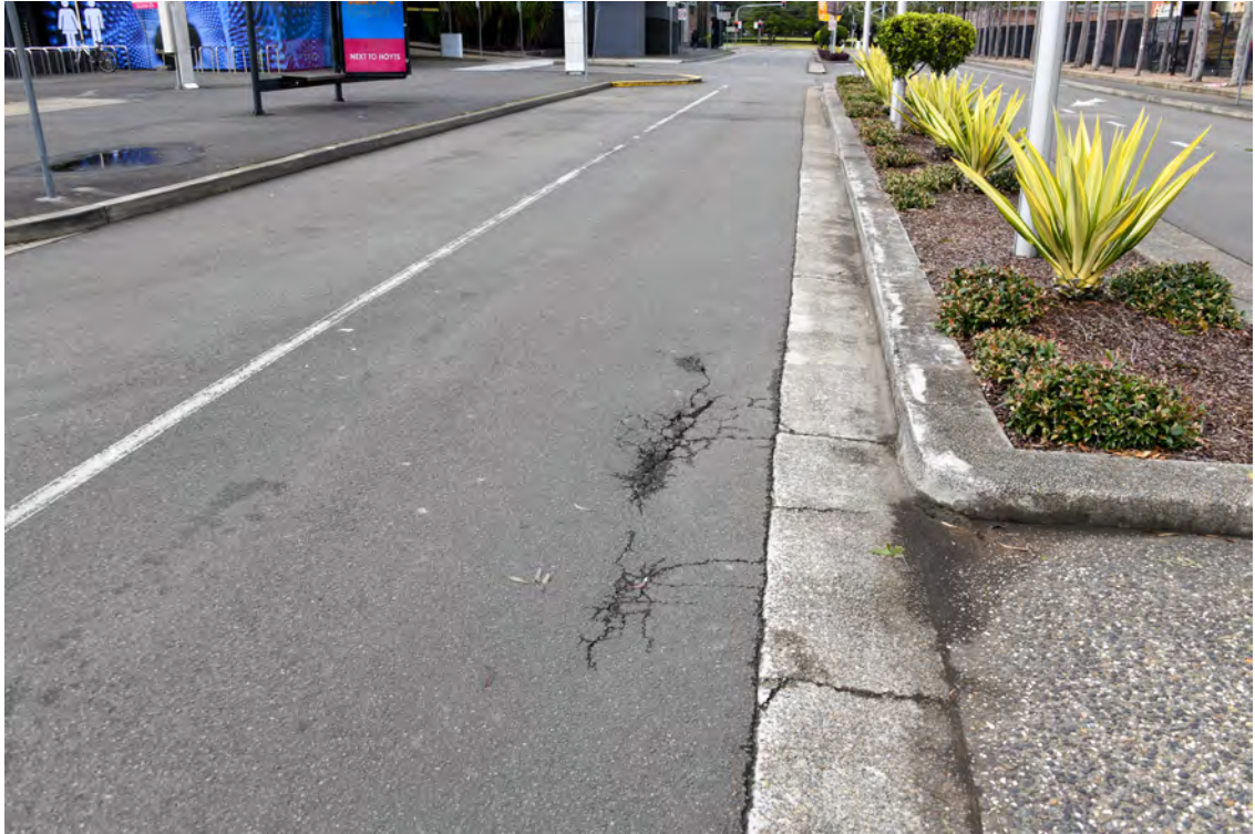
Eastern side of the Boulevard. Area opposite the area between 'The Hordern Pavilion' and 'The Royal Hall of Industries'. Intersection with Park Road. Heading south. Gap in the median strip. Cracked adjacent road paving.
