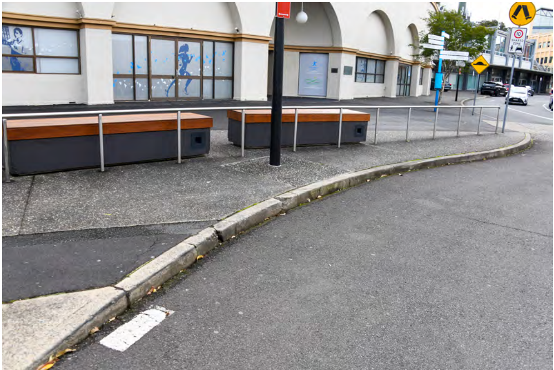
Roundabout at the northern end of the Boulevard. Heading clockwise. North-western side of the roundabout. Cracked and chipped kerb.
