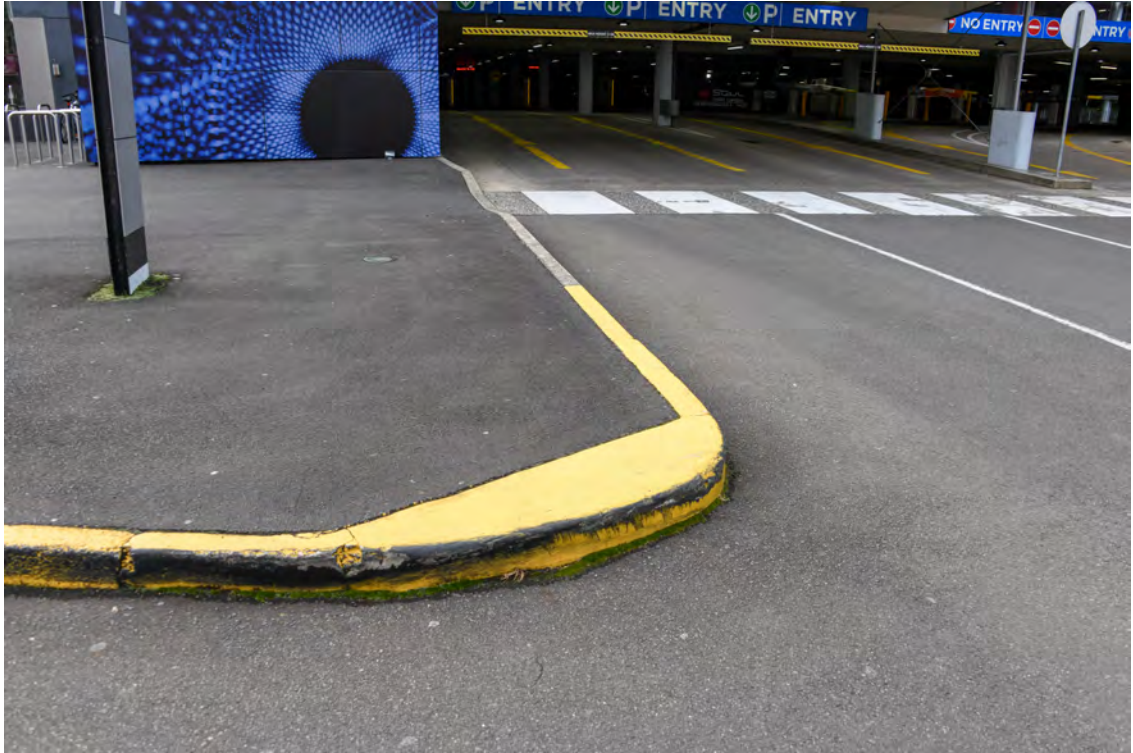
Eastern side of the Boulevard. Area opposite the 'The Royal Hall of Industries'. Area of the entry / exit to the 'Wilson Car Park'. Heading south. Chipped yellow painted kerb.
