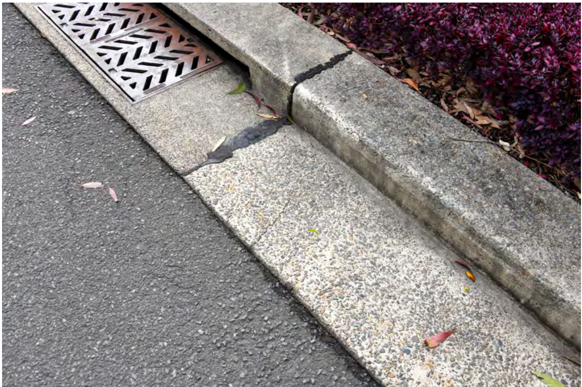
Western side of the Boulevard. Area adjacent to 'The Hordern Pavilion'. Area on the southern side of the roundabout. Cracked median strip gutter.
