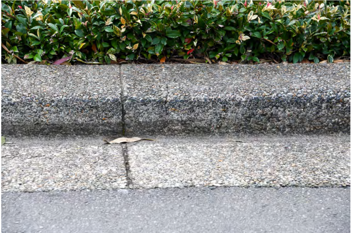
Western side of the Boulevard. Area adjacent to 'The Royal Hall of Industries'. Heading north. Area of the lid to the services pit in the road. Median strip. Cracked kerb.
