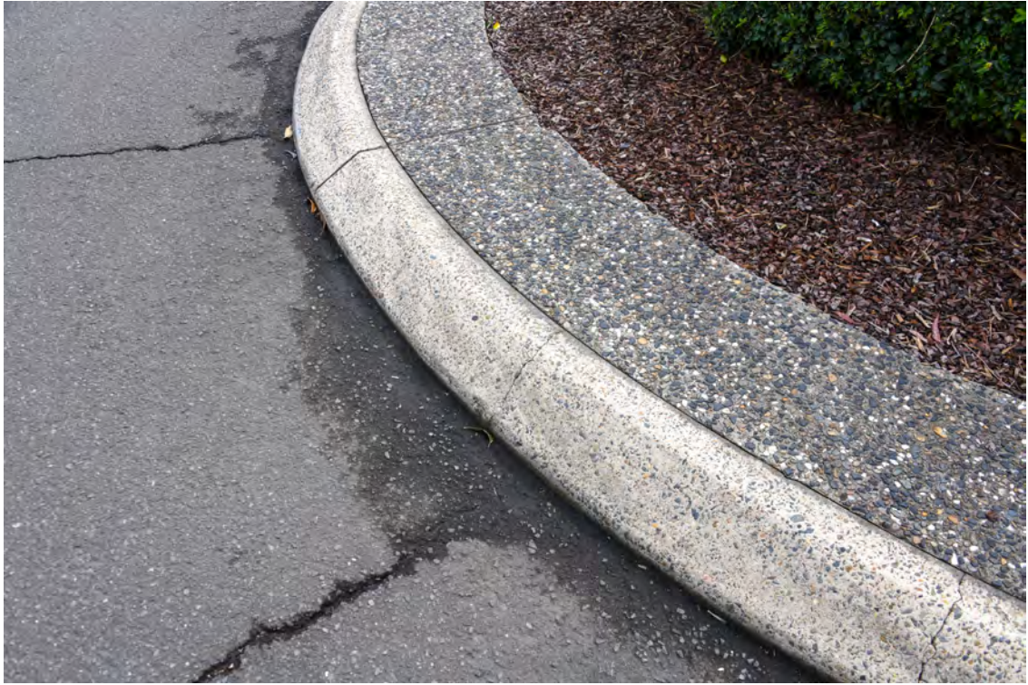
Roundabout at the northern end of the Boulevard. Heading clockwise around the centre of the roundabout. Western side. Cracked kerb.
