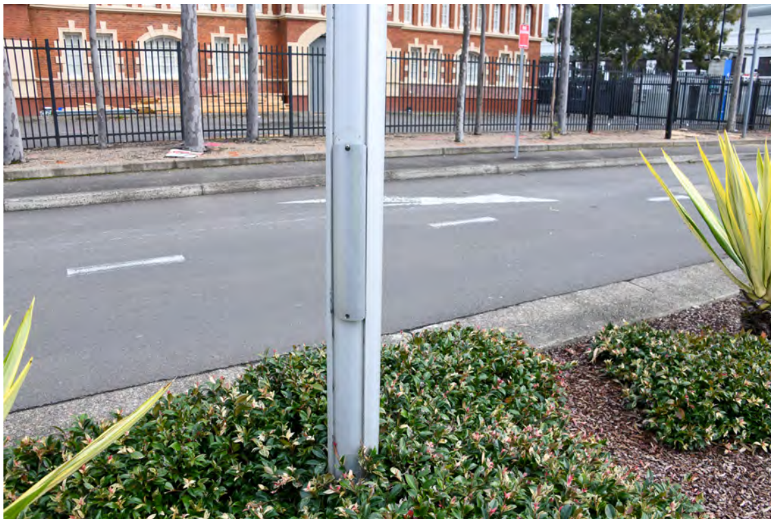
Eastern side of the Boulevard. Area opposite the 'The Royal Hall of Industries'. Area approaching the entry / exit to the 'Wilson Car Park'. Heading south along the median strip. Flagpole. Loose cover plate.
