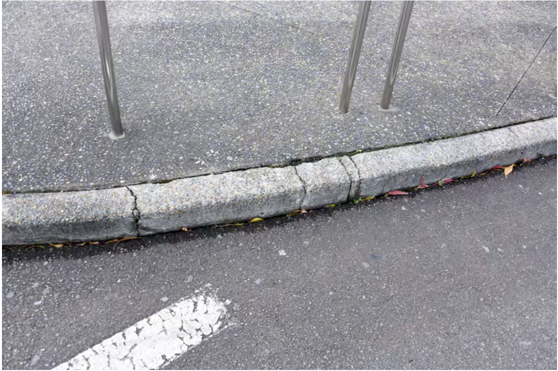
Roundabout at the northern end of the Boulevard. Eastern side of the roundabout. Heading clockwise. Cracked kerb.
