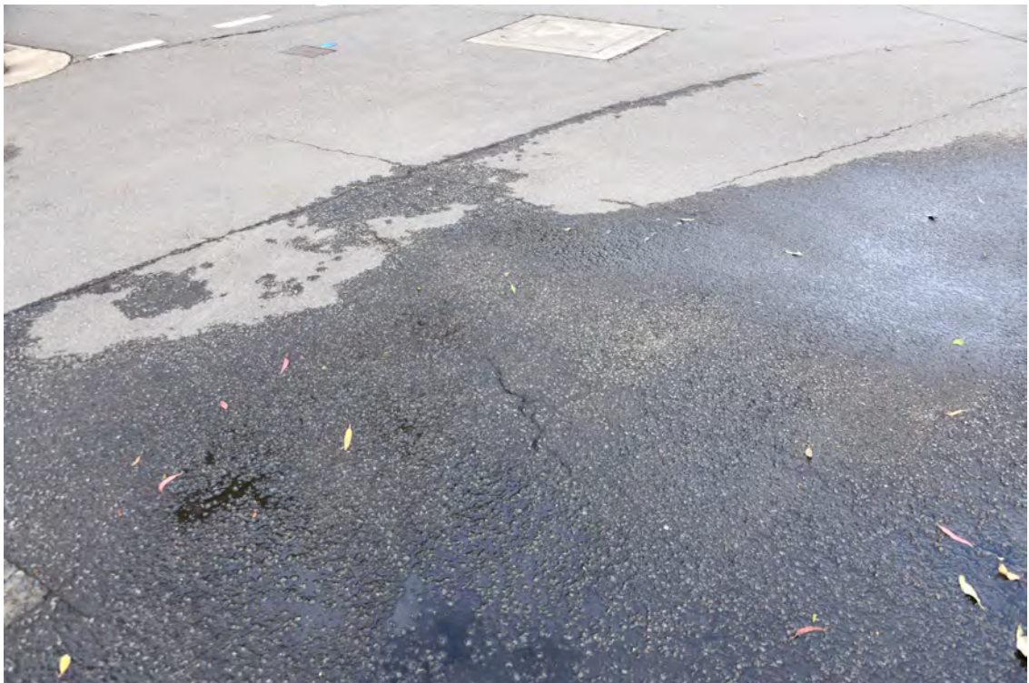
Roundabout at the northern end of the Boulevard. Southern side of the roundabout. Facing west. Cracked road paving.
