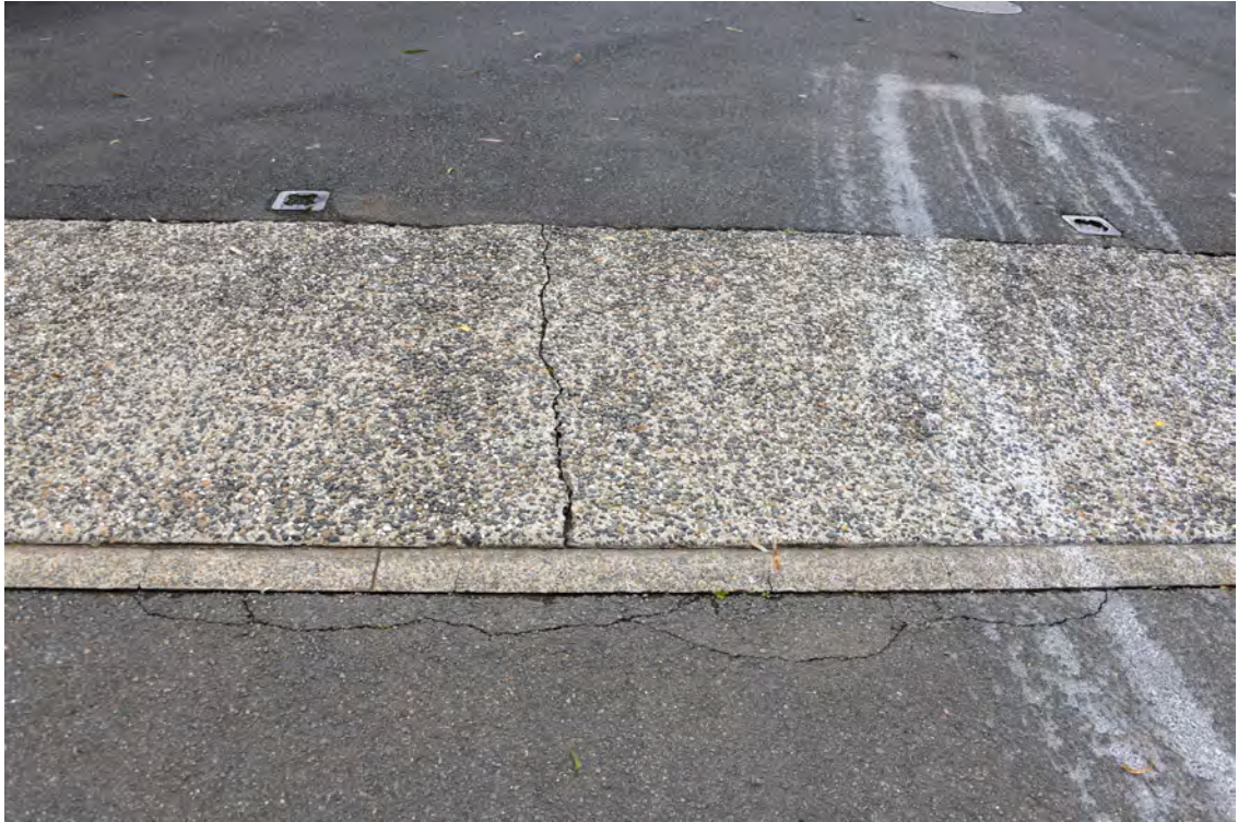
Eastern side of the Boulevard. Area opposite the area between 'The Hordern Pavilion' and 'The Royal Hall of Industries'. Intersection with Park Road. Heading south. Cracked paving.
