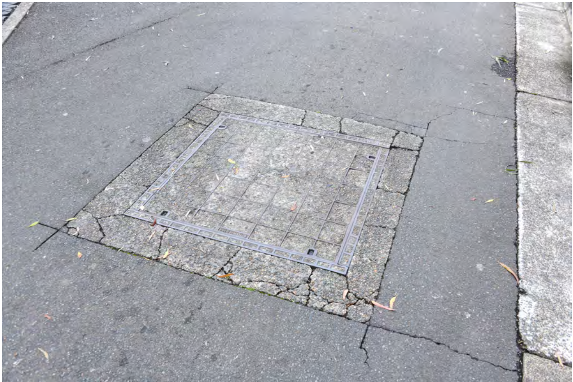
Eastern side of the Boulevard. Area opposite the area between 'The Hordern Pavilion' and 'The Royal Hall of Industries'. Area of the pedestrian crossing. Heading south. Lid to the services pit in the road. Cracked surrounding paving.
