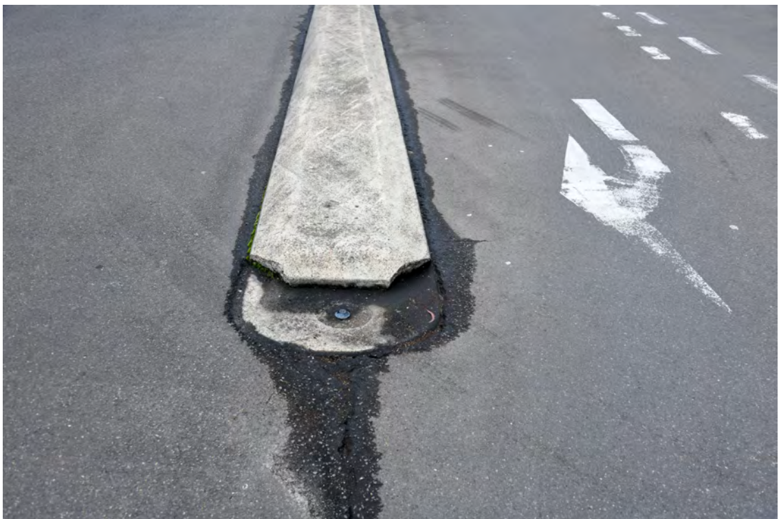
Eastern side of the Boulevard. Area opposite the 'The Royal Hall of Industries'. Area of the entry / exit to the 'Wilson Car Park'. Heading south. Chipped northern end of the median strip.
