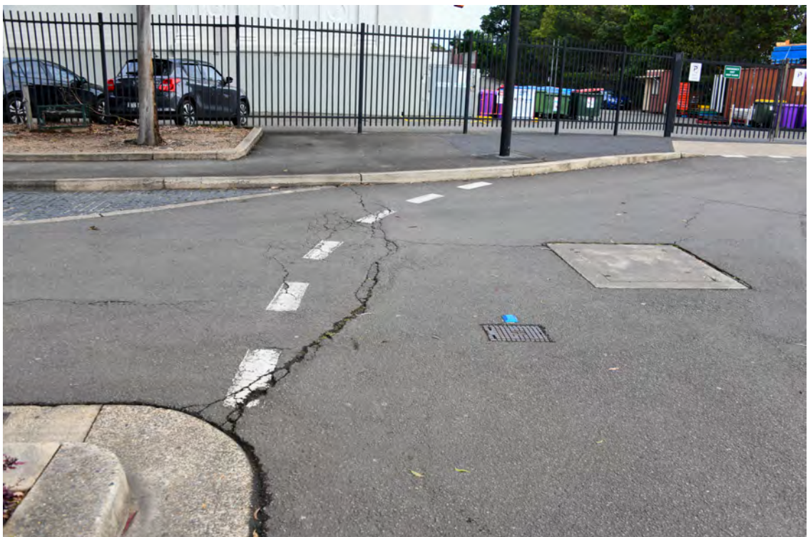
Western side of the Boulevard. Area adjacent to 'The Hordern Pavilion'. Area on the southern side of the roundabout. Facing west. Cracked road paving.
