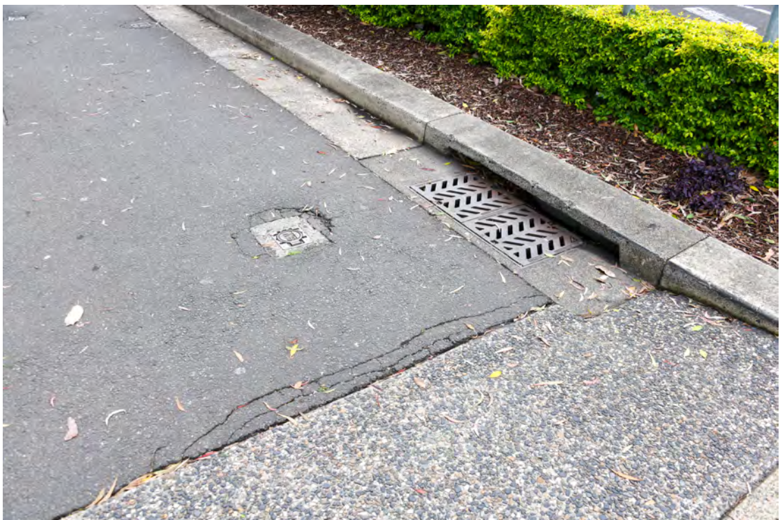
Western side of the Boulevard. Area adjacent to area between 'The Royal Hall of Industries' & 'The Hordern Pavilion'. Heading north. Area of the pedestrian crossing. Facing east. Cracked asphalt paving.
