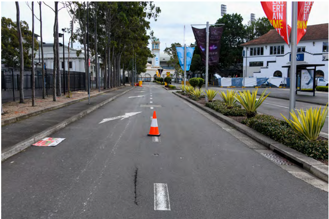
Western side of the Boulevard. Area adjacent to 'The Royal Hall of Industries'. Heading north. Area of the entry / exit to the 'Wilson Car Park'. Crack in the asphalt road paving.
