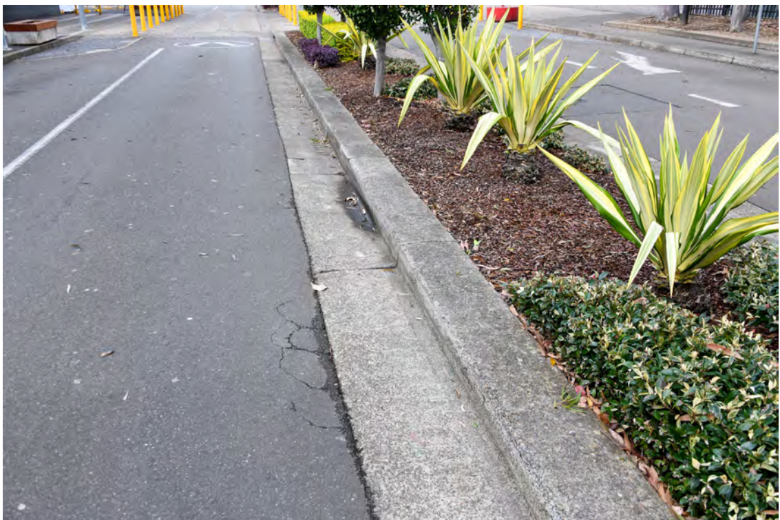
Eastern side of the Boulevard. Area opposite 'The Hordern Pavilion'. Area approaching the intersection with Park Road. Heading south. Cracked paving adjacent to the median strip.
