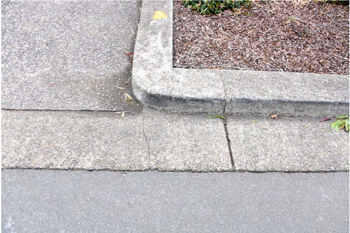
Western side of the Boulevard. Area adjacent to area between 'The Royal Hall of Industries' & 'The Hordern Pavilion'. Heading north. Intersection with Park Road. Median strip. Cracked kerb and gutter.
