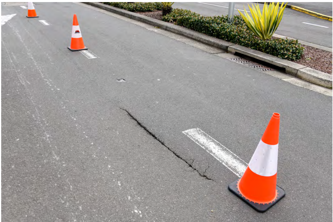
Western side of the Boulevard. Area adjacent to 'The Royal Hall of Industries'. Heading north. Crack in the asphalt road paving.
