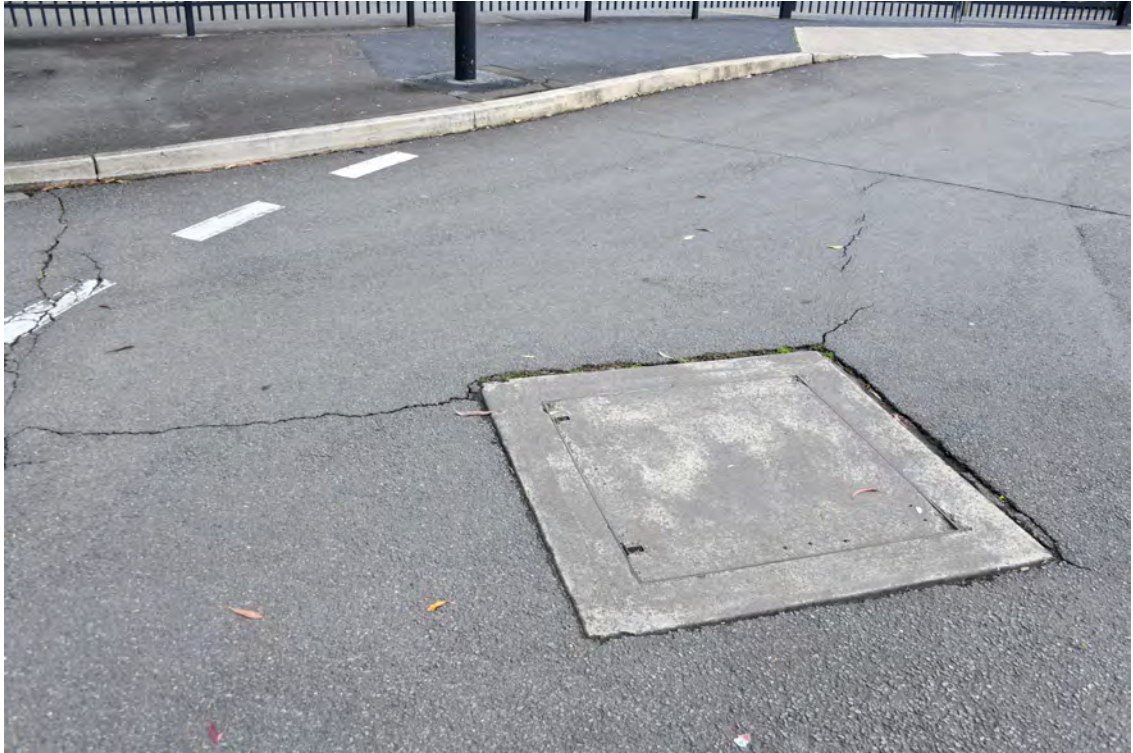
Roundabout at the northern end of the Boulevard. Heading clockwise. South-western side of the roundabout. Lids to the services in the road. Cracked adjacent paving.
