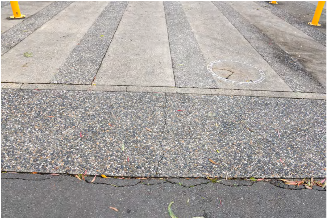
Western side of the Boulevard. Area adjacent to area between 'The Royal Hall of Industries' & 'The Hordern Pavilion'. Heading north. Area of the pedestrian crossing. Cracked concrete and asphalt road paving.
