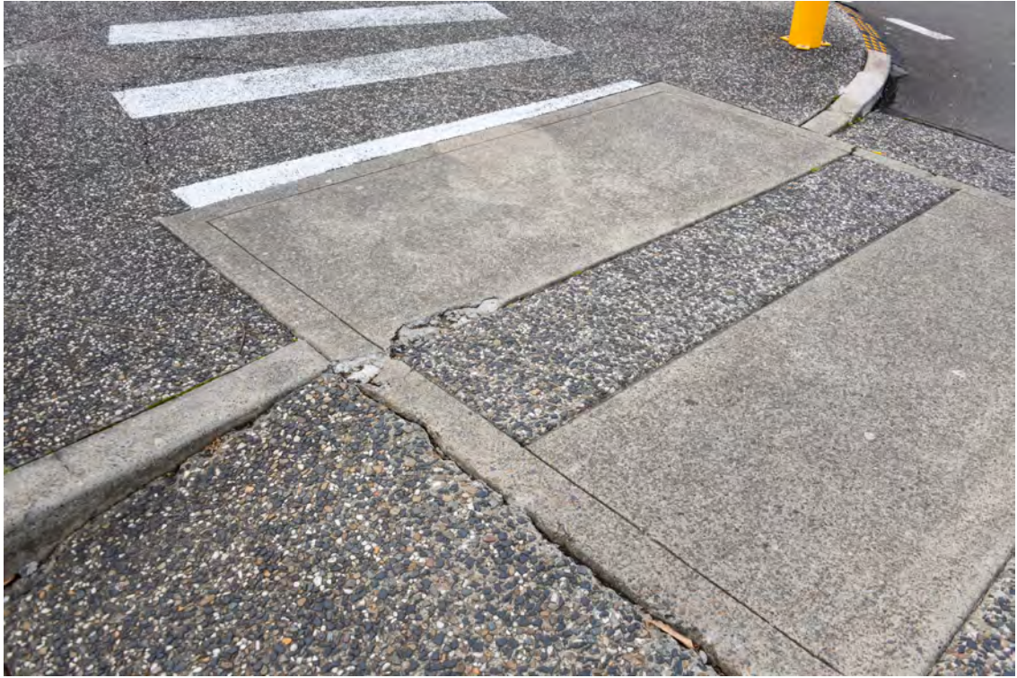
Roundabout at the northern end of the Boulevard. Intersection with Bent Street. Chipped paving.
