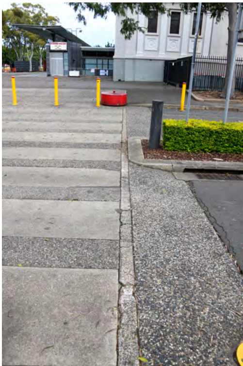
Eastern side of the Boulevard. Area opposite 'The Hordern Pavilion'. Area of the pedestrian crossing. Heading south. Cracked paving.
