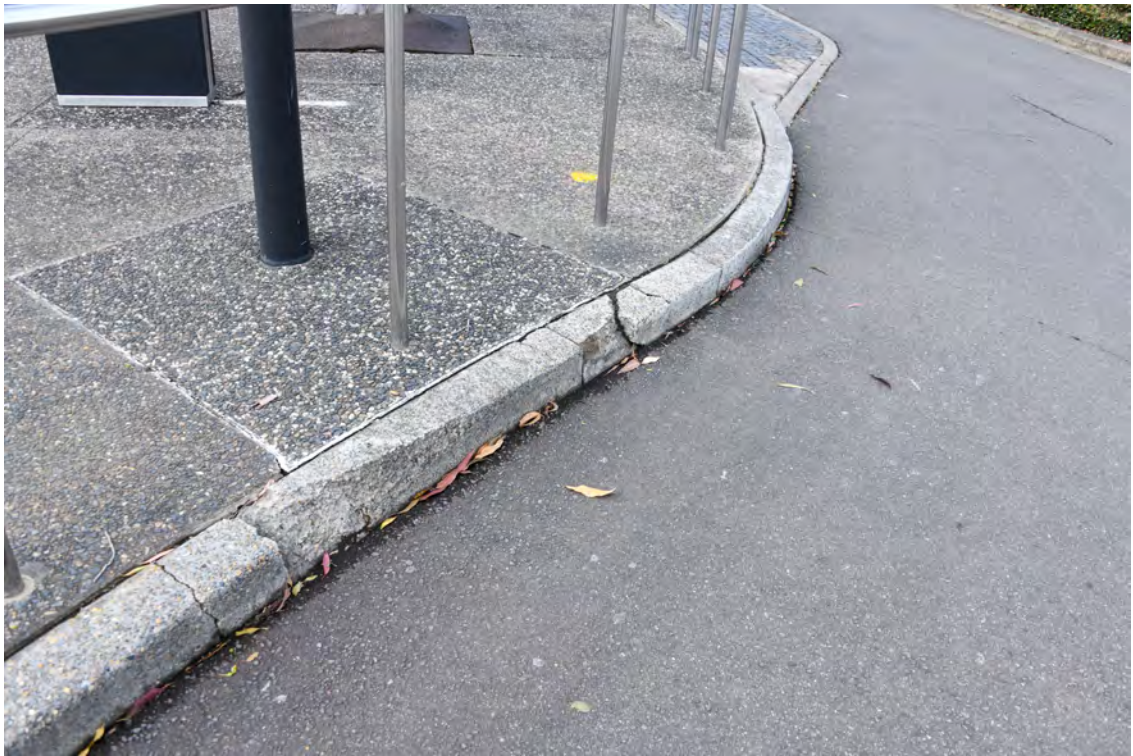
Roundabout at the northern end of the Boulevard. Eastern side of the roundabout. Heading clockwise. Cracked and chipped kerb.
