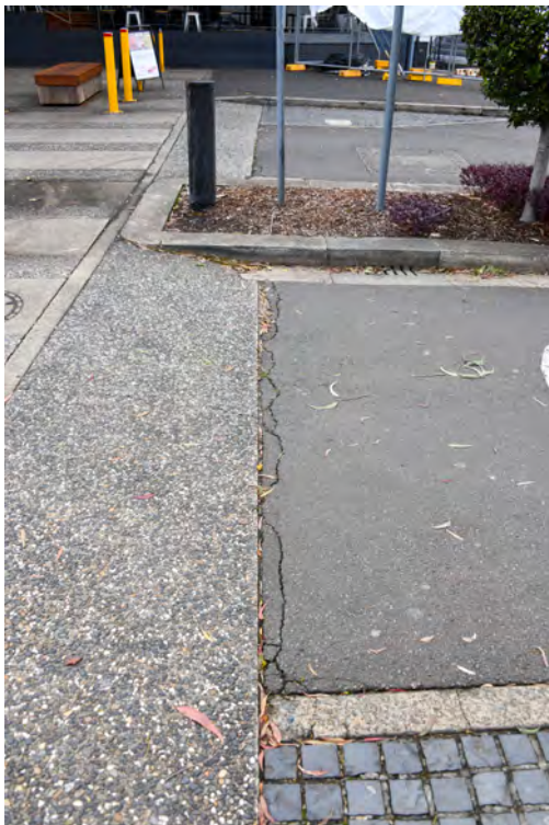
Western side of the Boulevard. Area adjacent to area between 'The Royal Hall of Industries' & 'The Hordern Pavilion'. Heading north. Area of the pedestrian crossing. Junction of the concrete and asphalt road paving.
