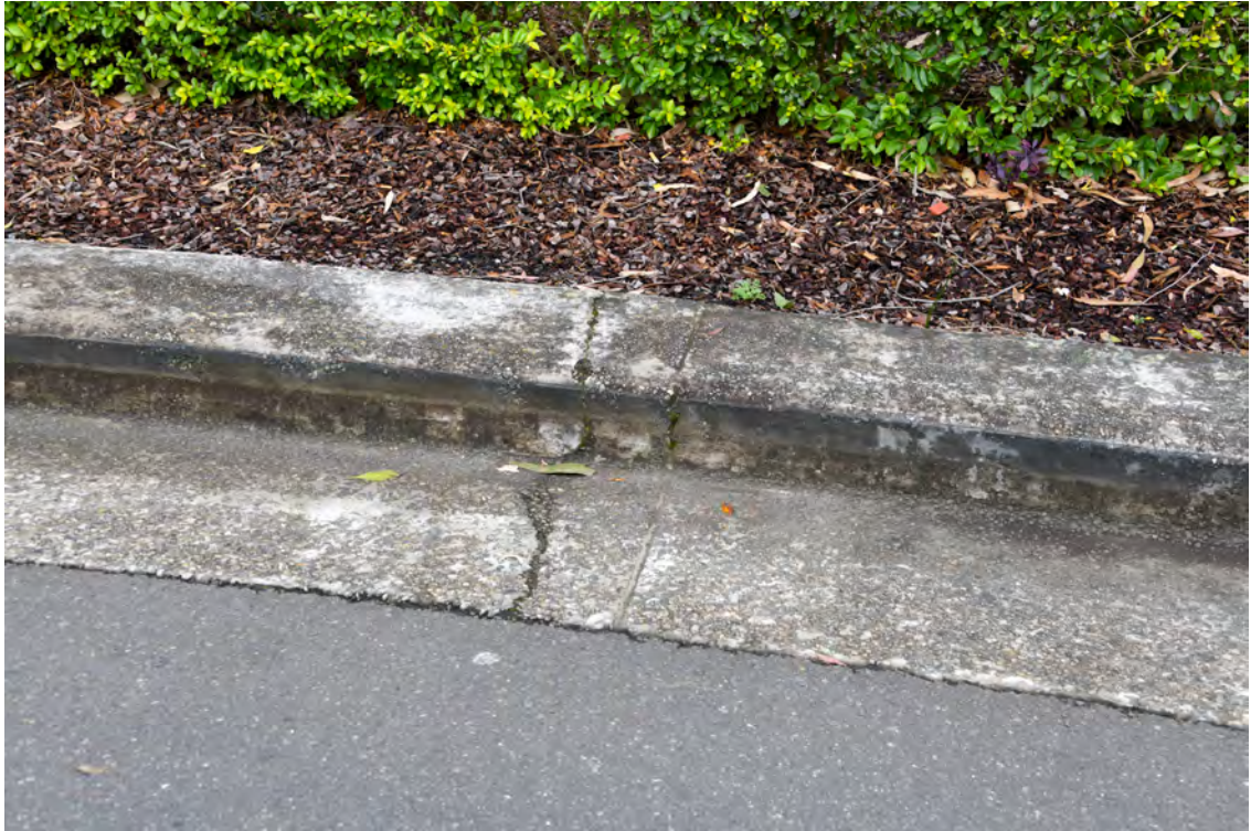
Eastern side of the Boulevard. Area opposite the area between 'The Hordern Pavilion' and 'The Royal Hall of Industries'. Intersection with Park Road. Cracked median strip kerb and gutter.
