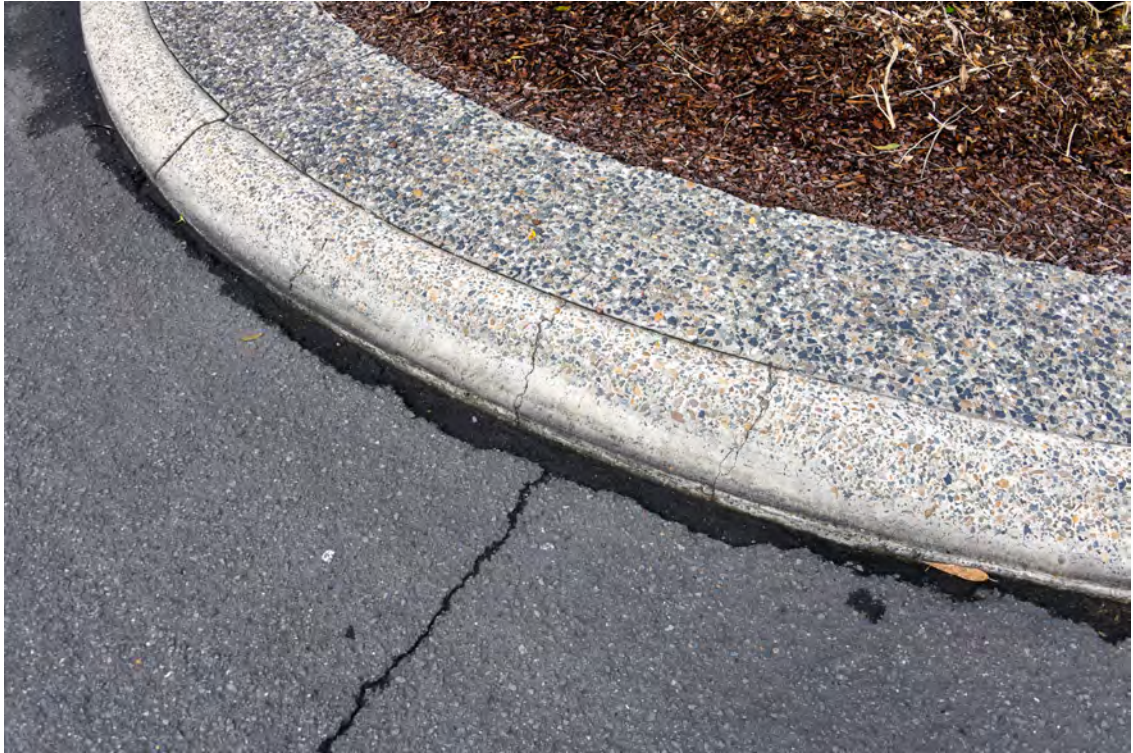
Roundabout at the northern end of the Boulevard. Heading clockwise around the centre of the roundabout. Eastern side. Cracked kerb.
