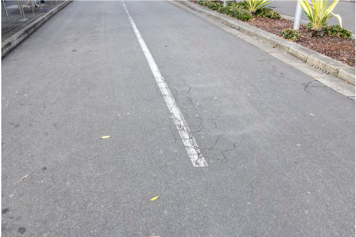
Eastern side of the Boulevard. Area opposite 'The Hordern Pavilion'. Area approaching the intersection with Park Road. Heading south. Cracked paving.
