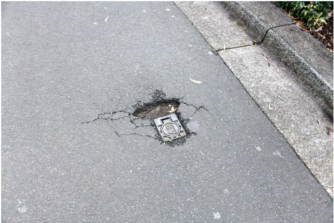
Western side of the Boulevard. Area adjacent to 'The Hordern Pavilion'. Heading north. Damaged paving around the service valve in the road paving.
