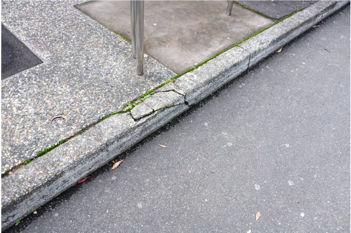
Eastern side of the Boulevard. Area opposite 'The Hordern Pavilion'. Area approaching the intersection with Park Road. Heading south. Cracked kerb.
