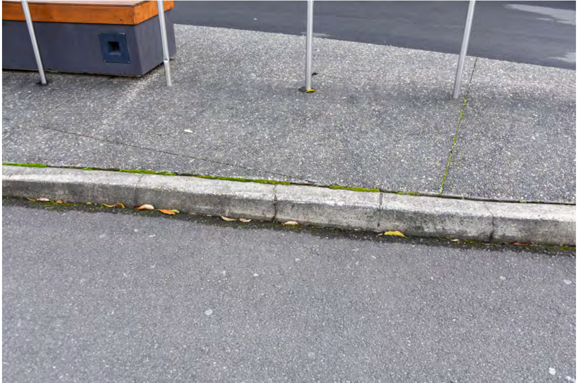
Roundabout at the northern end of the Boulevard. Heading clockwise. Northern side of the roundabout. Cracked kerb.
