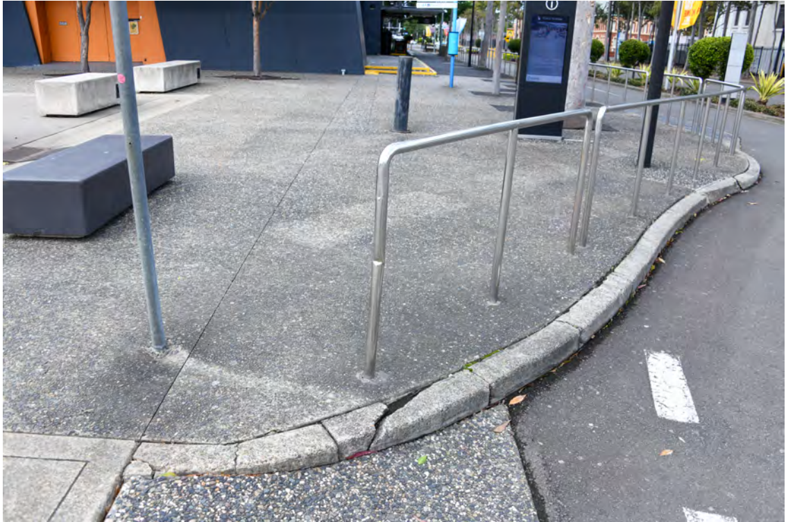
Roundabout at the northern end of the Boulevard. Eastern side of the roundabout. Heading clockwise. Cracked kerb and indentations in the balustrade.
