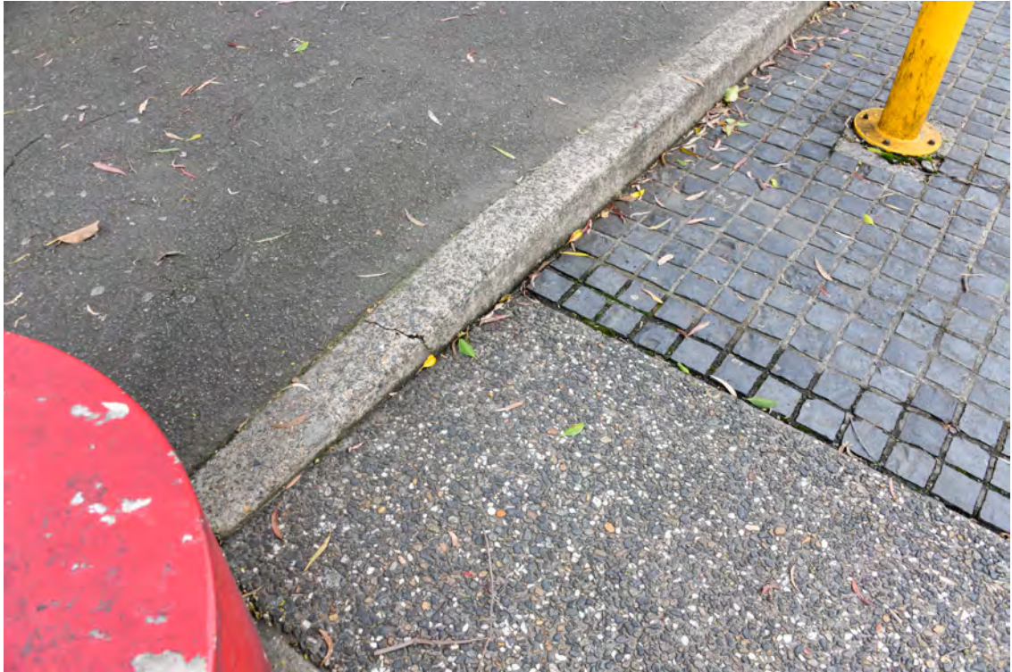
Western side of the Boulevard. Area adjacent to area between 'The Royal Hall of Industries' & 'The Hordern Pavilion'. Heading north. Area of the pedestrian crossing. Cracked kerb.
