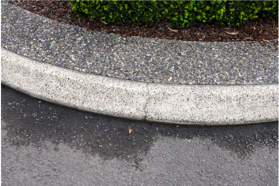
Roundabout at the northern end of the Boulevard. Heading clockwise around the centre of the roundabout. South-western side. Cracked kerb.
