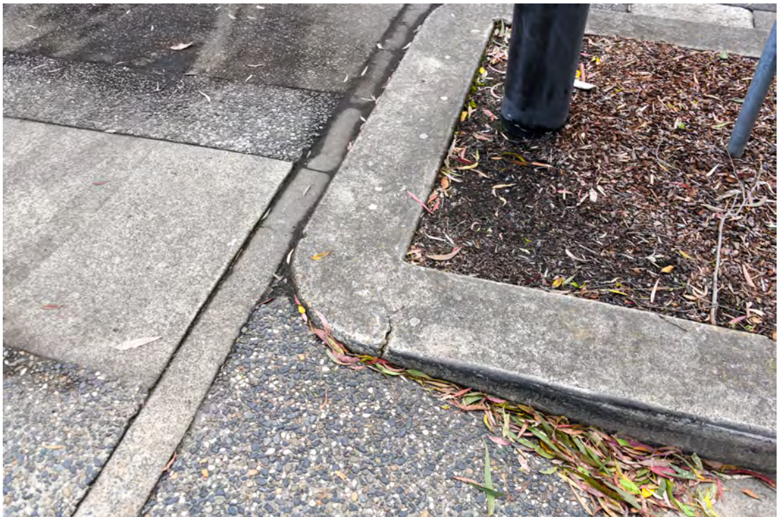
Western side of the Boulevard. Area adjacent to area between 'The Royal Hall of Industries' & 'The Hordern Pavilion'. Heading north. Area of the pedestrian crossing. Cracked median strip kerb.
