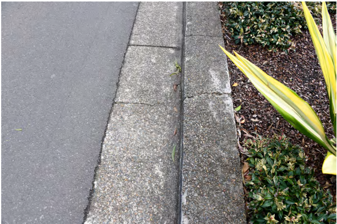
Western side of the Boulevard. Area adjacent to 'The Royal Hall of Industries'. Heading north. Median strip. Cracked kerb and gutter.
