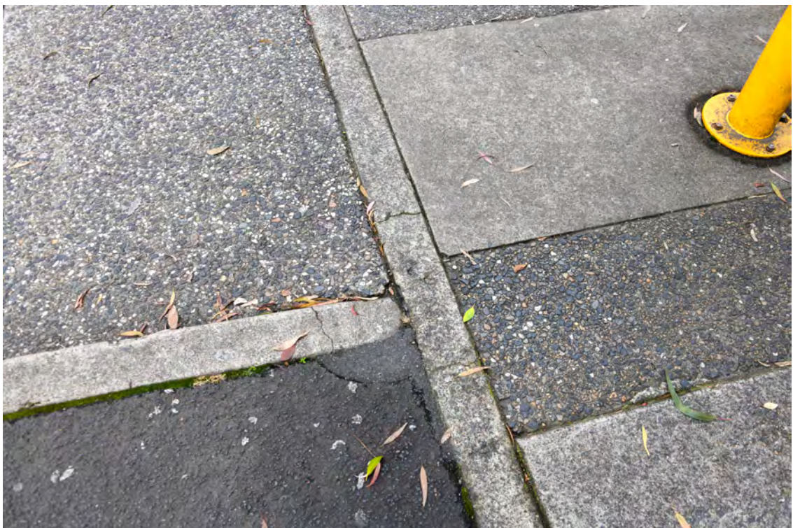
Eastern side of the Boulevard. Area opposite the area between 'The Hordern Pavilion' and 'The Royal Hall of Industries'. Area of the pedestrian crossing. Heading south. Cracked paving.
