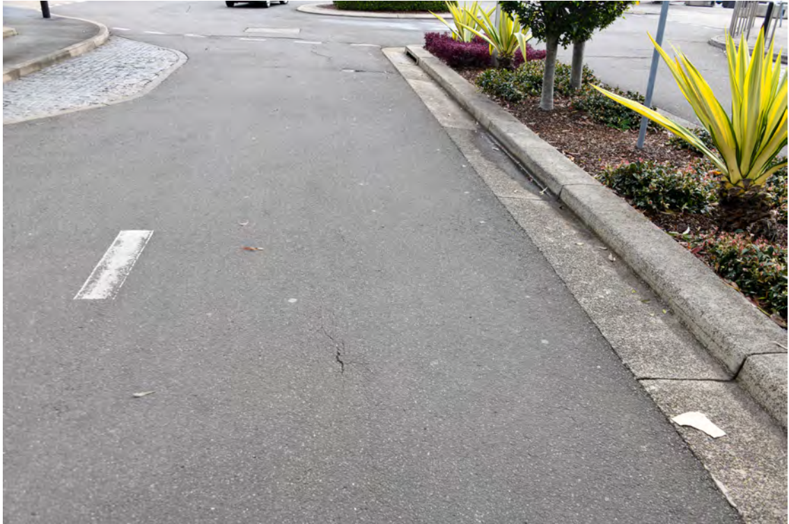
Western side of the Boulevard. Area adjacent to 'The Hordern Pavilion'. Heading north. Cracked paving.
