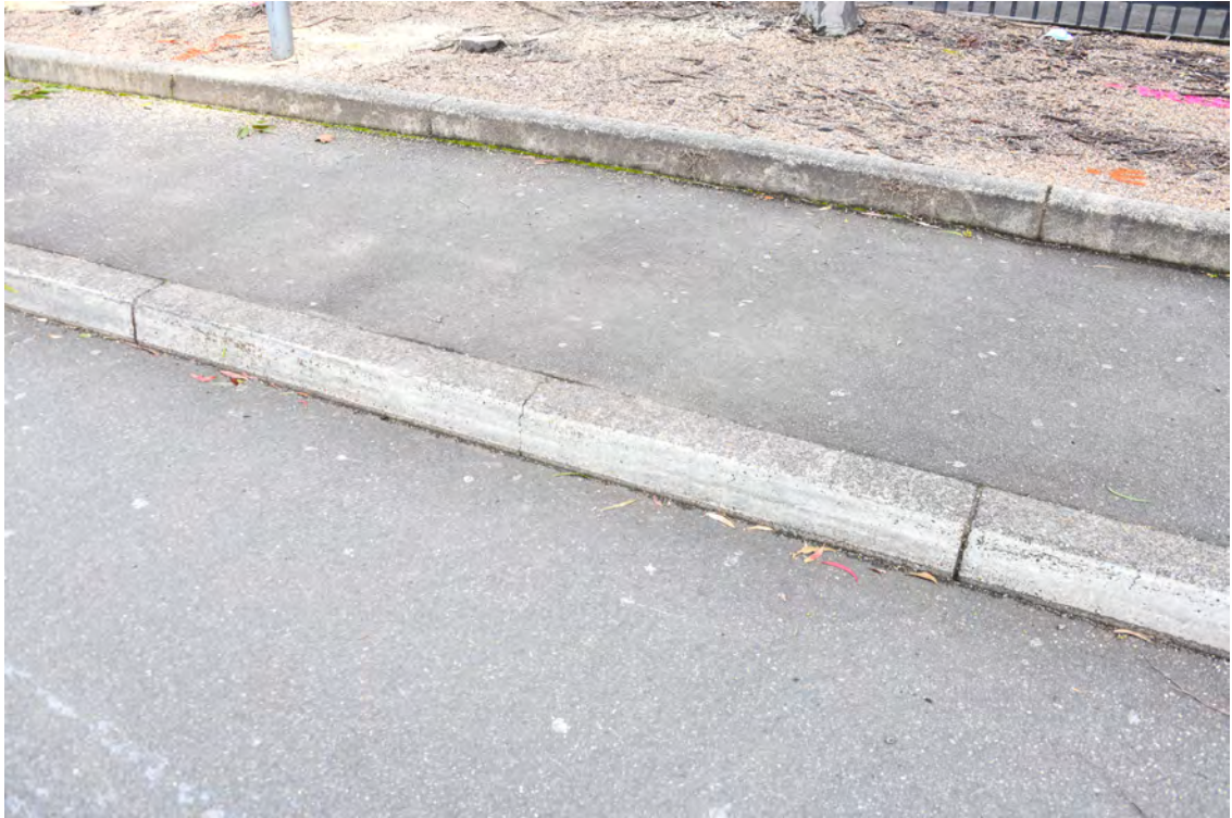
Western side of the Boulevard. Area adjacent to area between 'The Royal Hall of Industries' & 'The Hordern Pavilion'. Heading north. Cracked kerb and gutter.
