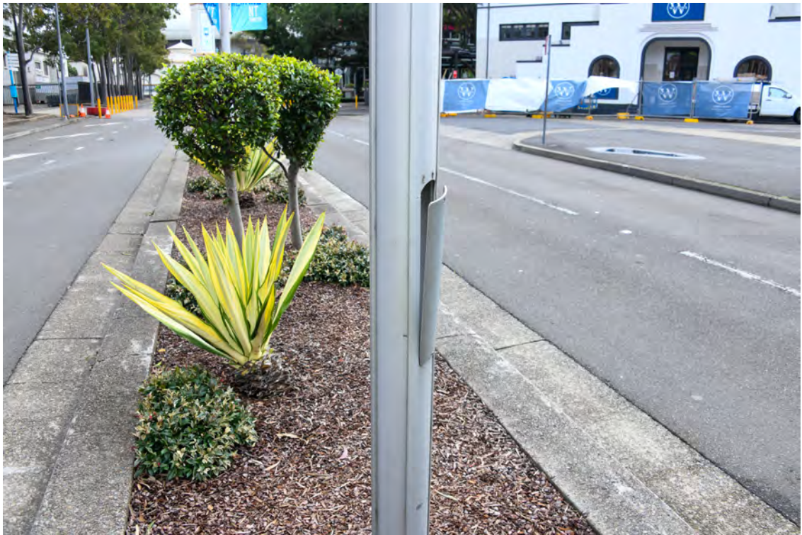
Western side of the Boulevard. Area adjacent to 'The Royal Hall of Industries'. Heading north. Flag pole on the median strip. Loose panel on the pole.
