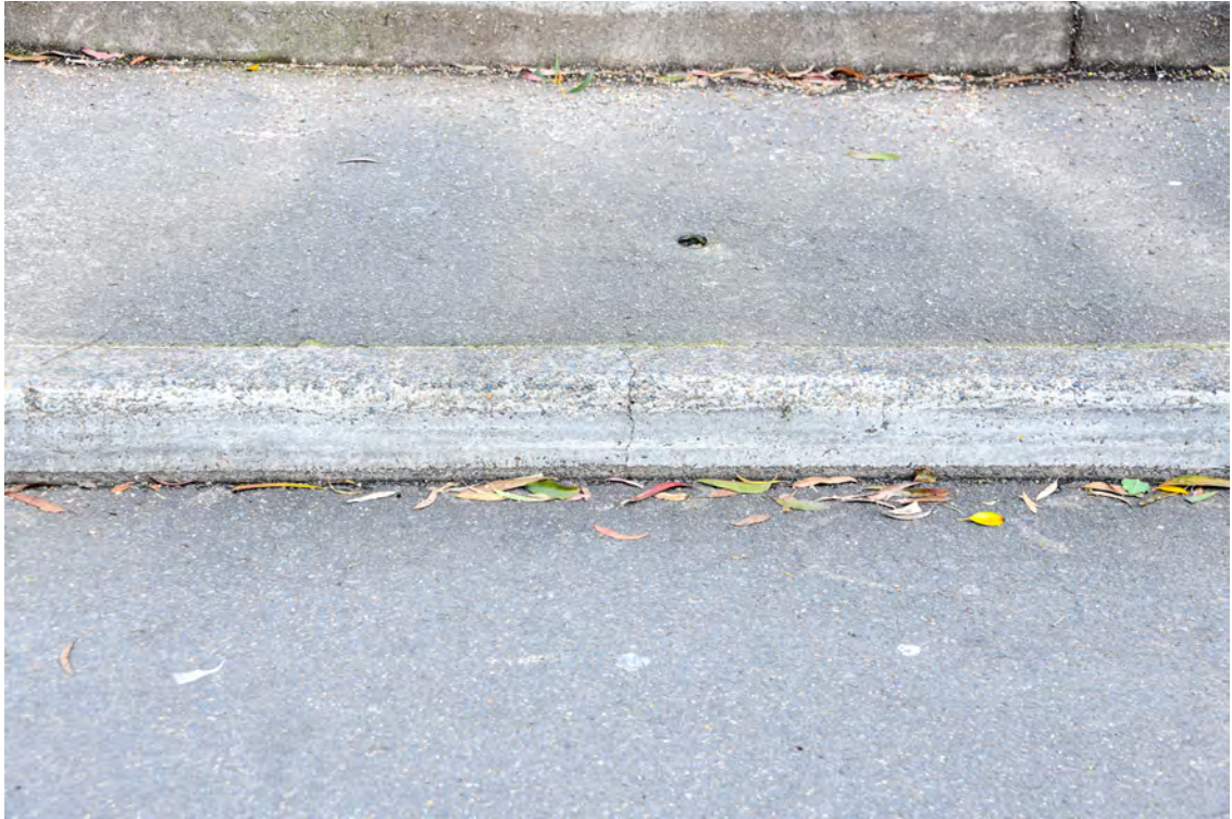
Western side of the Boulevard. Area adjacent to area between 'The Royal Hall of Industries' & 'The Hordern Pavilion'. Heading north. Intersection with Park Road. Cracked kerb and gutter.
