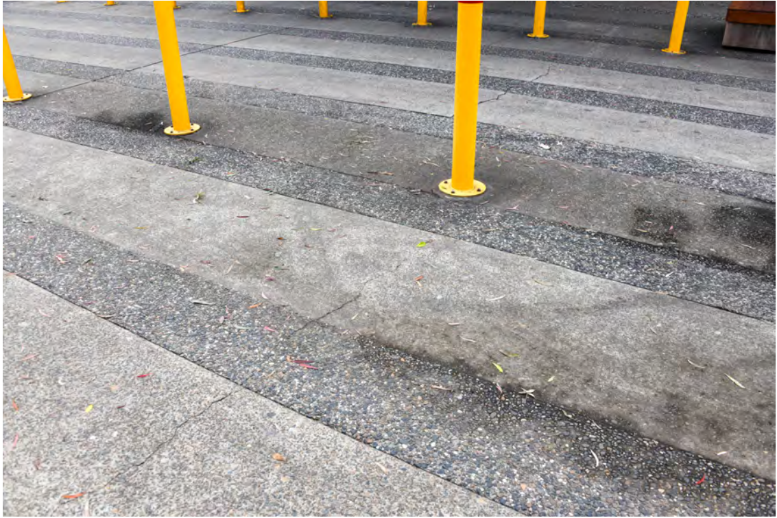
Western side of the Boulevard. Area adjacent to area between 'The Royal Hall of Industries' & 'The Hordern Pavilion'. Heading north. Area of the pedestrian crossing. Cracked paving.
