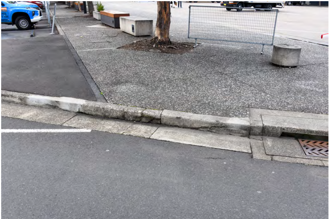
Roundabout at the northern end of the Boulevard. Intersection with Bent Street. Cracked adjacent kerb.
