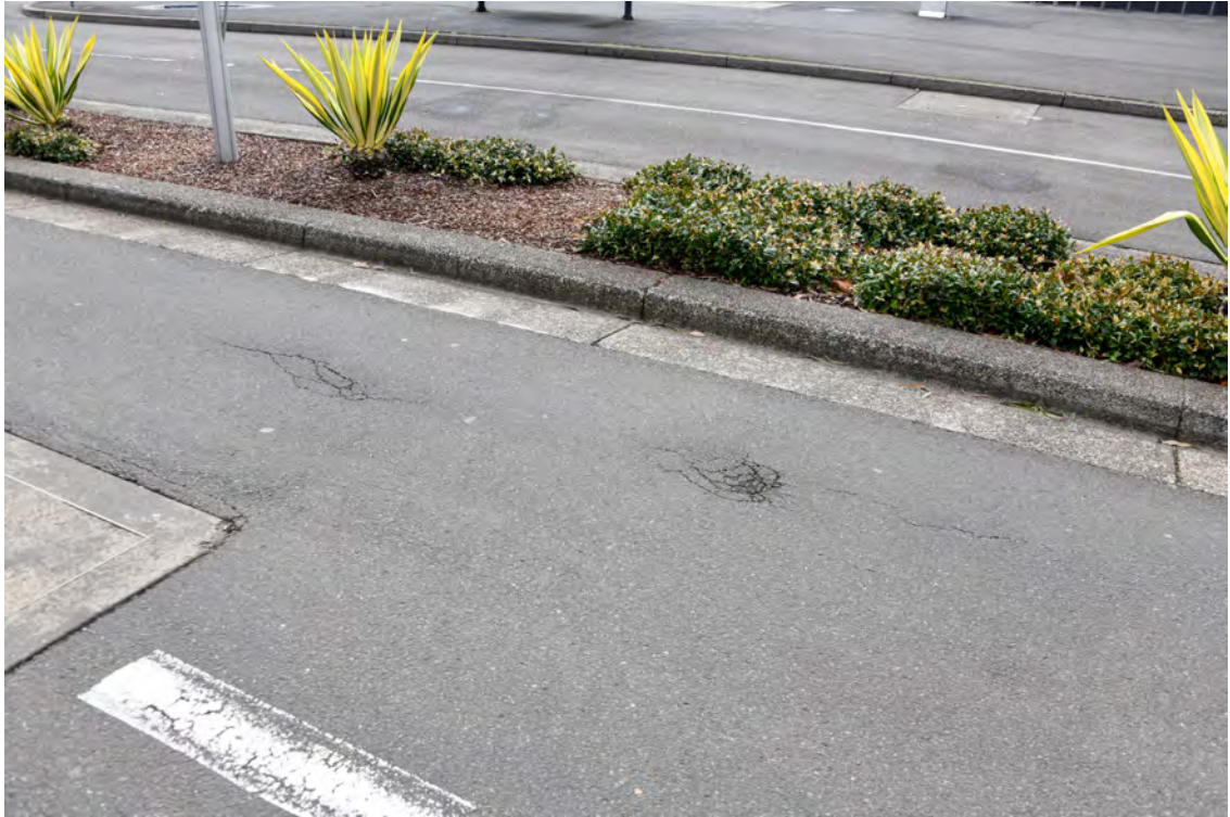
Western side of the Boulevard. Area adjacent to 'The Royal Hall of Industries'. Heading north. Area of the lid to the services pit in the road. Isolated areas of damaged road paving.
