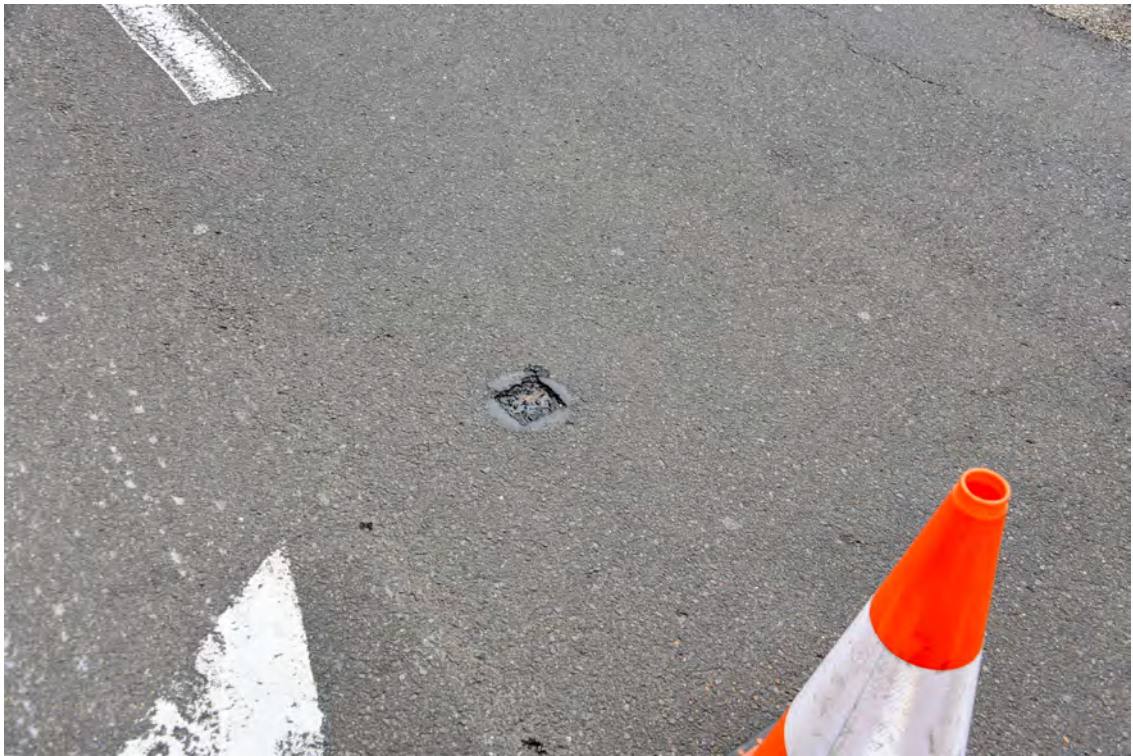
Western side of the Boulevard. Area adjacent to 'The Royal Hall of Industries'. Heading north. Missing reflector.
