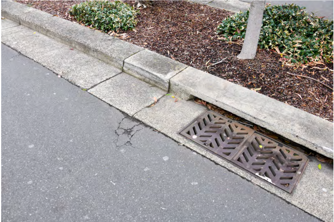
Eastern side of the Boulevard. Area opposite 'The Hordern Pavilion'. Area approaching the intersection with Park Road. Heading south. Storm water drain in the median strip. Cracked adjacent paving.
