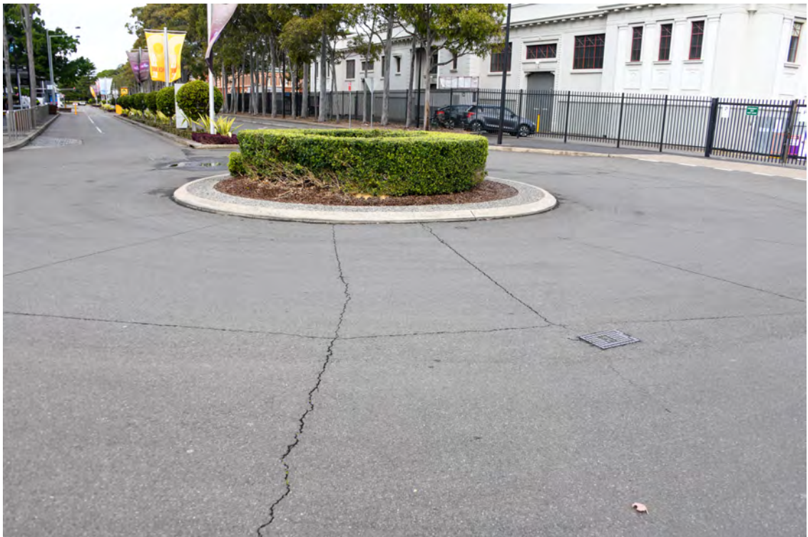
Roundabout at the northern end of the Boulevard. Heading clockwise. Northern side of the roundabout. Intersection with Bent Street. Cracked road paving.
