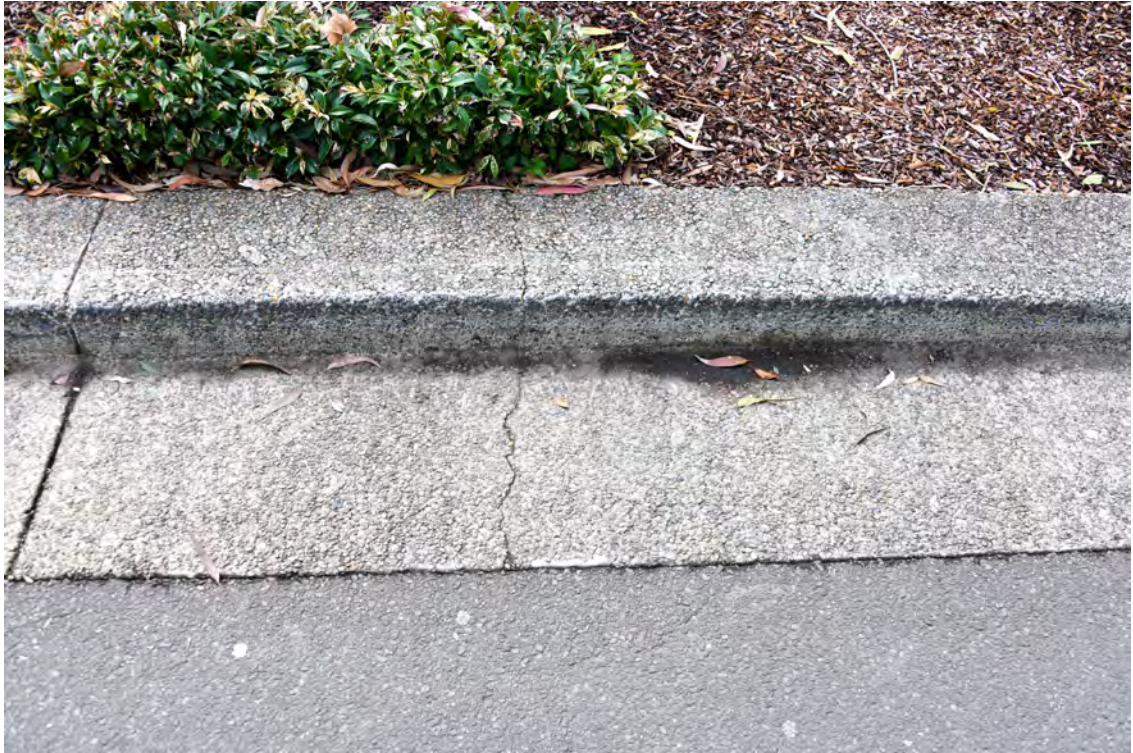
Western side of the Boulevard. Area adjacent to 'The Hordern Pavilion'. Heading north. Median strip. Cracked kerb and gutter.
