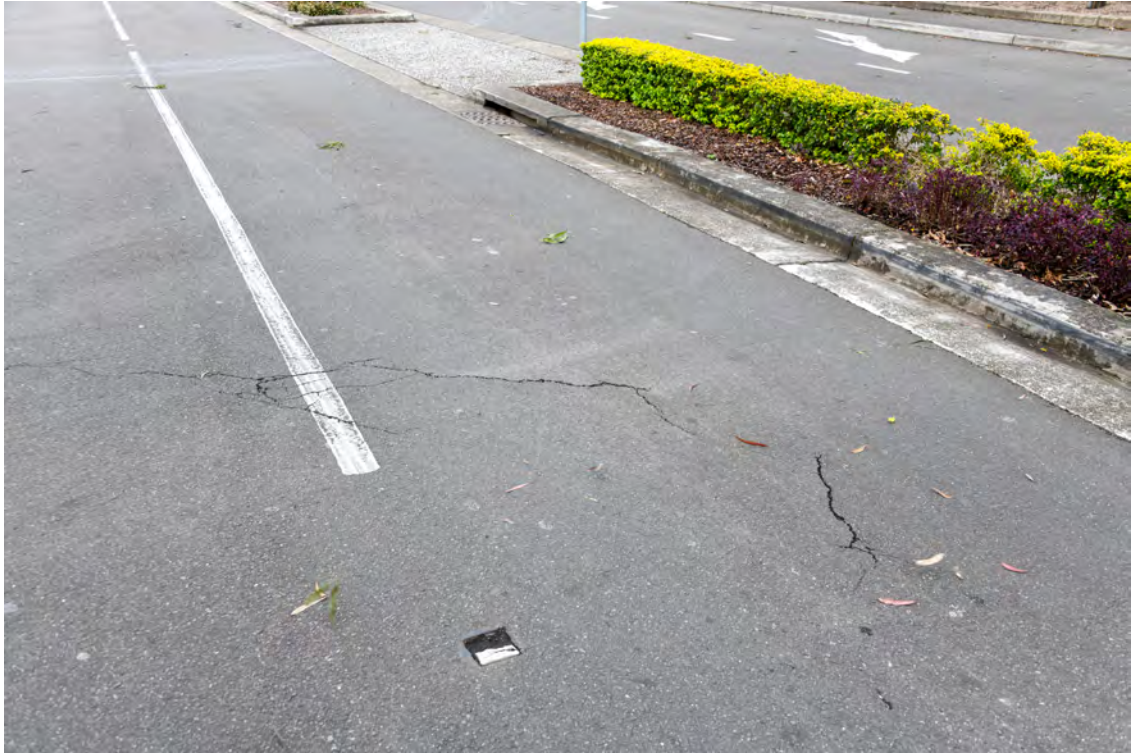
Eastern side of the Boulevard. Area opposite the area between 'The Hordern Pavilion' and 'The Royal Hall of Industries'. Intersection with Park Road. Cracked road paving.
