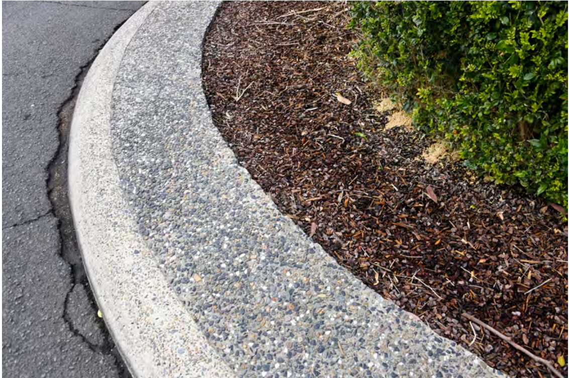
Roundabout at the northern end of the Boulevard. Heading clockwise around the centre of the roundabout. Northern side. Chipped edges of the paving.
