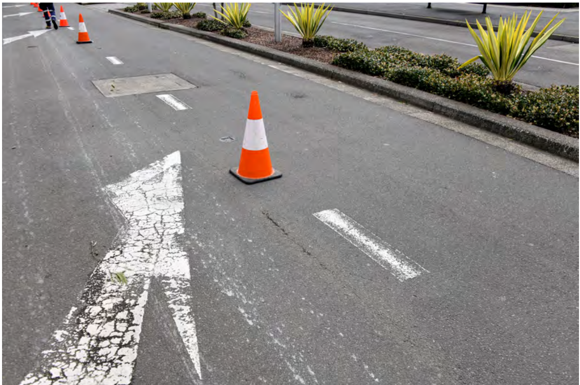
Western side of the Boulevard. Area adjacent to 'The Royal Hall of Industries'. Heading north. Median Strip. Crack in the asphalt road paving.
