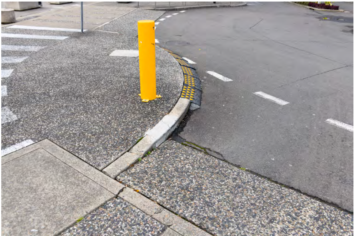
Roundabout at the northern end of the Boulevard. Intersection with Bent Street. Cracked kerb.
