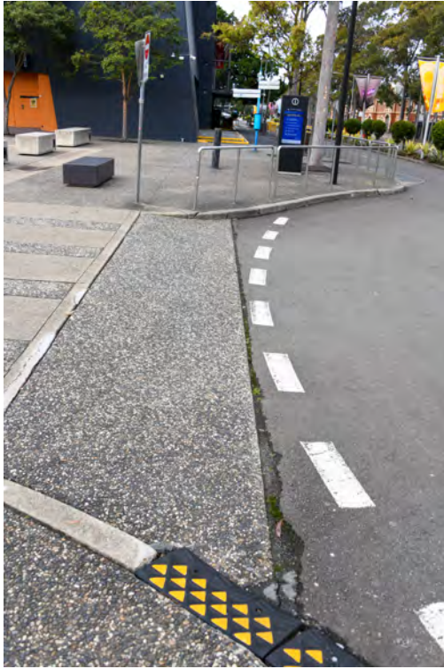
Roundabout at the northern end of the Boulevard. Eastern side of the roundabout. Heading clockwise. Damaged edge of the road paving.
