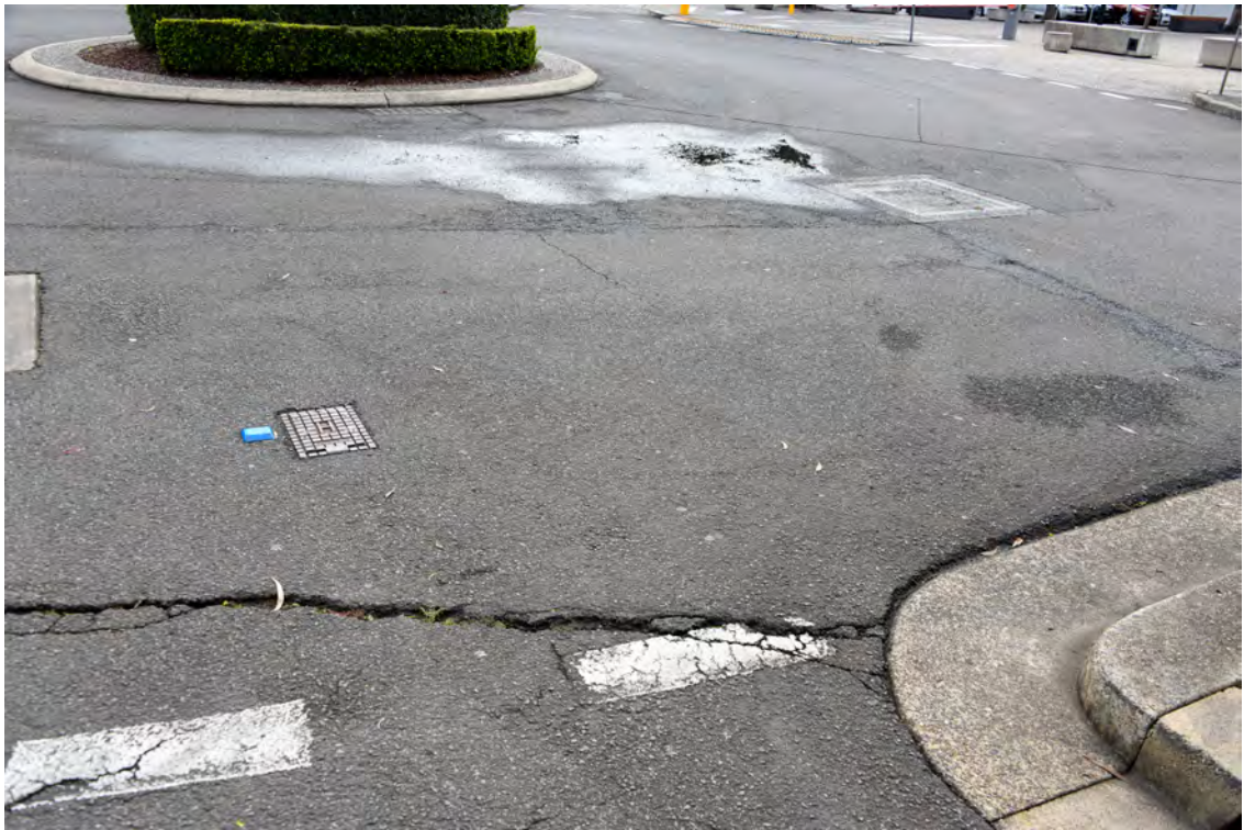
Western side of the Boulevard. Area adjacent to 'The Hordern Pavilion'. Area on the southern side of the roundabout. Cracked road paving.
