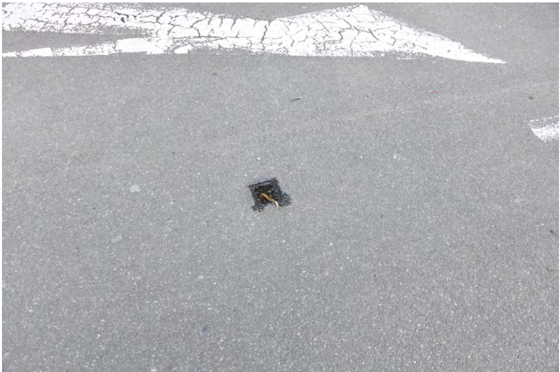
Western side of the Boulevard. Area adjacent to area between 'The Royal Hall of Industries' & 'The Hordern Pavilion'. Heading north. Intersection with Park Road. Missing road reflector.
