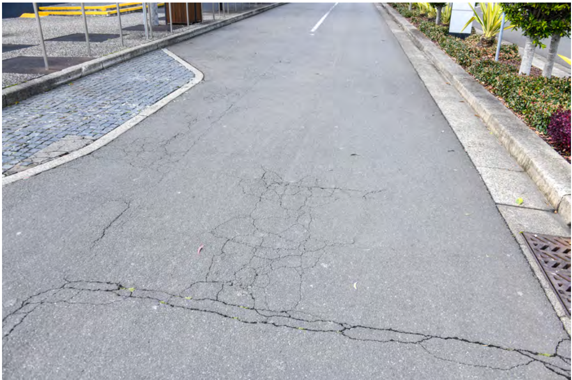
Eastern side of the Boulevard. Heading south from the roundabout at the northern end of the Boulevard. Eastern side of the road. Cracked road paving.
