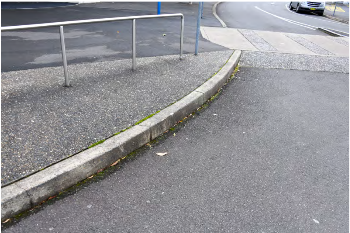
Roundabout at the northern end of the Boulevard. Heading clockwise. Northern side of the roundabout. Intersection with Bent Street. Cracked kerb.
