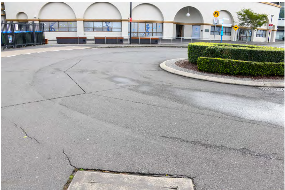
Roundabout at the northern end of the Boulevard. Heading clockwise. South-western side of the roundabout. Cracked road paving.
