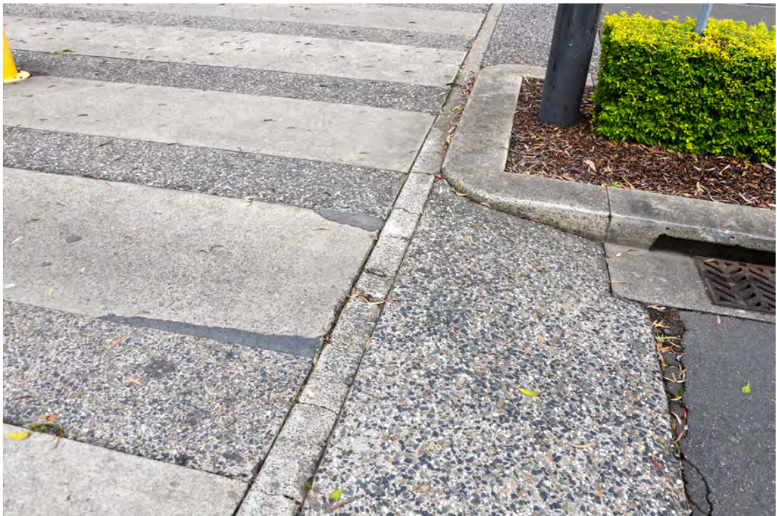
Eastern side of the Boulevard. Area opposite 'The Hordern Pavilion'. Area of the pedestrian crossing. Cracked paving.
