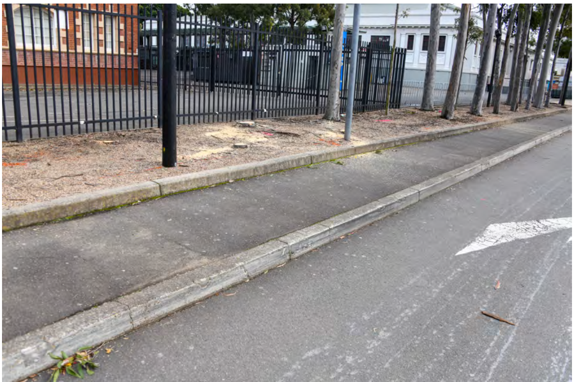
Western side of the Boulevard. Area adjacent to 'The Royal Hall of Industries'. Heading north. Cracked kerb and gutter.
