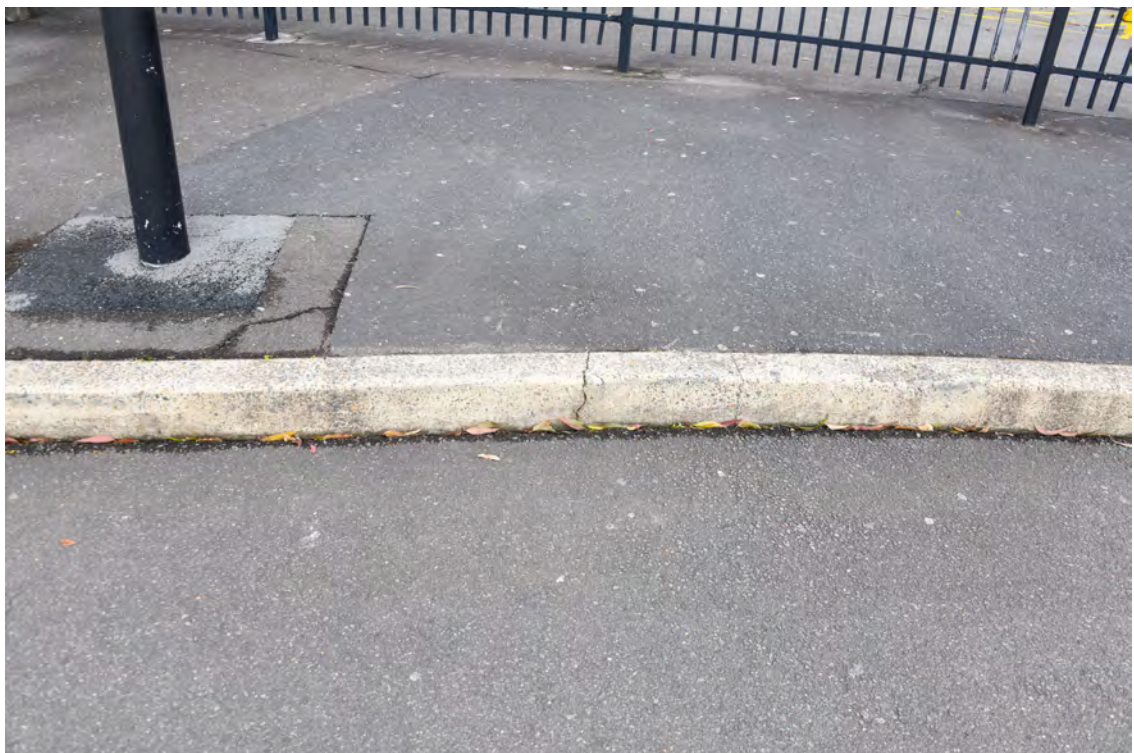
Roundabout at the northern end of the Boulevard. Heading clockwise. Western side of the roundabout. Cracked kerb.
