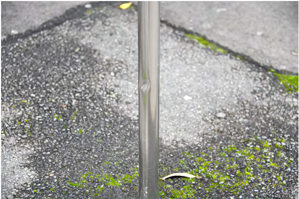
Eastern side of the Boulevard. Area opposite 'The Hordern Pavilion'. Area approaching the intersection with Park Road. Heading south. Indentation in the balustrade.
