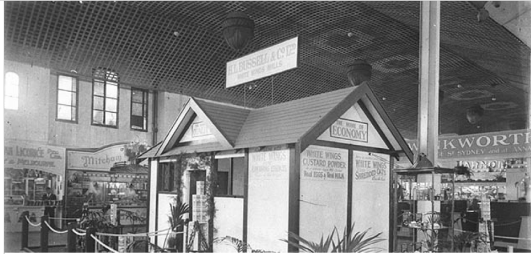
Picture 36 – c1930s. White Wings Flour exhibit showing mesh ceiling below trusses.
