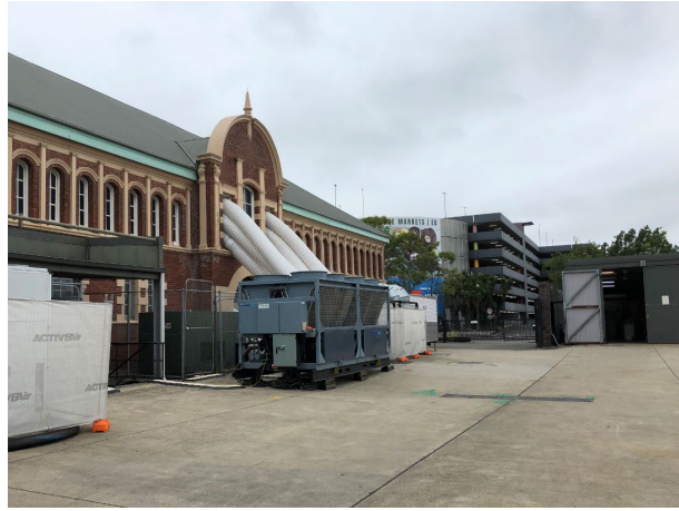
Picture 10 – View across open space to south of building showing temporary air conditioning measures.
