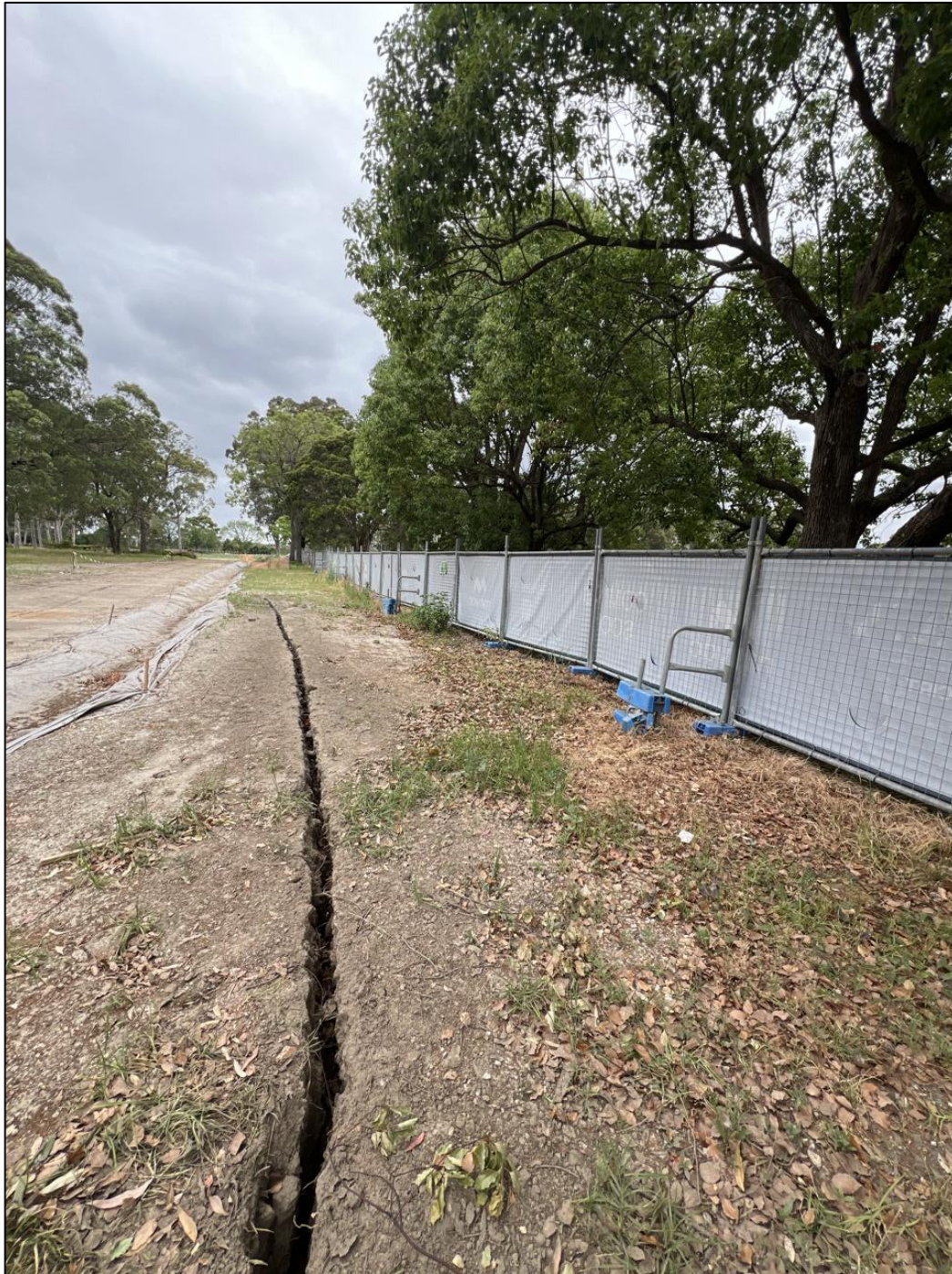
Figure 25. Survey Trench 5 with one Major root encountered. Image taken from northern edge of trench.
