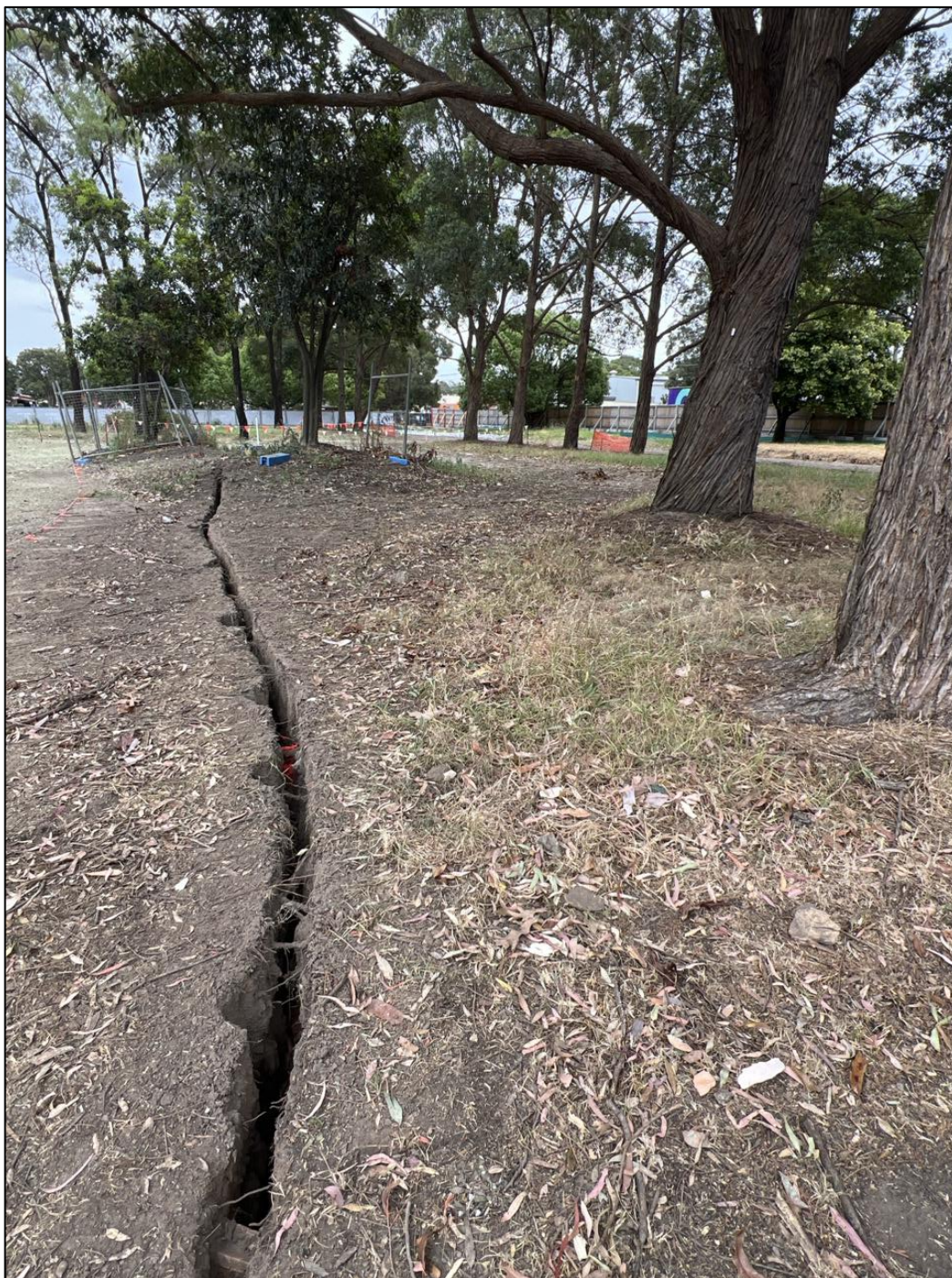
Figure 17. Survey Trench 3 with three Major roots encountered. Image taken from eastern edge of trench.
