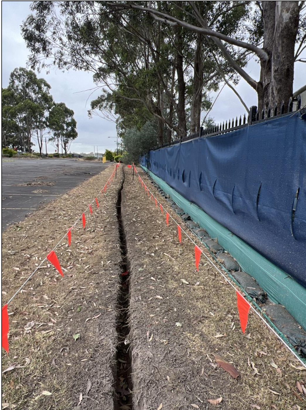
Figure 10. Survey Trench 2 with eleven Major roots encountered. Image taken from western edge of trench.
