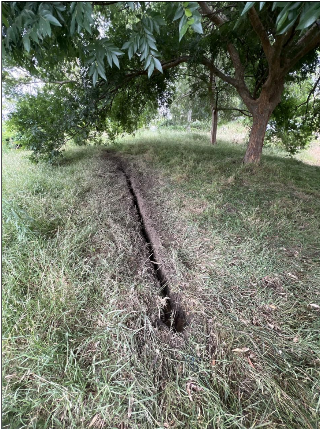
Figure 71. Trench 19 with no major roots encountered. Image taken from southern edge of trench.
