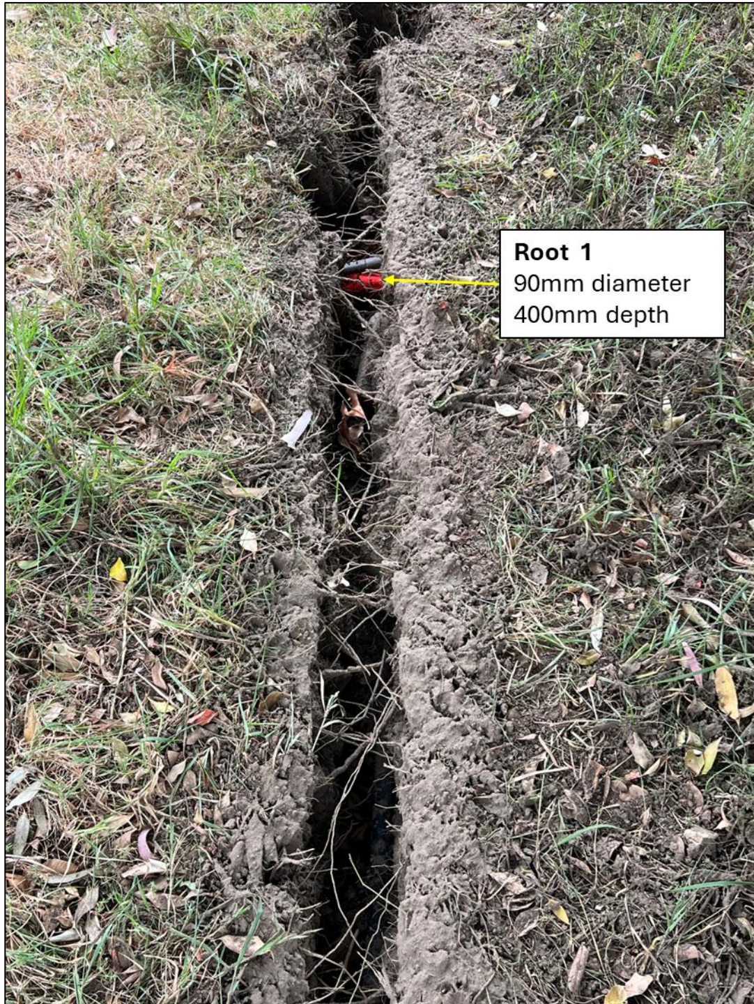
Figure 23. Eastern and central portion of Survey Trench 4.
