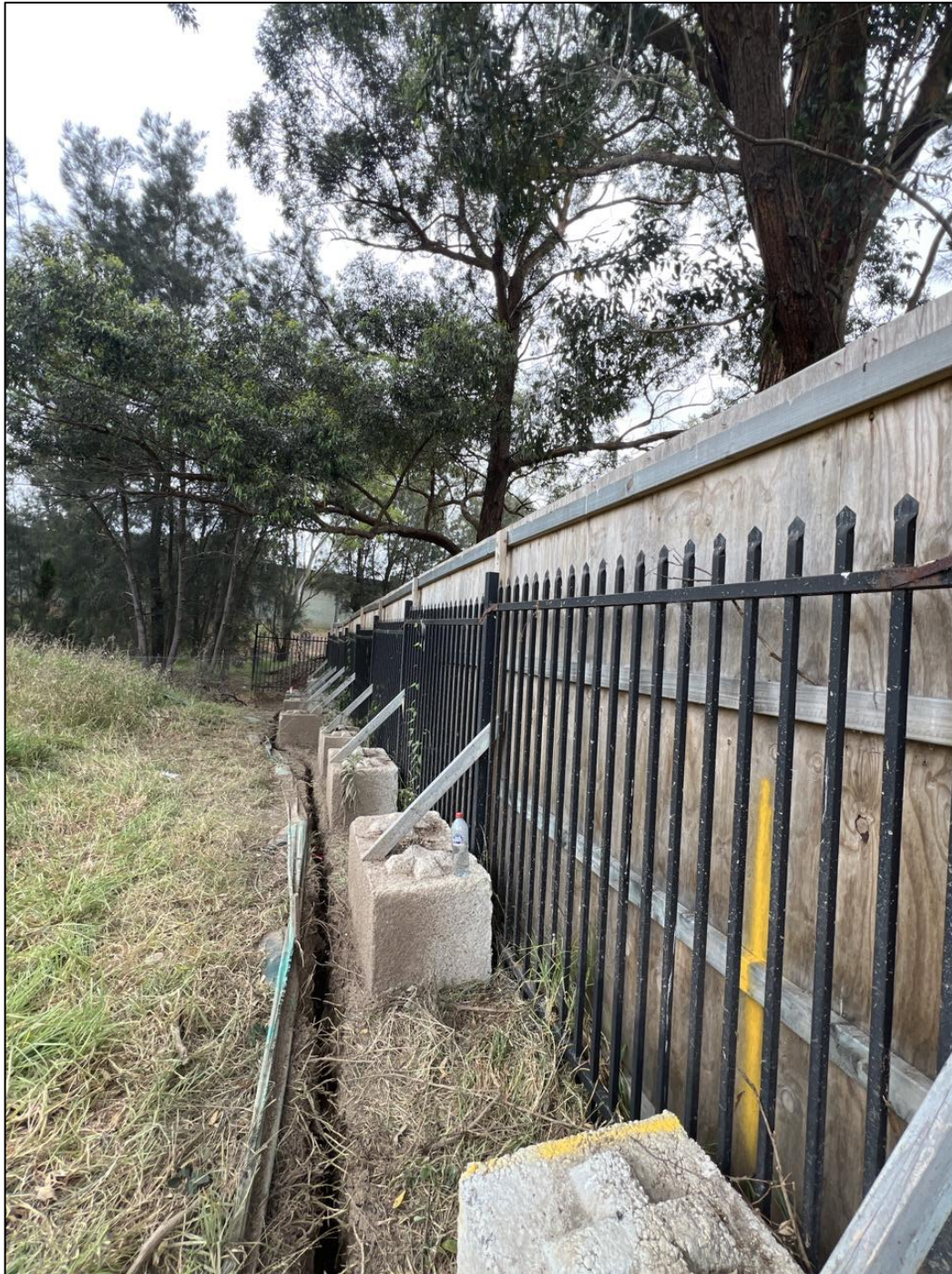
Figure 41. Trench 11 with three major roots encountered. Image taken from eastern edge of trench.
