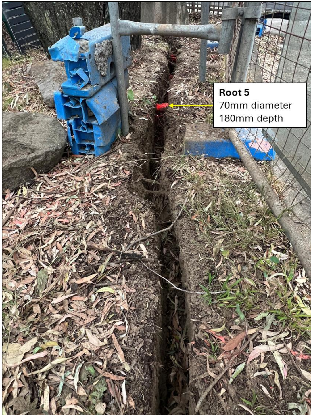
Figure 8. Northern portion of Survey Trench 1.
