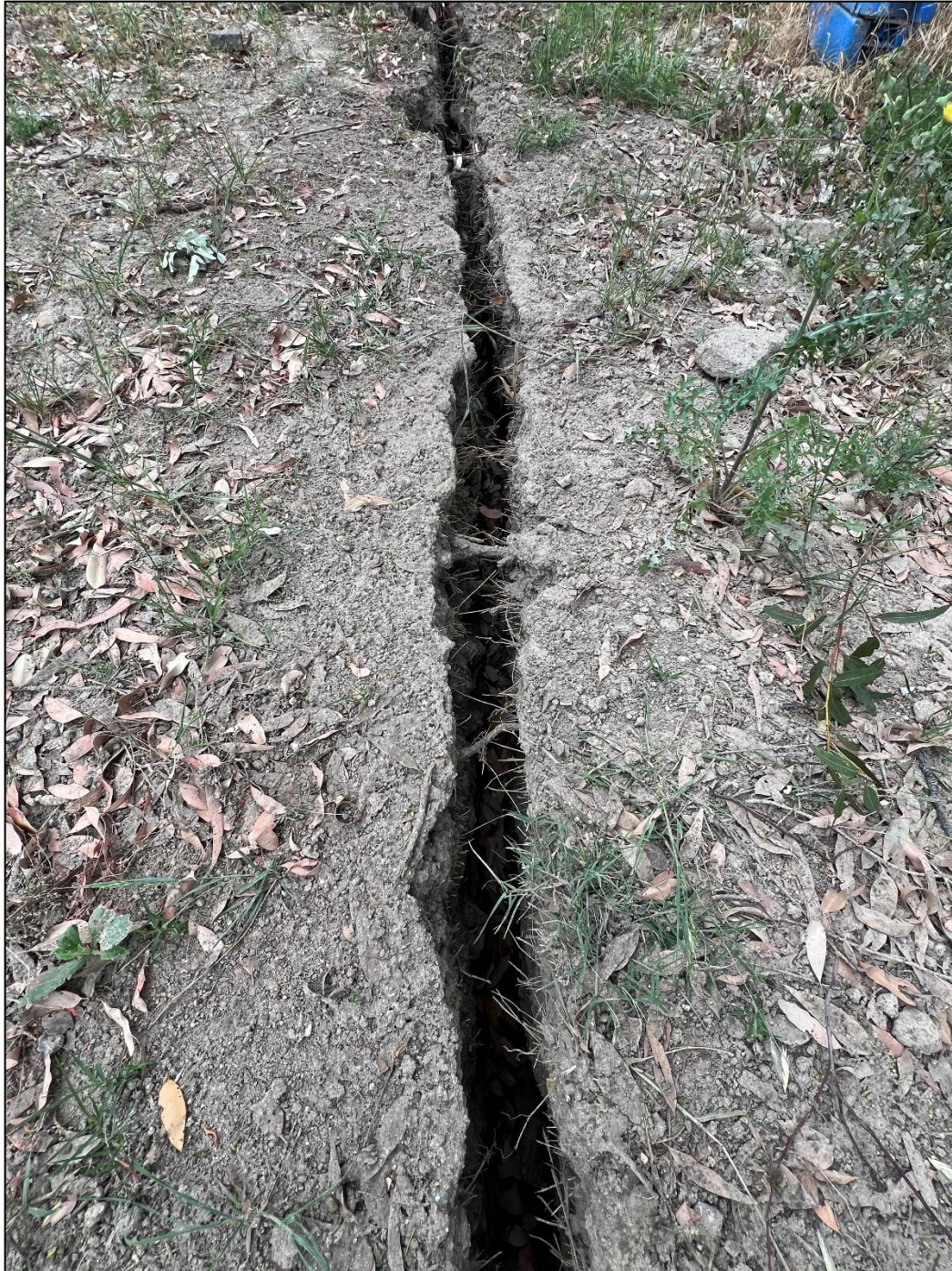
Figure 31. Trench 7 with heavily compact soils and no major roots observed. Minor root growth (14 minor roots) encountered within trench.
