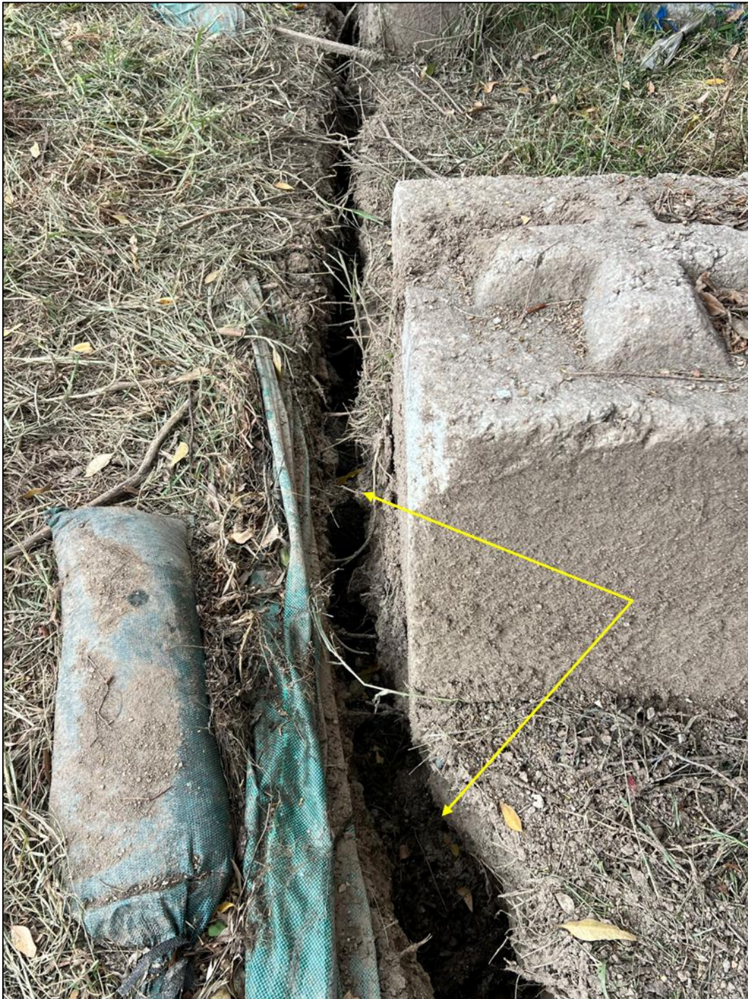
Figure 44. No major roots observed within the southern portion of Survey Trench 11. Heavy clay and a considerable amount of buried rubble were encountered.
