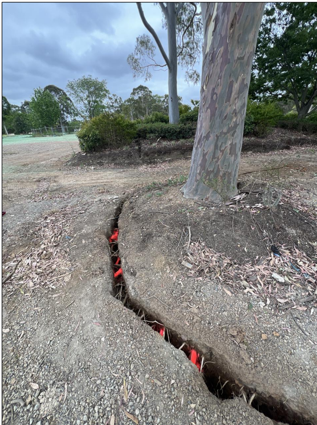
Figure 45. Trench 12 with sixteen major roots encountered. Image taken from south-eastern edge of trench.
