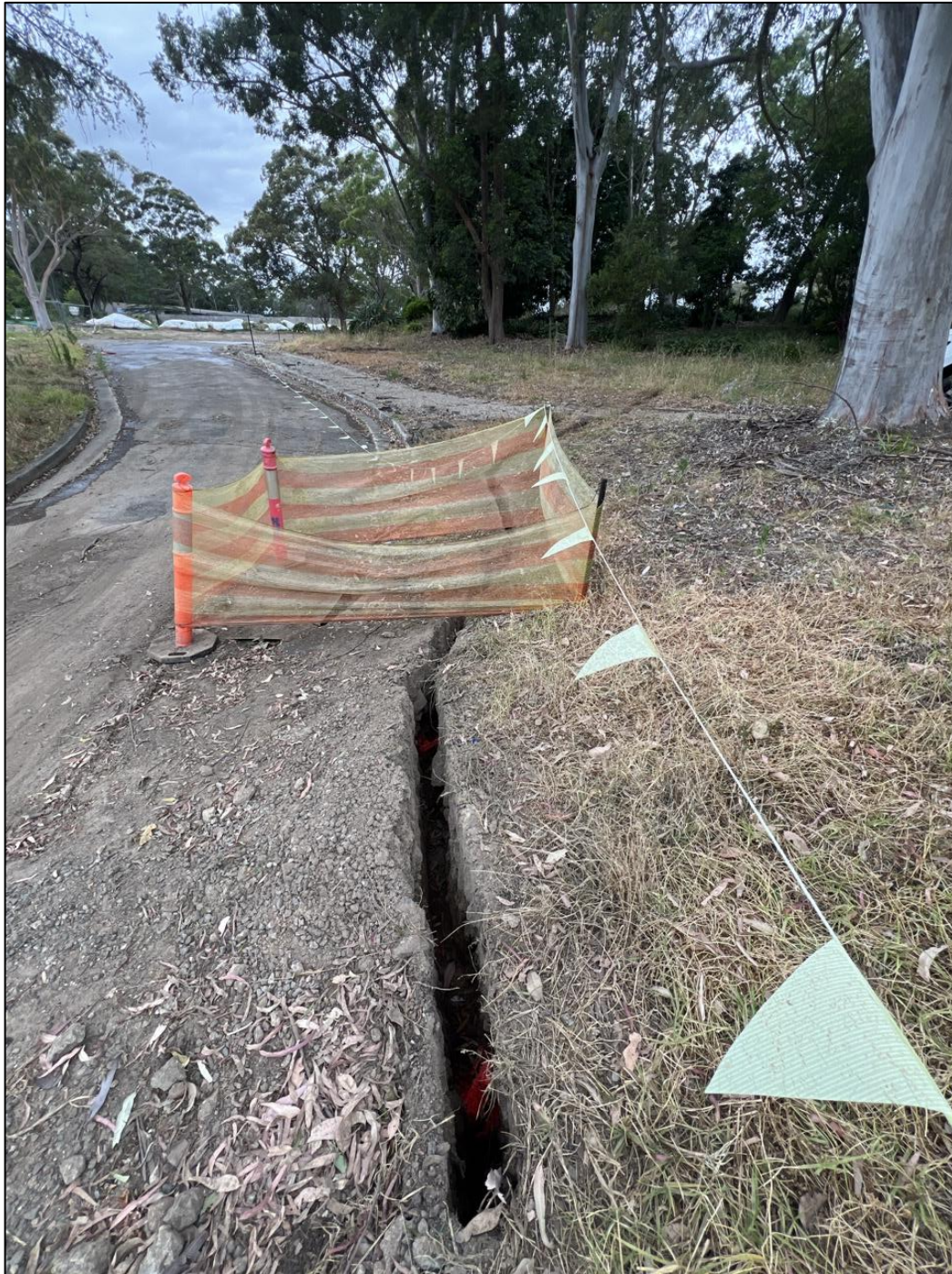
Figure 59. Trench 15 with three major roots encountered. Image taken from western edge of trench.
