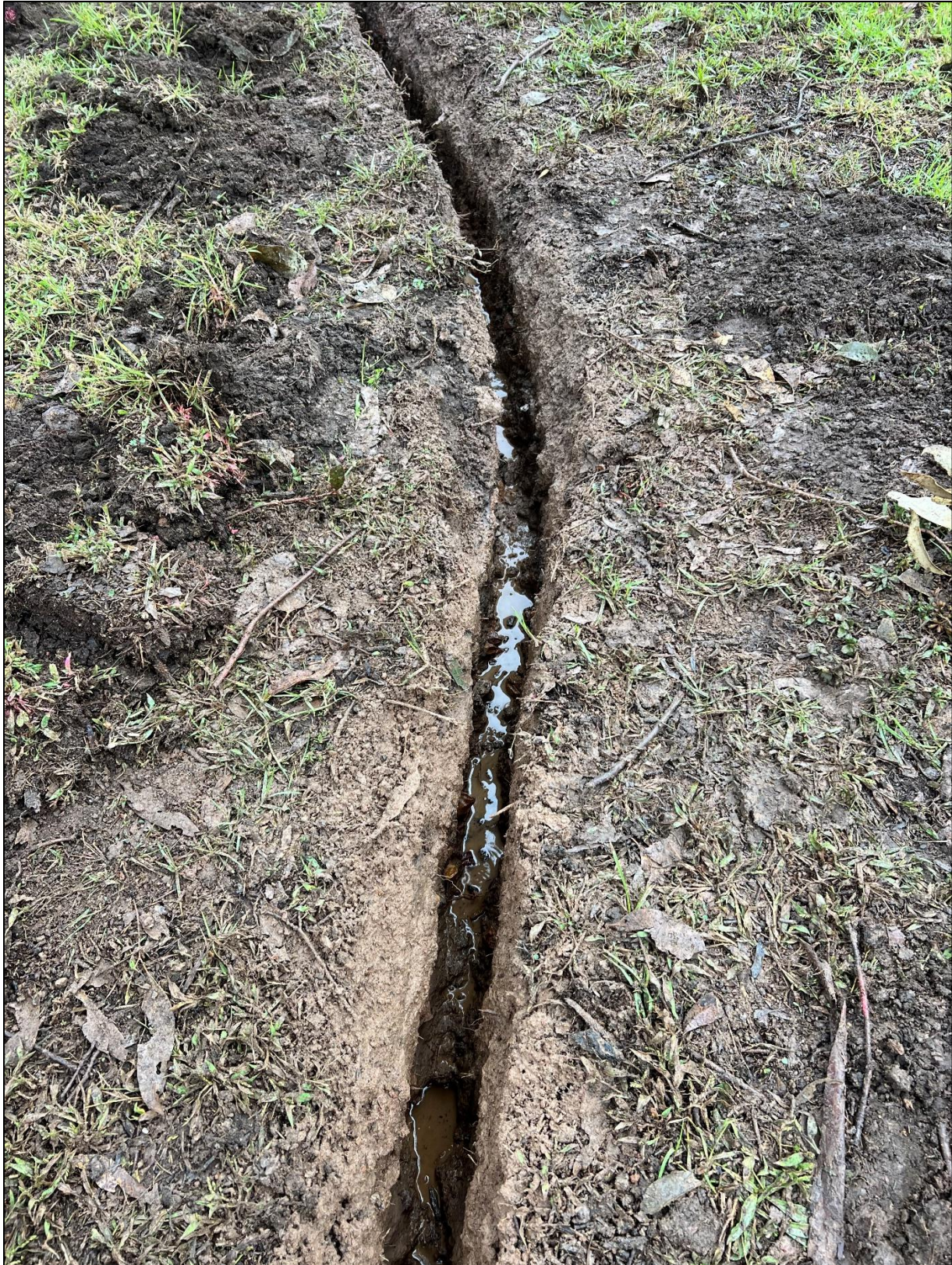
Figure 12. No tree roots observed within the central portion of Survey Trench 1.
