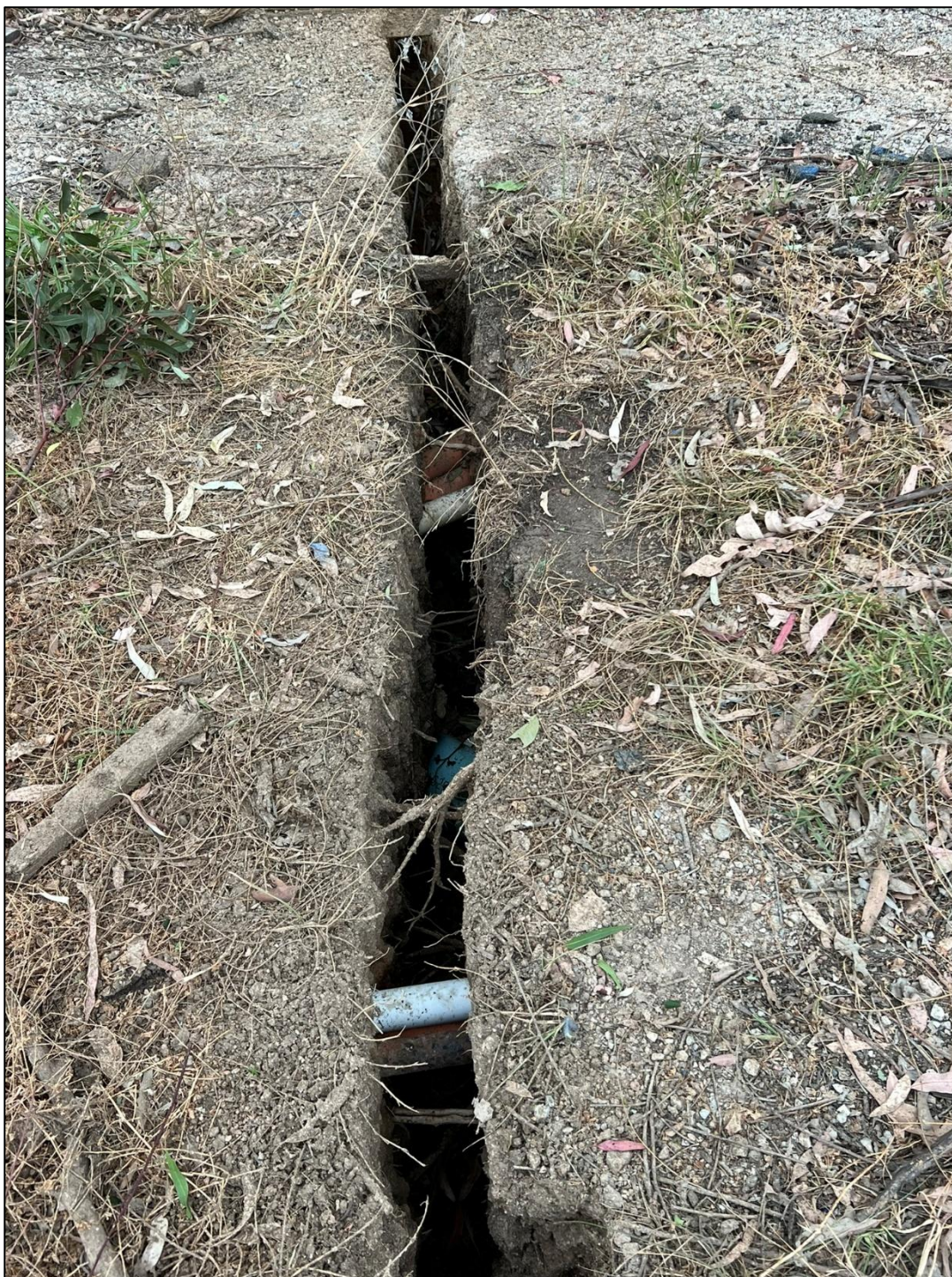
Figure 61. No major roots encountered within the eastern portion of Trench 15.
