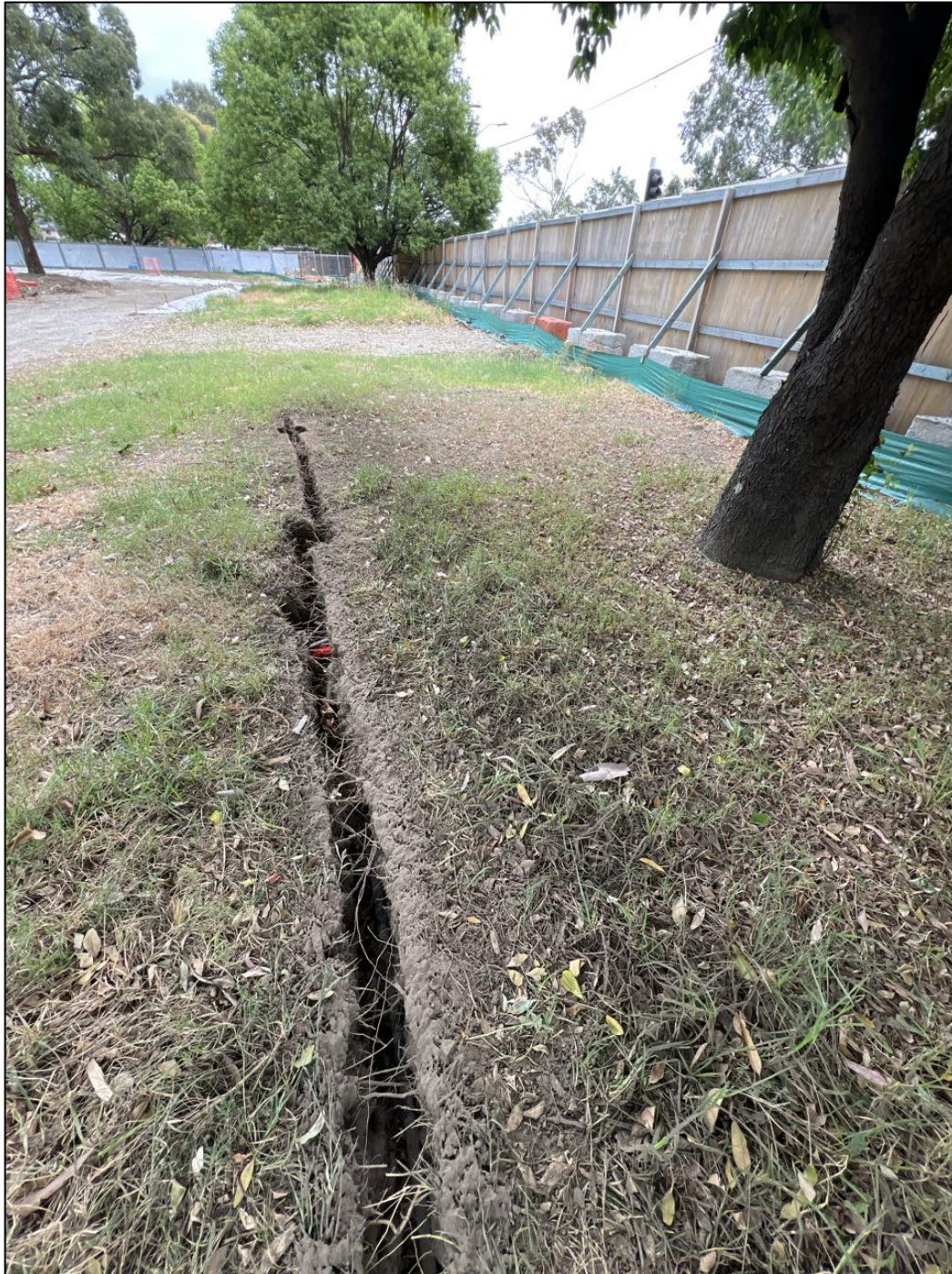
Figure 22. Survey Trench 4 with one Major root encountered. Image taken from eastern edge of trench.
