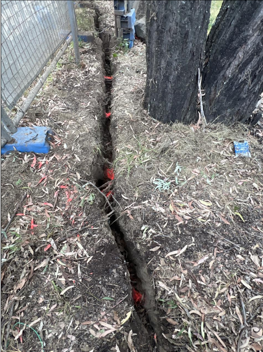
Figure 6. Survey Trench 1 with five Major roots encountered. Image taken from eastern edge of trench.
