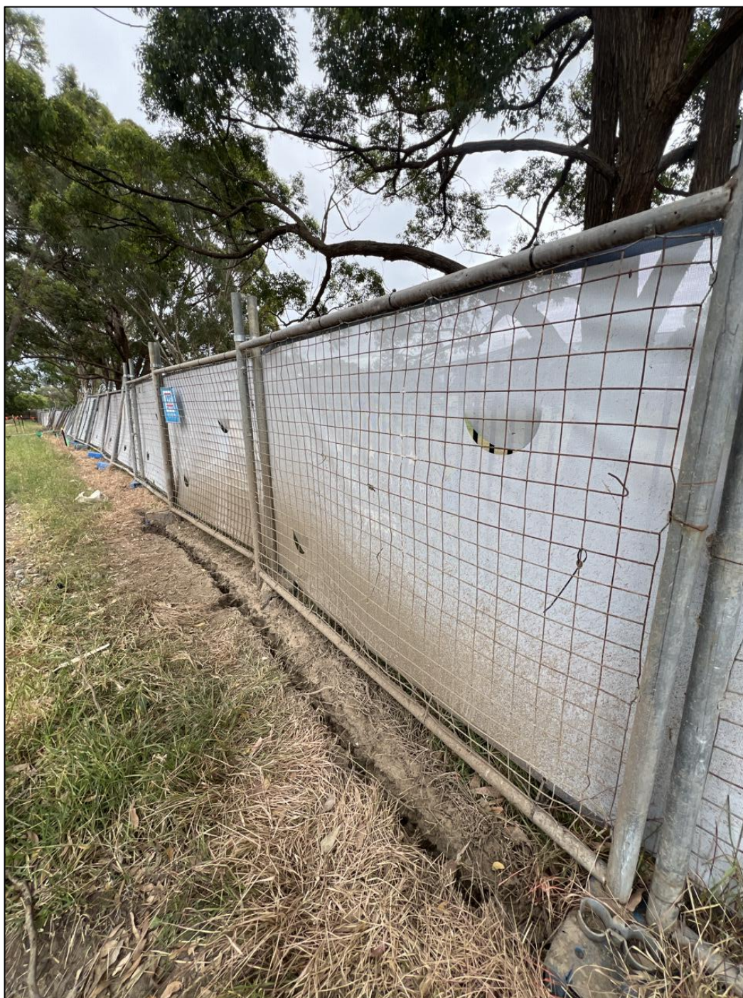
Figure 33. Trench 8 with no major or minor roots encountered. Image taken from eastern edge of trench.
