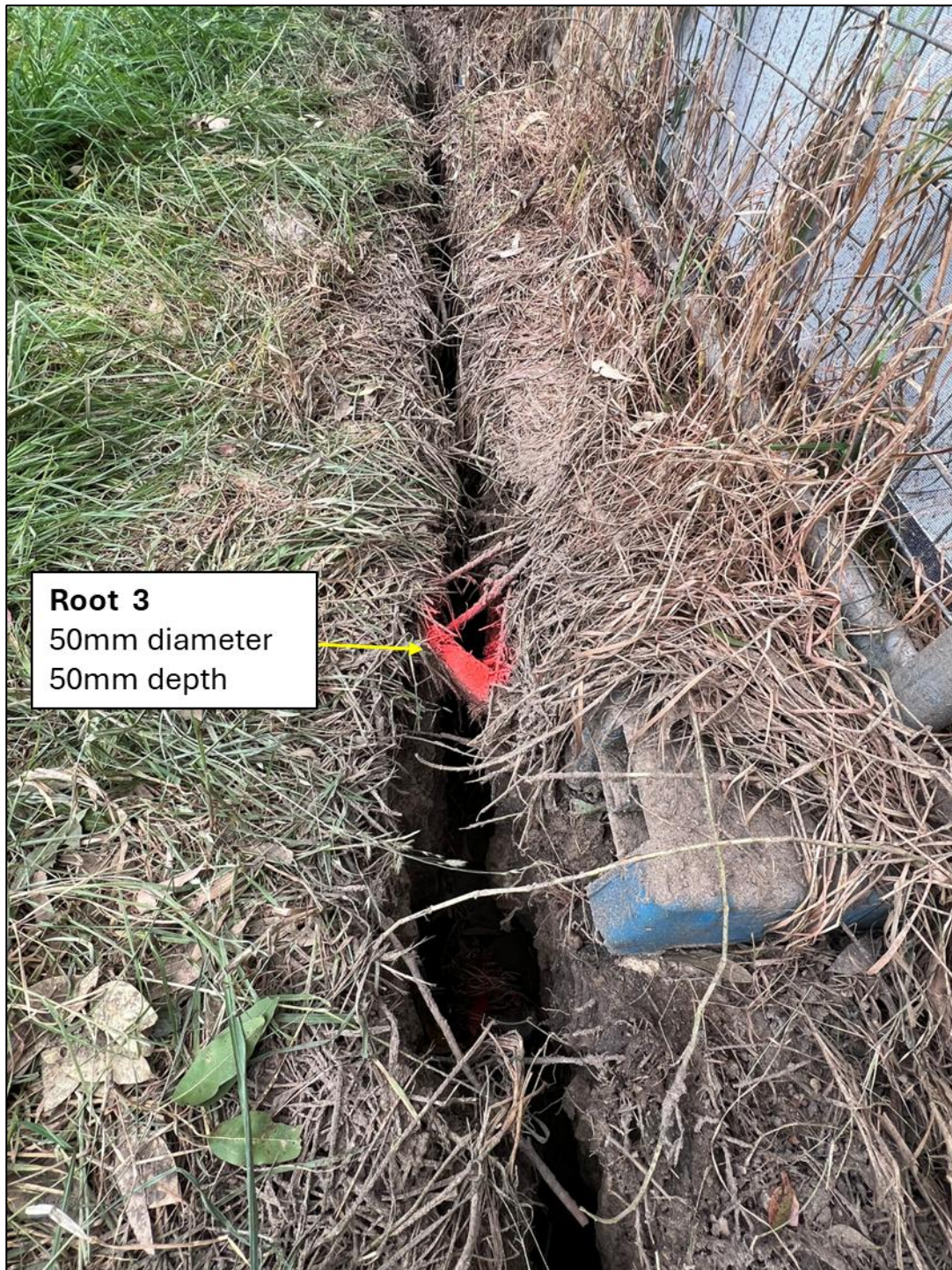
Figure 40. Root 3 within central portion of Survey Trench 10. No major roots observed within western portion of trench.
