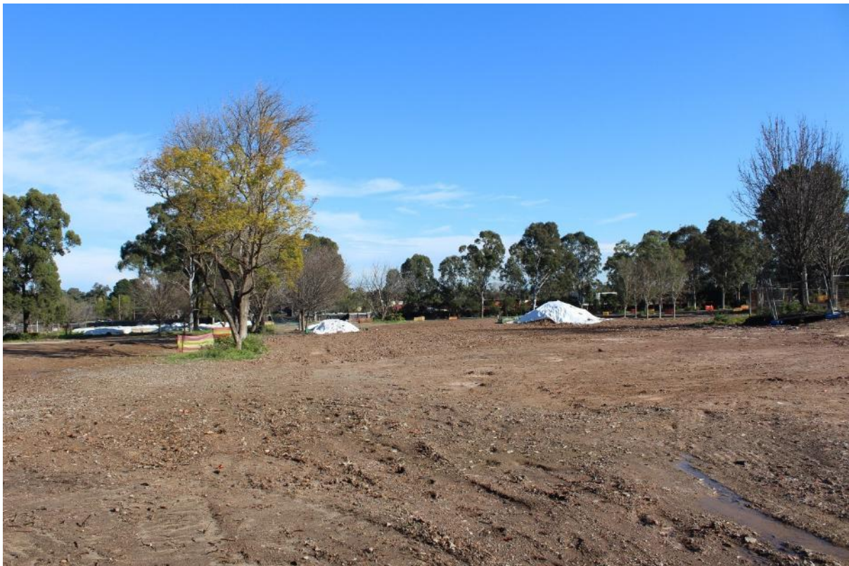
Plate 6. Good visibility showing clay/sand with building rubble, following demolition of former buildings in SU2. (Source: Heritage Now 2025)
