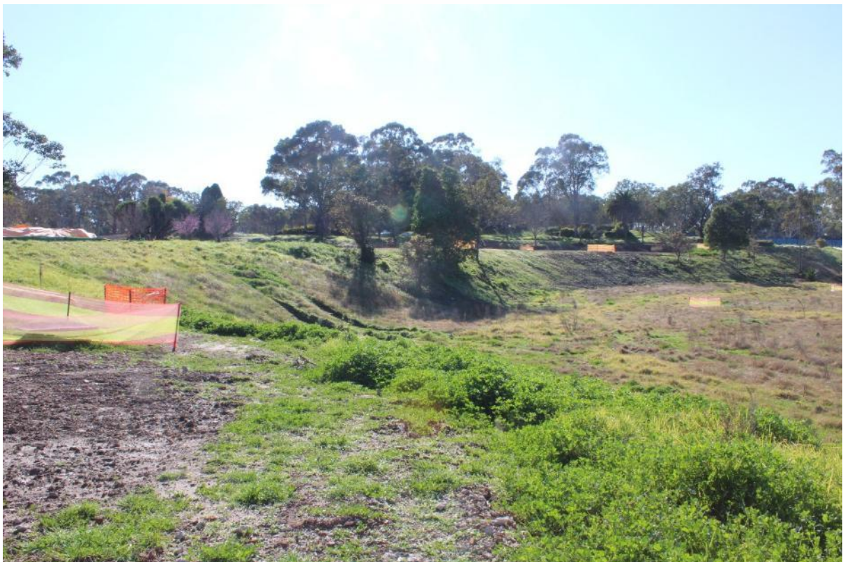
Plate 8. Major earthworks/landscape modification to build up the landform above the low-lying south-western portion of the Project Area. (Source: Heritage Now 2025)
