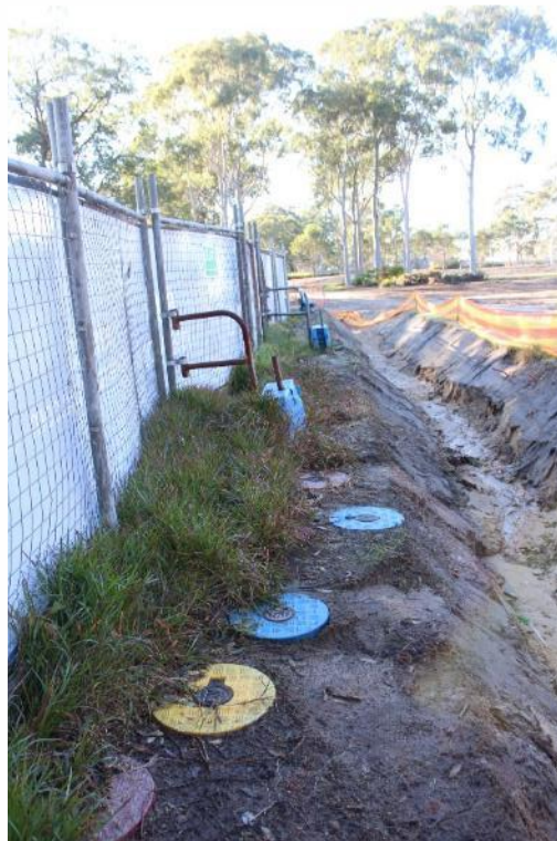
Plate 7. Evidence of services and drainage trench in the western part of the Project Area (SU2). (Source: Heritage Now 2025)
