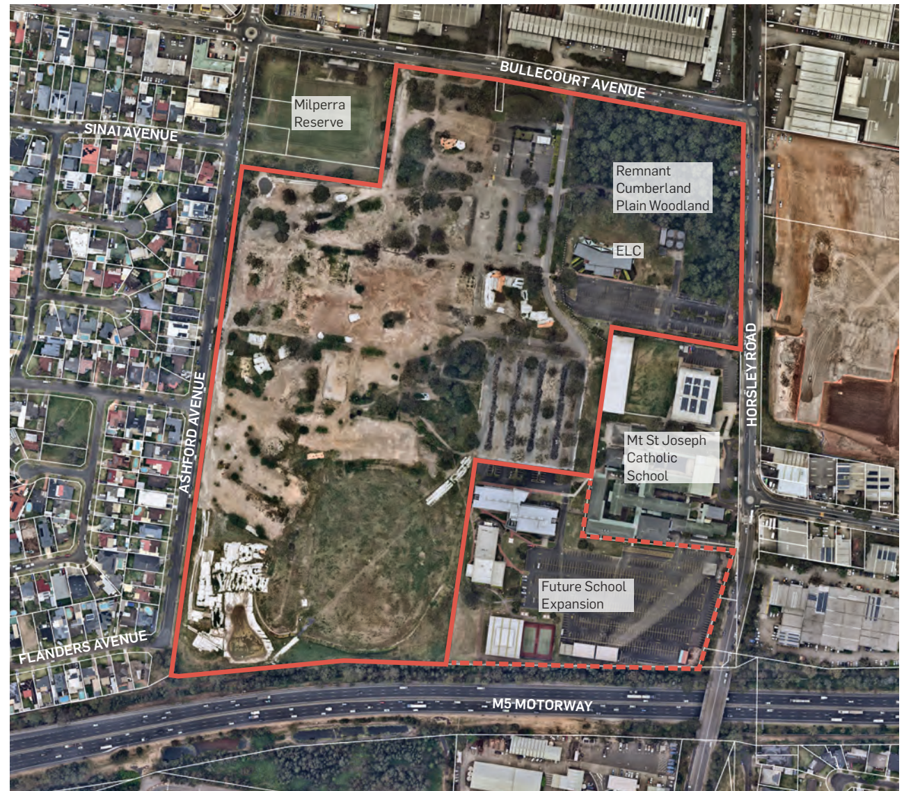
Figure 2 Existing Site Condition
