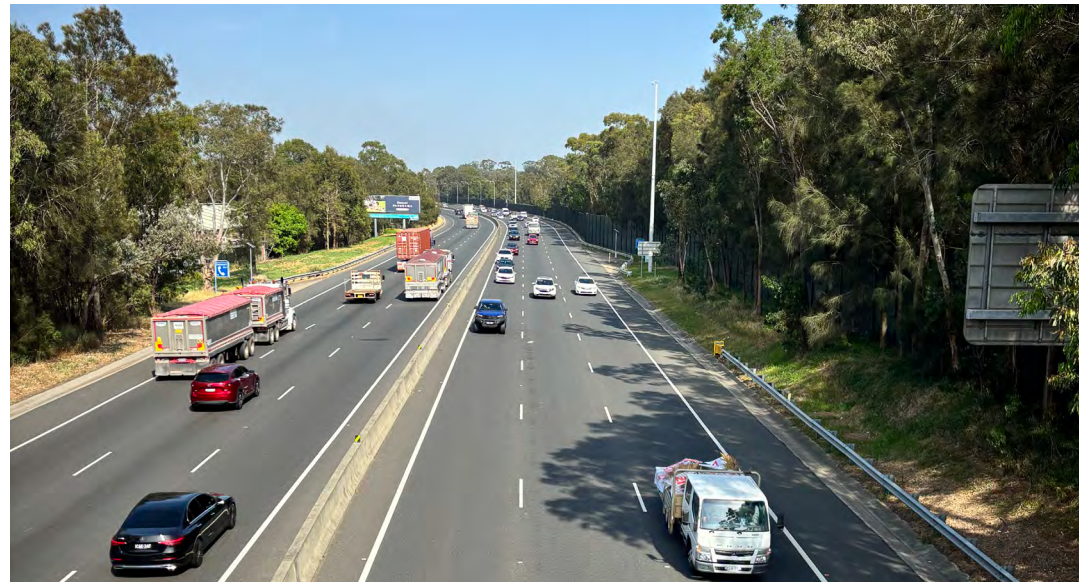
Figure 27 View west of M5 from Horsley Road bridge.
