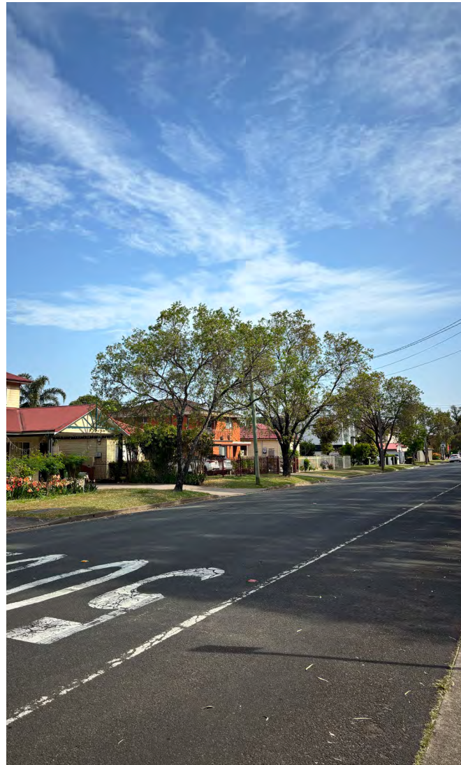
Figure 22 View north along Ashford Ave.
