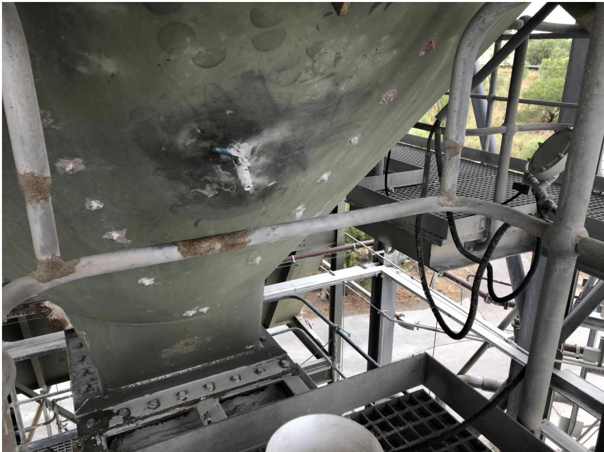
Figure 3 Bayswater Power Station – Silo A Fly Ash Sampling Point (a similar sampling point is located at Silo B)
