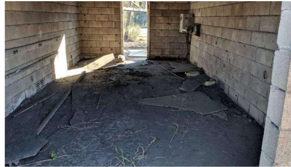
Photo 8: Potential ACM sheeting within abandoned concrete building – intersection of ash pipeline and Liddell Station Road
