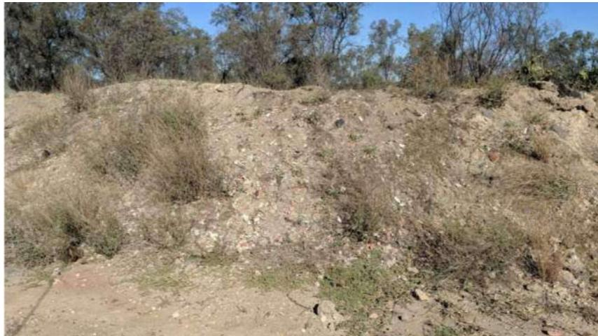
Photo 2: Stockpiles of silty clay fill with anthropogenic materials – Former Contractor Storage Area
