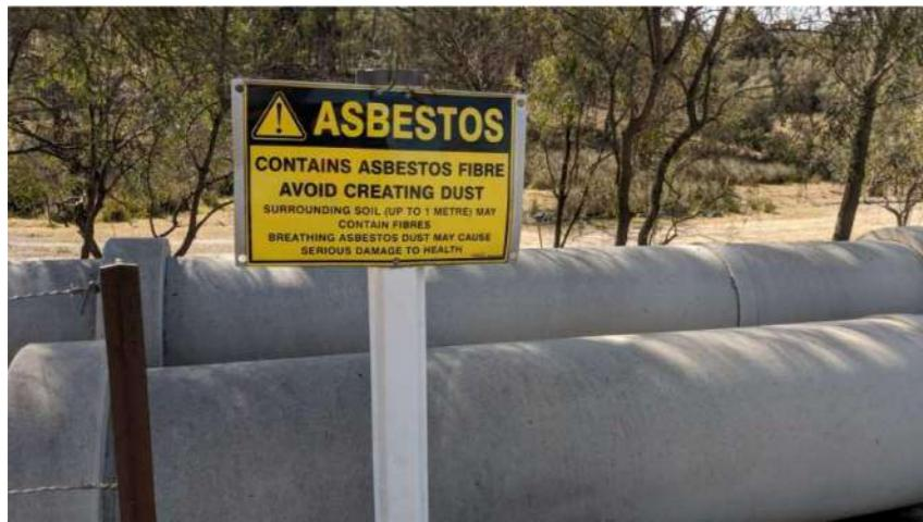
Photo 1: Signage for ACM piping - north of the Fly Ash Plant
