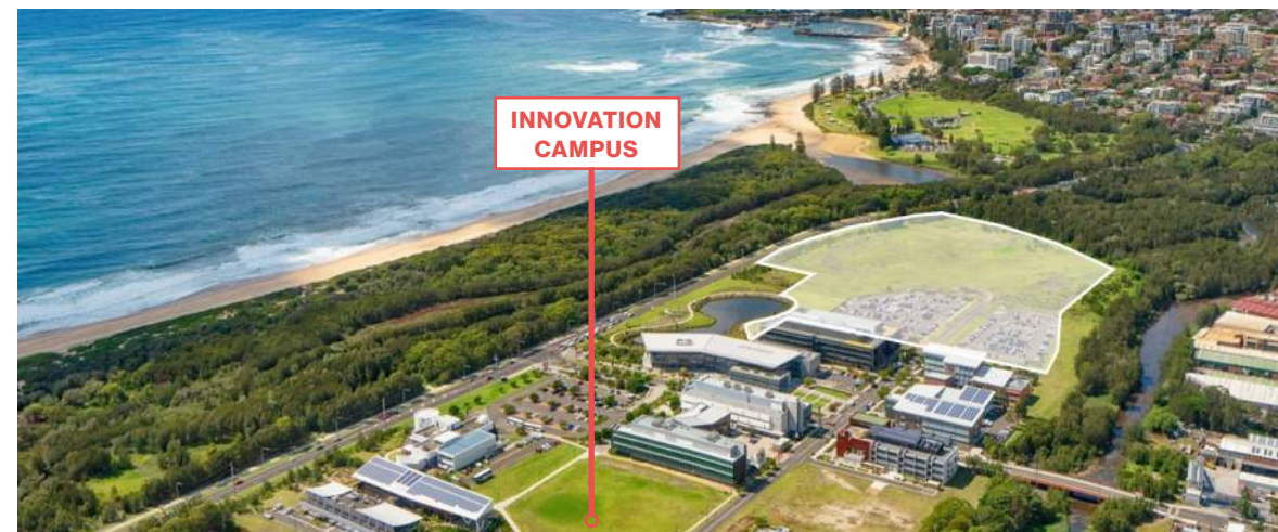
View looking south- east with Fairy Creek, Fairy Meadow Beach, Wollongong CBD in the background
