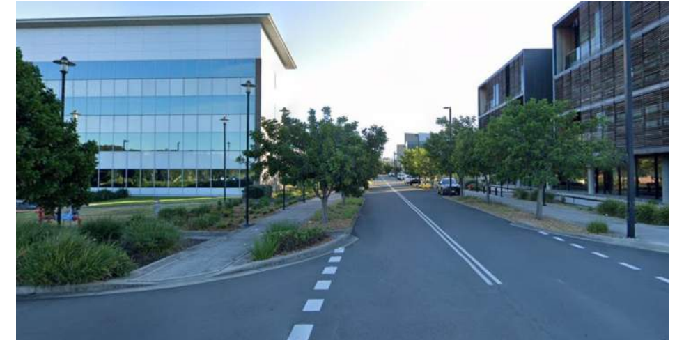
2. View looking north towards 4-5 storey university buildings setback from road - dense street tree plantings
