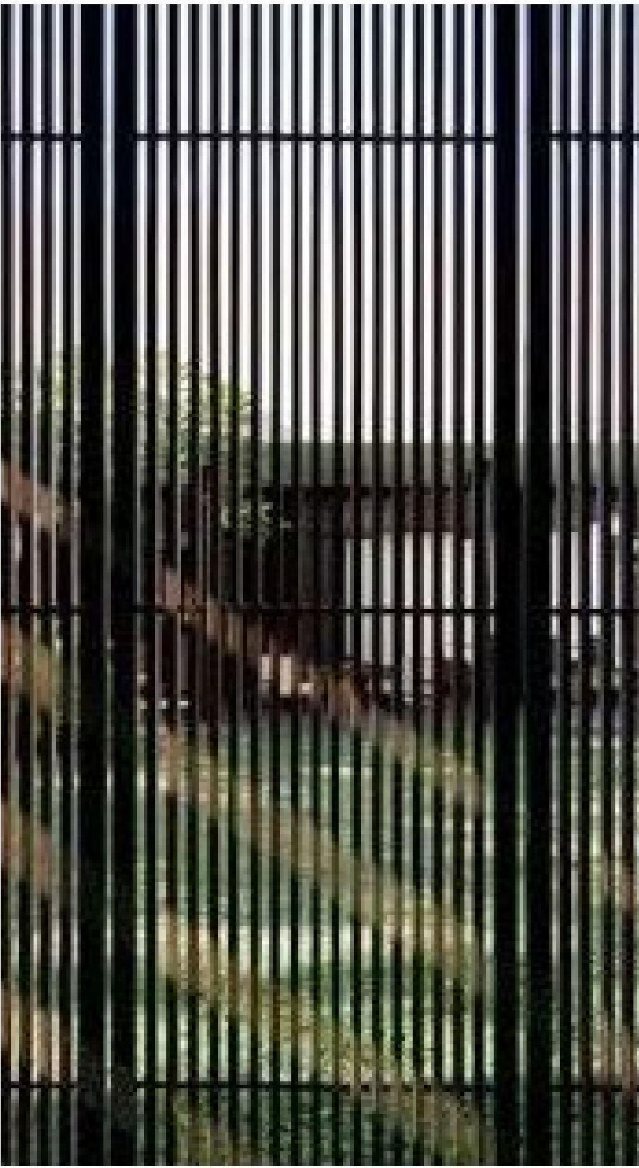
Louvers to Provide Privacy, Assure Ventilation and Conceal Parking
