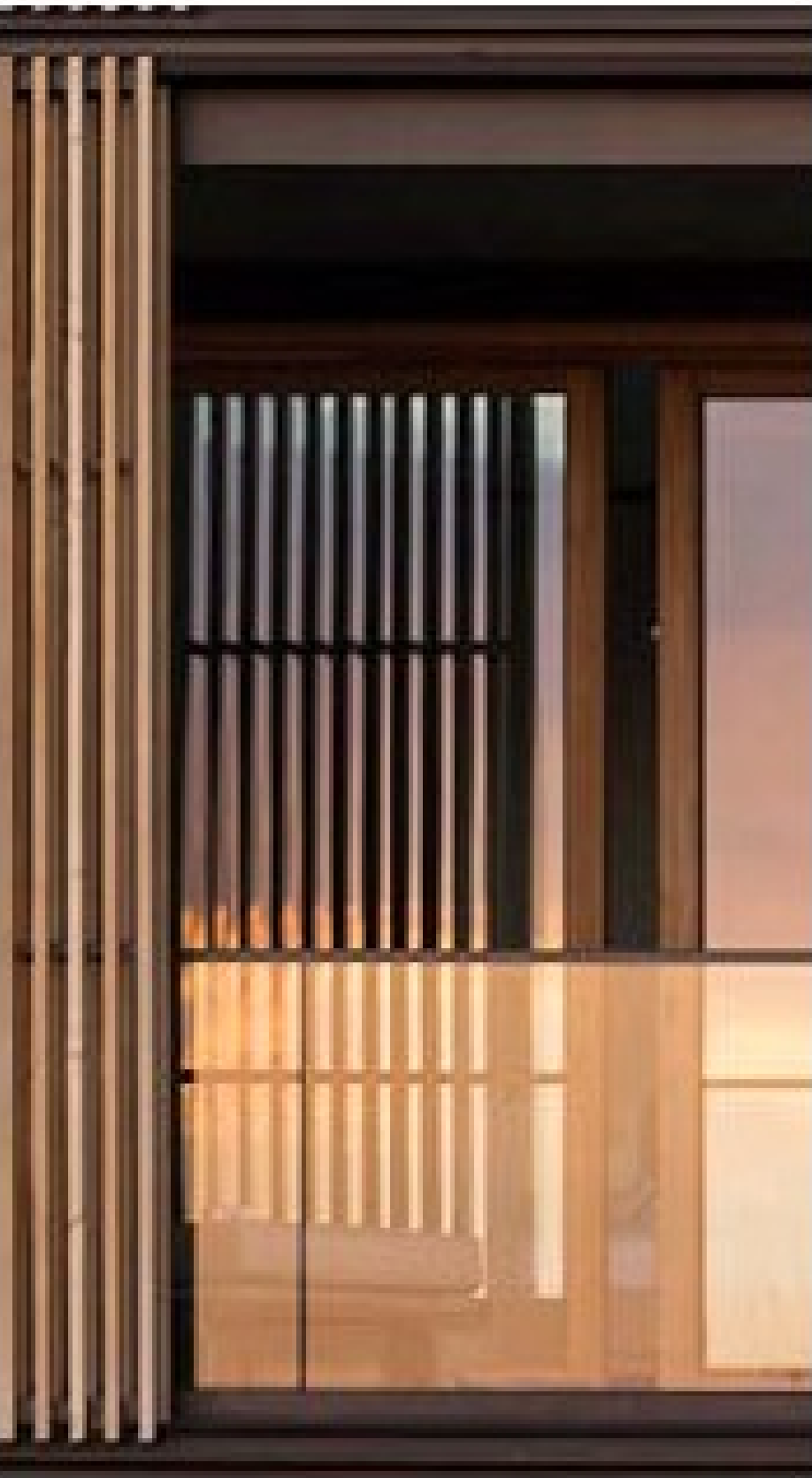
Louvers and Sun Control
