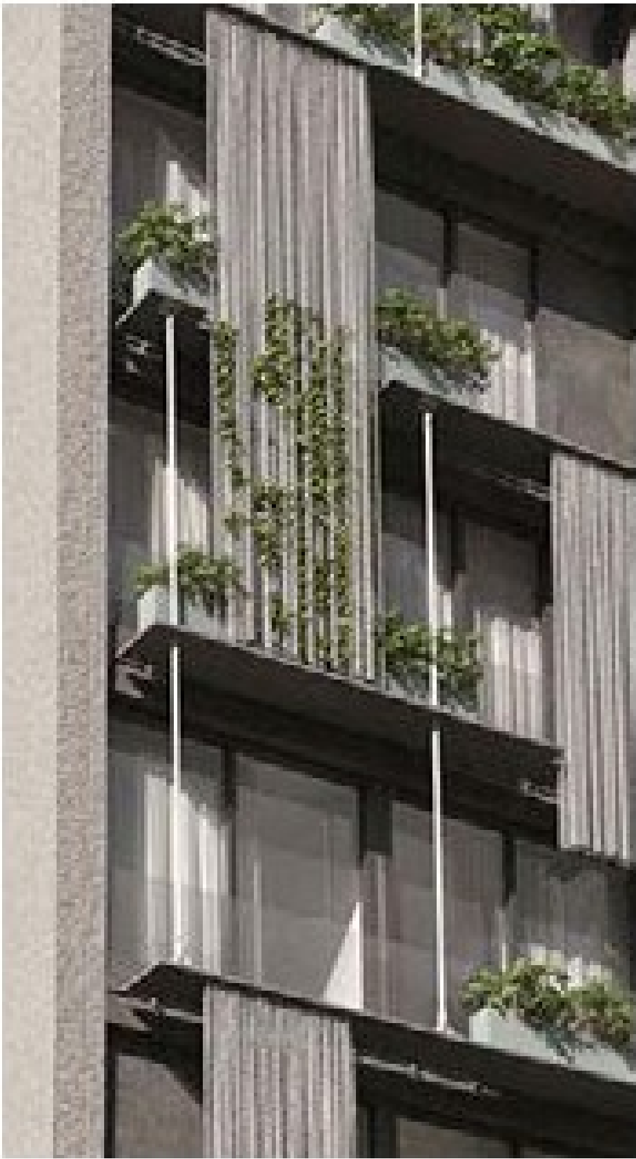
Projected Structure to Provide Adjustable Shading
