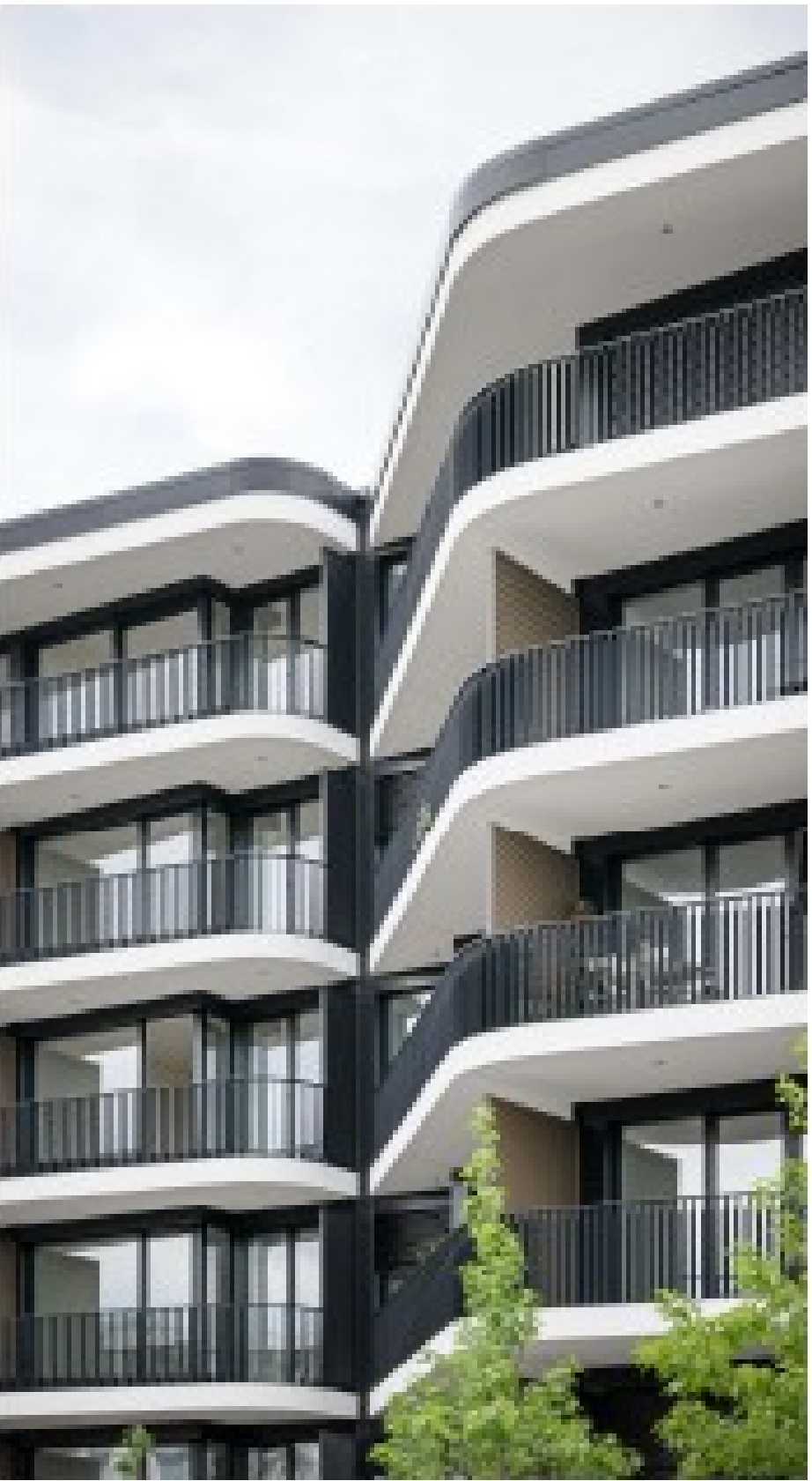
Curvature of Ocean Side Balconies
