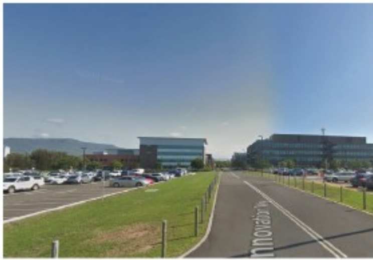
Streetview, Innovation Way, Looking North
