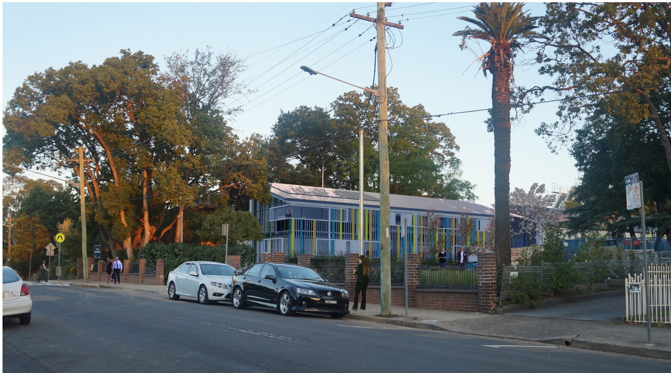
Street View looking East
