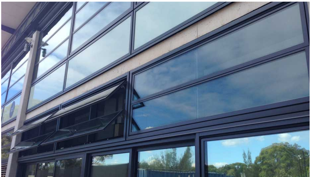
Figure 14: EBSA MP2 glazed louvre system
