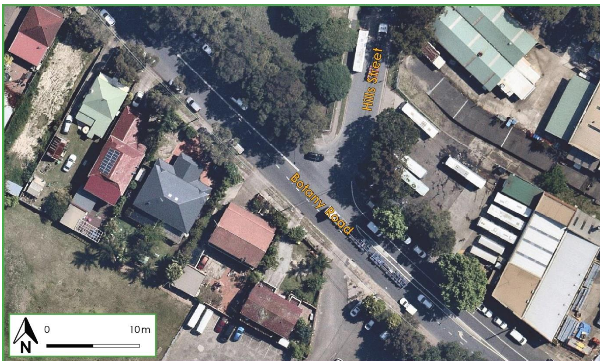
Figure 6: Intersection of Botany Road and Hills Street
