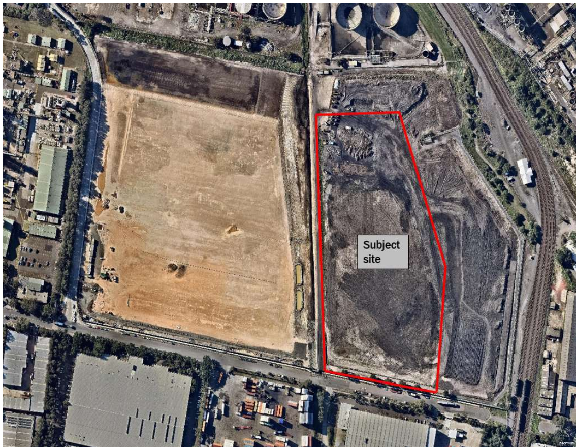
Figure 10: Earthworks activities on the site in March 2015 (Base source: Nearmap)
