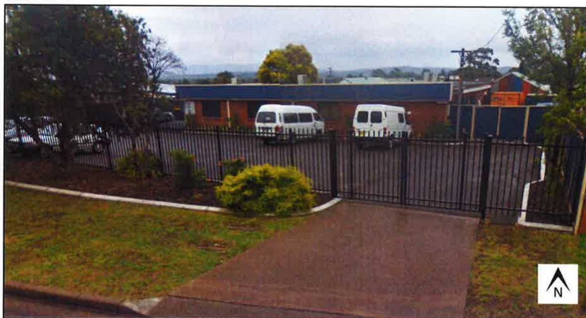
Figure 3 | Site as viewed from James Street (Source: Applicant's Environmental Impact Statement (EIS))
