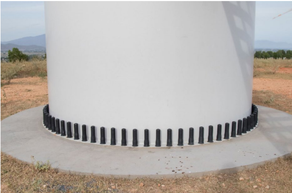
Figure 3-10 Typical Wind Farm Tower Foundation
