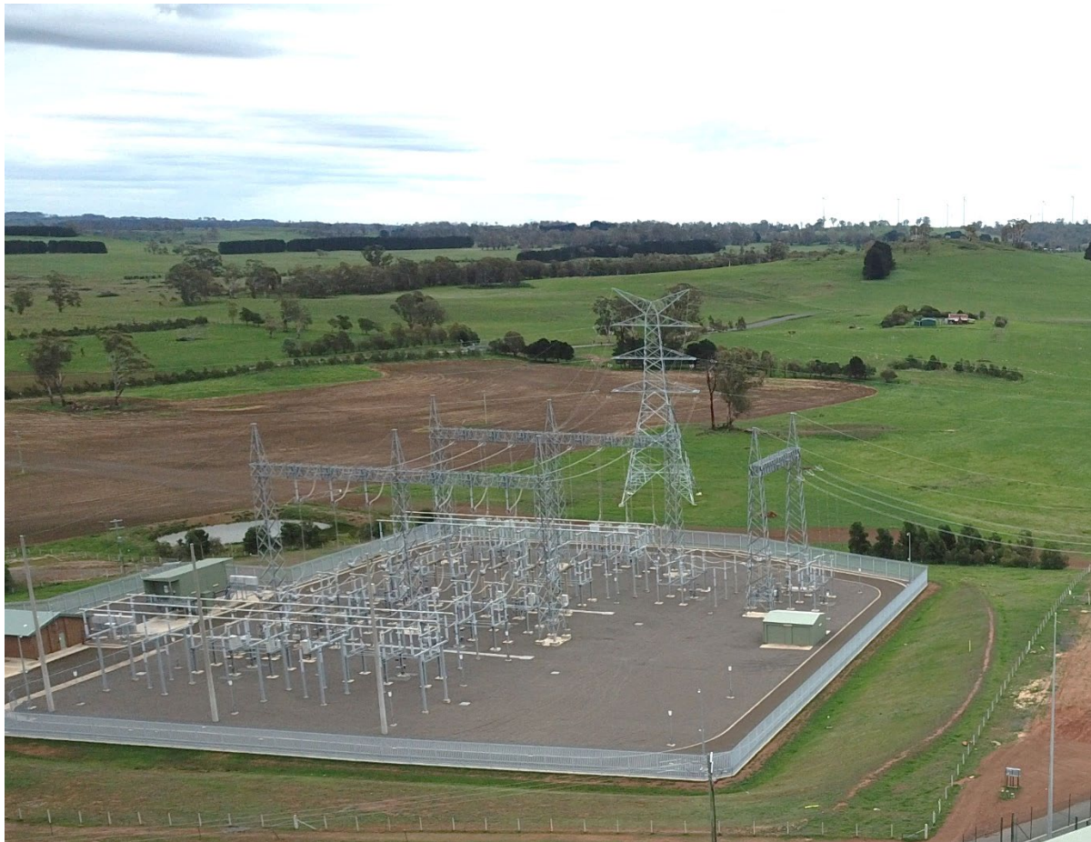
Figure 3-14 Typical Switching Station – Gullen Range Wind Farm 330 kV Switching Station
