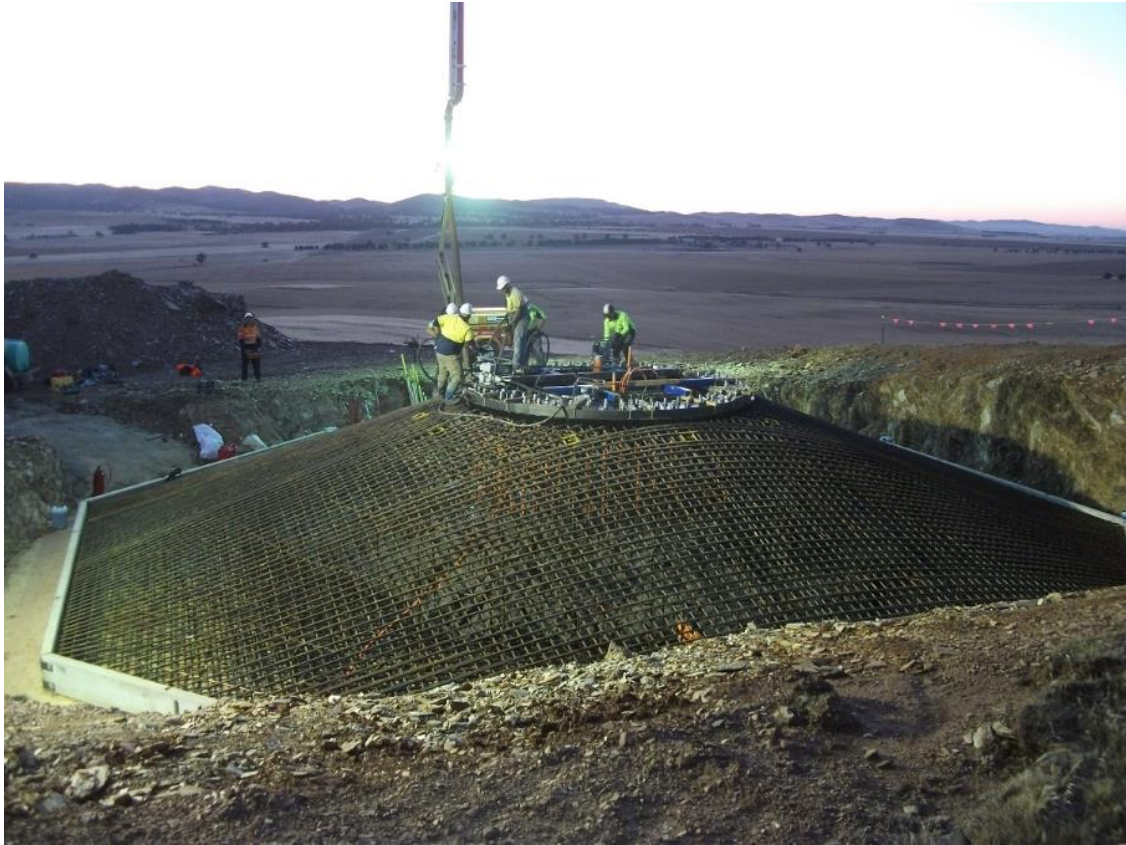
Figure 3-9 Typical Gravity Foundation for a Wind Farm (ENGIE Willogoleche Wind Farm in construction)
