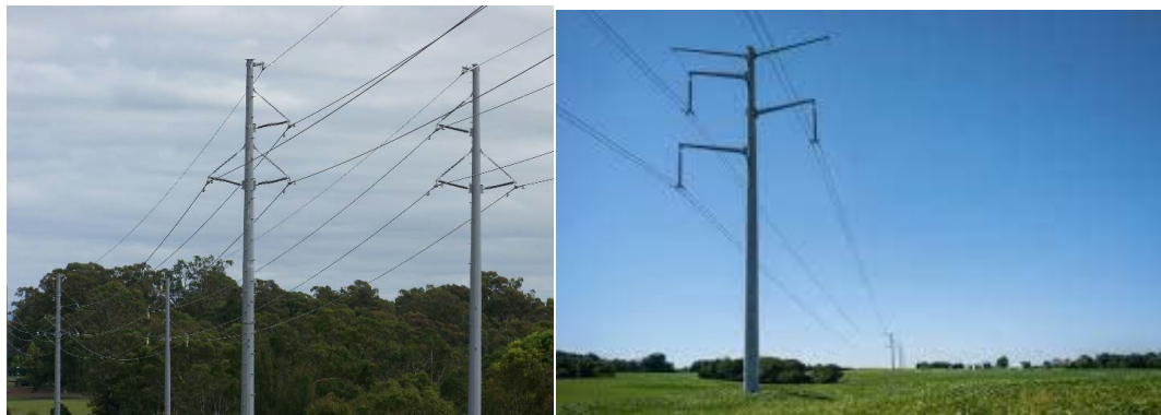
Figure 3-11 Typical Steel Pole Structures, Transmission Line
