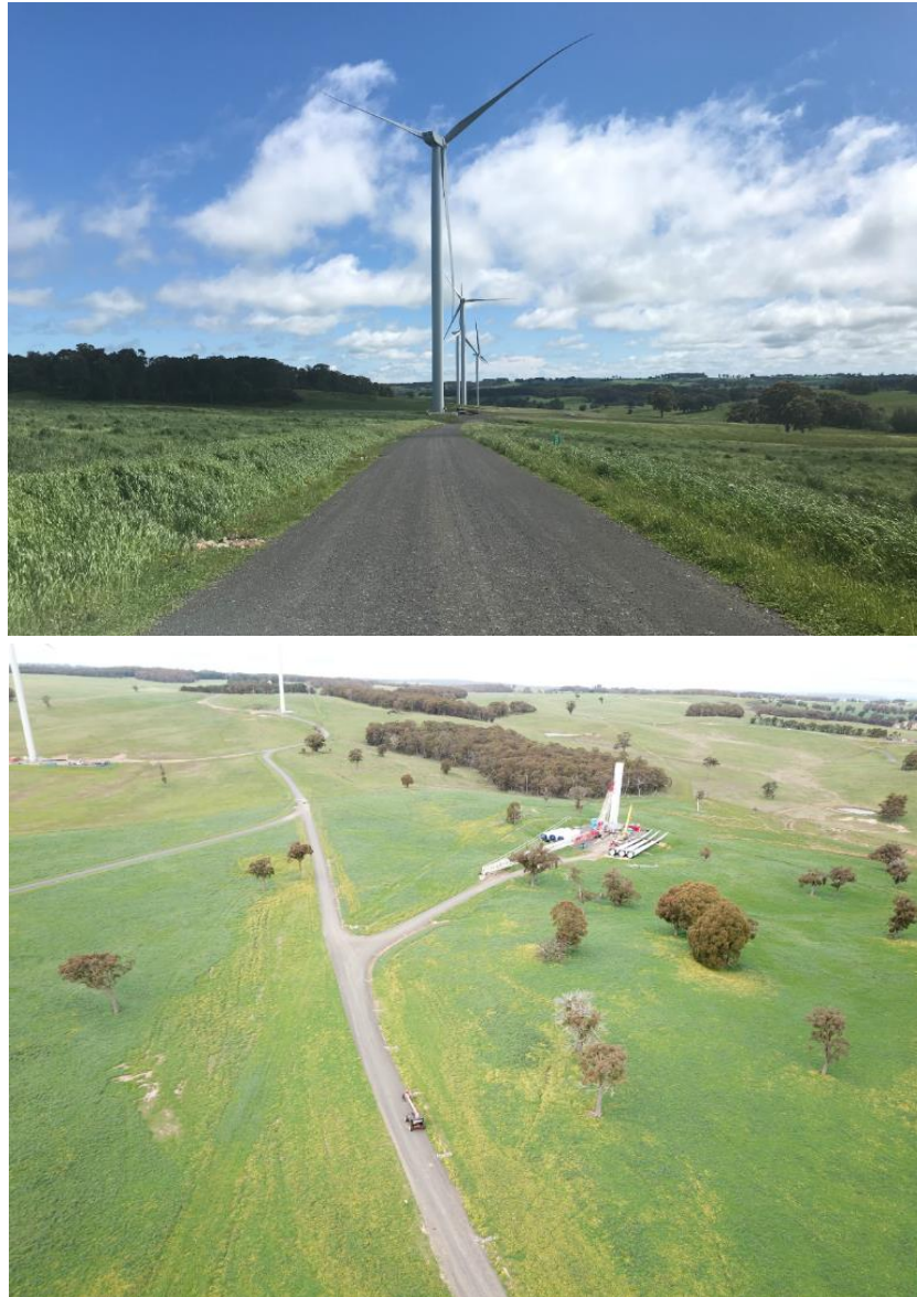
Figure 3-24 Examples of Rehabilitation of Road Batters and Verges – Biala Wind Farm
