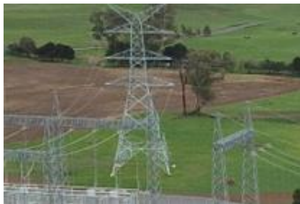
Figure 3-12 Typical 330 kV Lattice Tower
