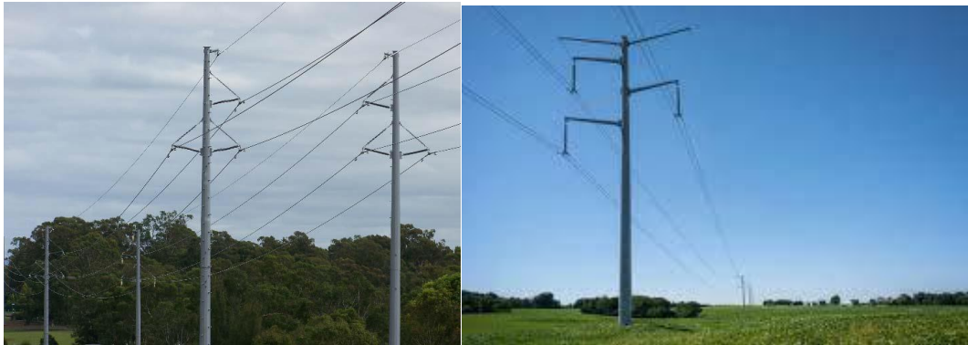
Figure 3-11 Typical Steel Pole Structures, Transmission Line
