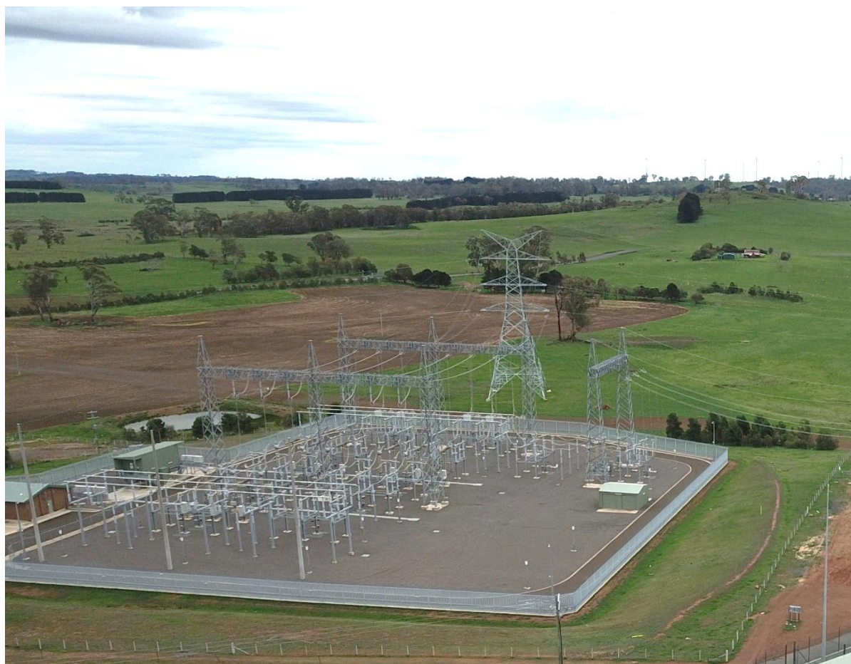
Figure 3-15 Typical Switching Station – Gullen Range Wind Farm 330 kV Switching Station
