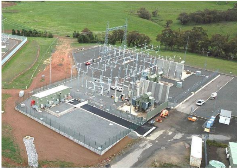
Figure 3-13 Typical Substation - Gullen Range Wind Farm 33/330kV Substation
