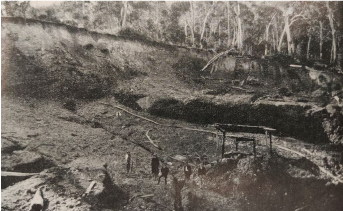
Photograph 3.8 Mount Sheba Gold Mine c.1888, lengths of hose used for carrying water to sluicing hydrants shown (Bayley 1953: 43)
