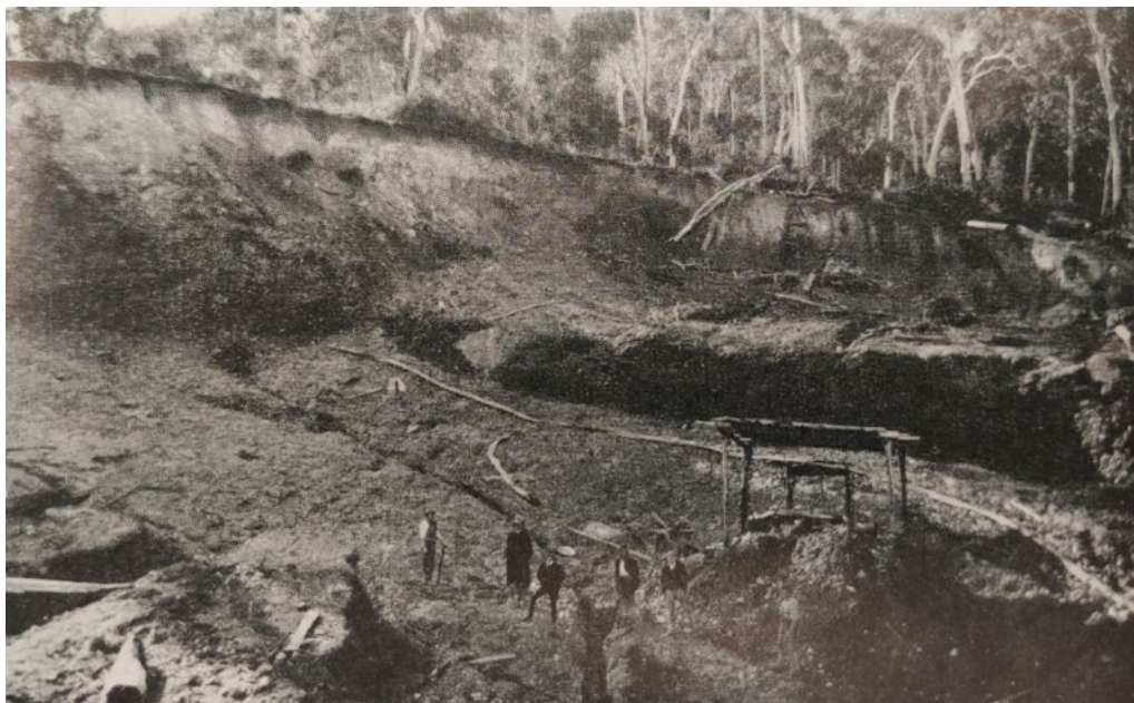
Photograph 4.12 Mount Sheba Gold Mine c.1888, lengths of hose used for carrying water to sluicing hydrants shown (Bayley 1953: 43)
