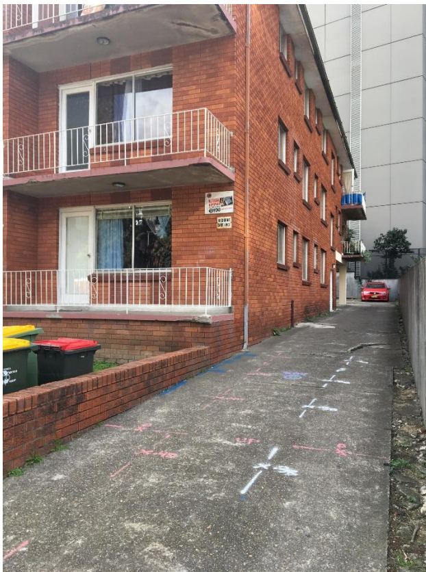
Figure 4.6: Looking northwest along the concrete driveway located on the eastern side of the apartment block providing access to parking at the rear of the building. (Casey & Lowe 2018).
