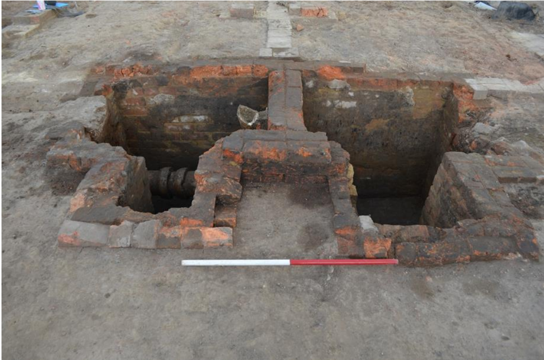
Figure 3.6: Cesspits at rear of No. 16-18 Darcy Street (4&6PS), showing later earthenware sewerage pipe (left) as part of the conversion to plumbed toilets. Looking south, 1m scale (Casey & Lowe 2016).
