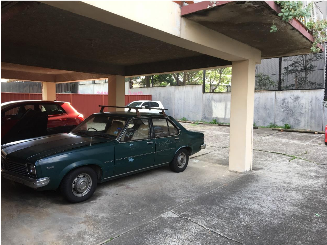
Figure 4.7: Looking northwest at the ground level car parking at the rear of the apartment block including some undercover spaces. (Casey & Lowe 2018).
