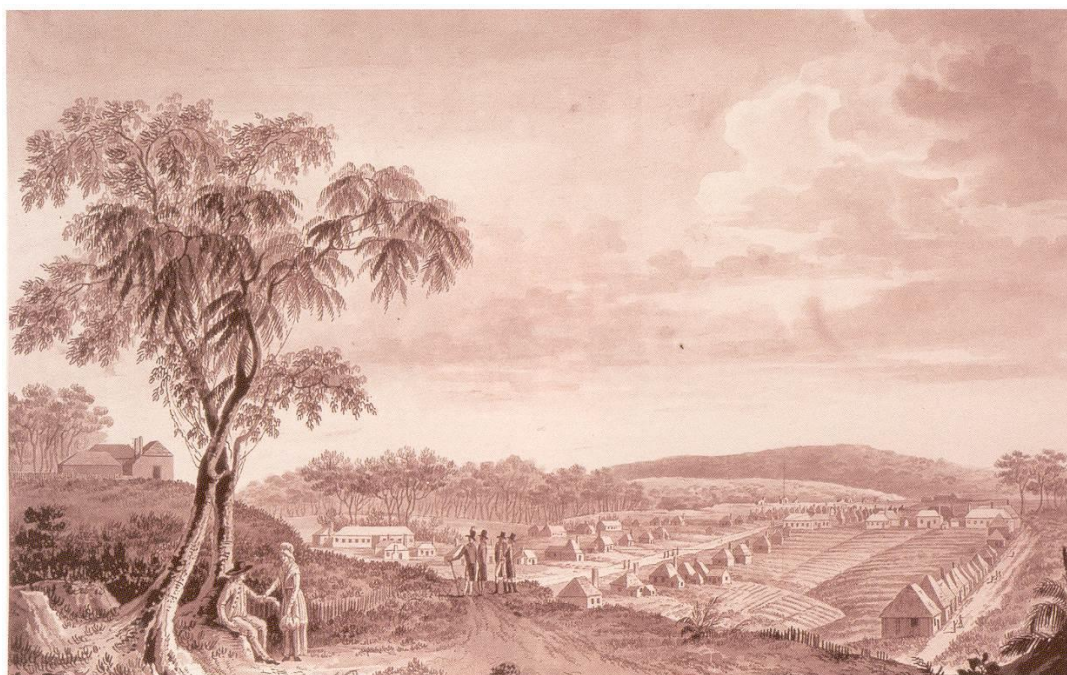
Figure 2.1: Fernando Brambila's 1793 view of George Street showing convict huts aligned with George Street (middle ground) and Government house (middle left). The study area is a 100m or so outside of this viewpoint and to the right. British Library, maps T.TOP.124 Supp F44.
