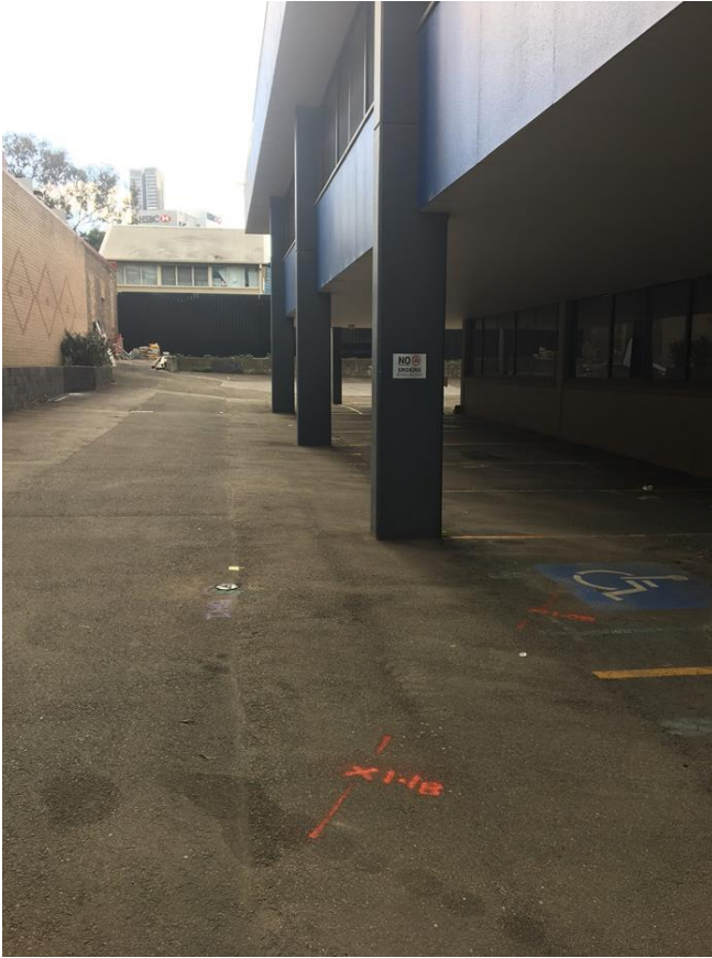
Figure 4.2: View looking north along the access to the rear car park. Note that the carpark surface is slightly raised to the west. The piers support the upper floor of the building allowing for additional undercover parking along the accessway. (Casey & Lowe 2018).
