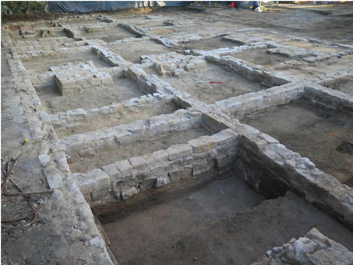
Figure 3.9: Footings from 1870s houses on Harris Street. These contained no underfloor deposits but beneath the houses was evidence of fill to raise this area about surround flooding.
