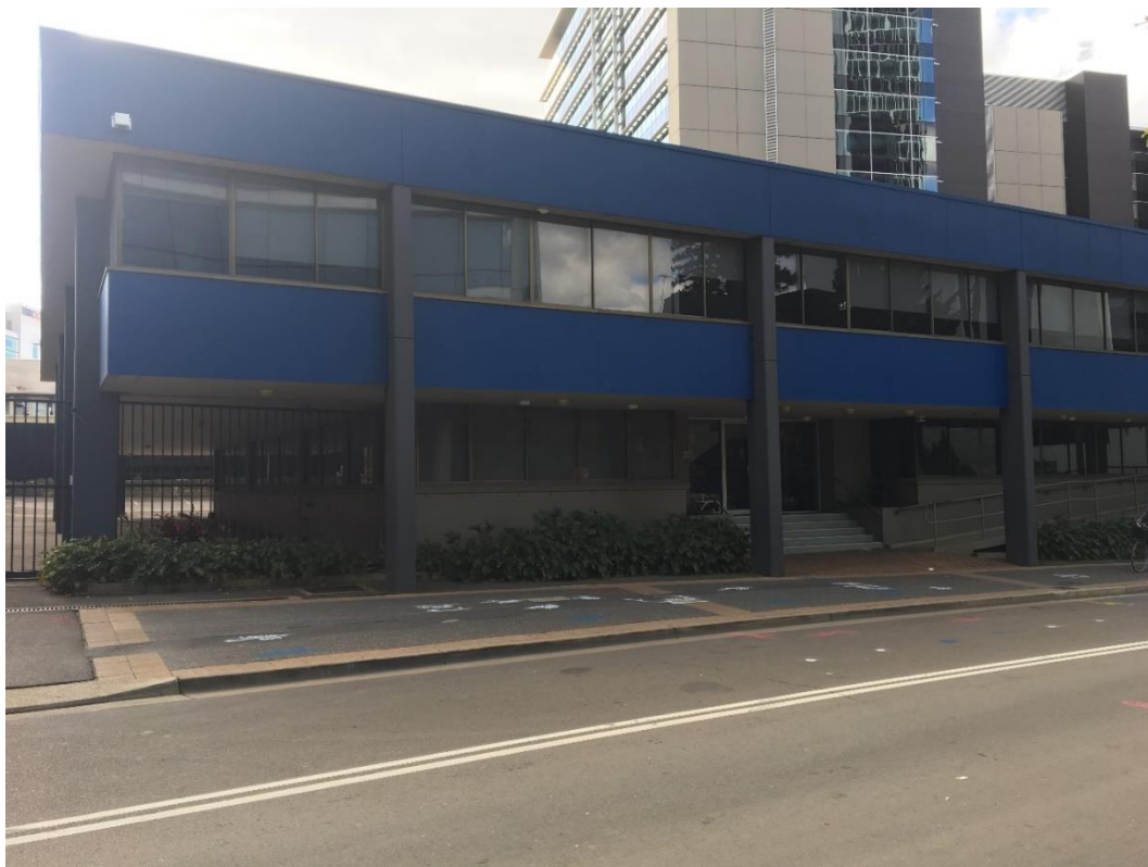
Figure 4.1: Photo showing existing two-storey building at No. 2 Hassall Street looking northeast. The ground floor is raised above street level so that the building itself sits higher than the street and footpath. (Casey & Lowe 2018).
