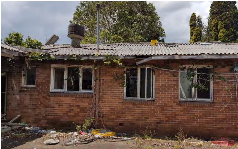
Photo 7 Former Army Compound (Building 1)
