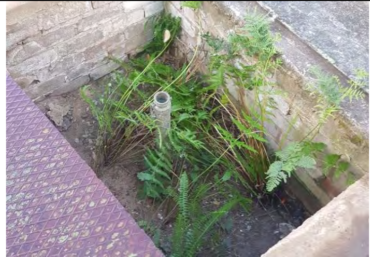
Photo 2 Former Army Compound – UST 1
