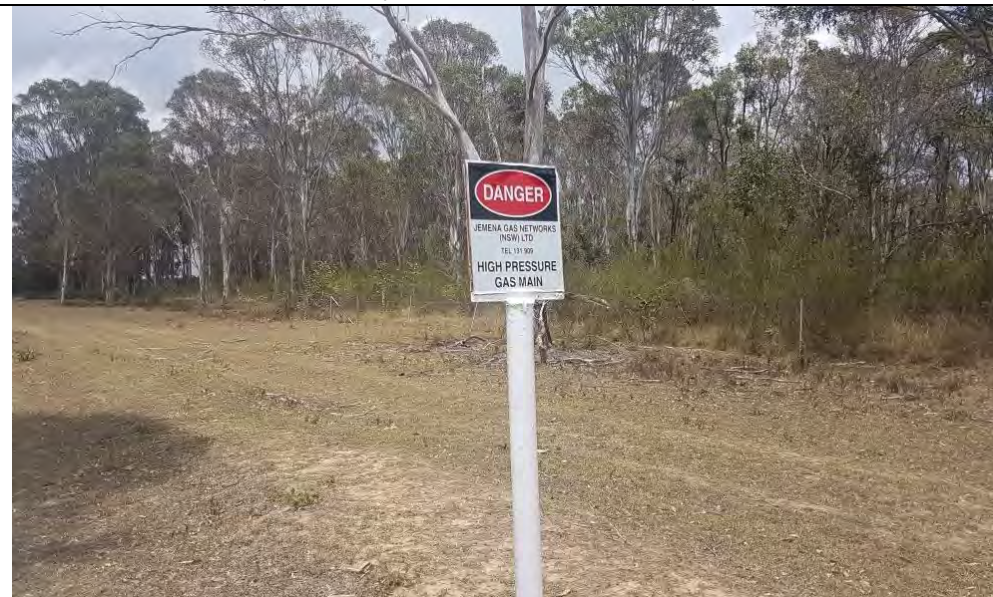
Photo 20 High pressure gas main
