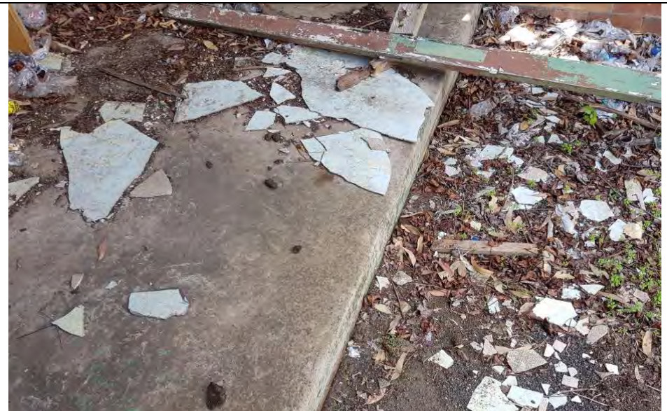
Photo 8 Asbestos fragments near Building 1 of Former Army Compound
