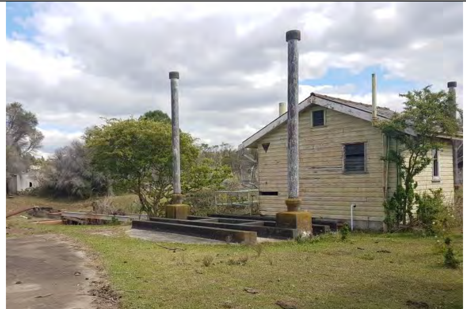
Photo 10 WWTP Control room, primary sedimentation tank, and distribution pit
