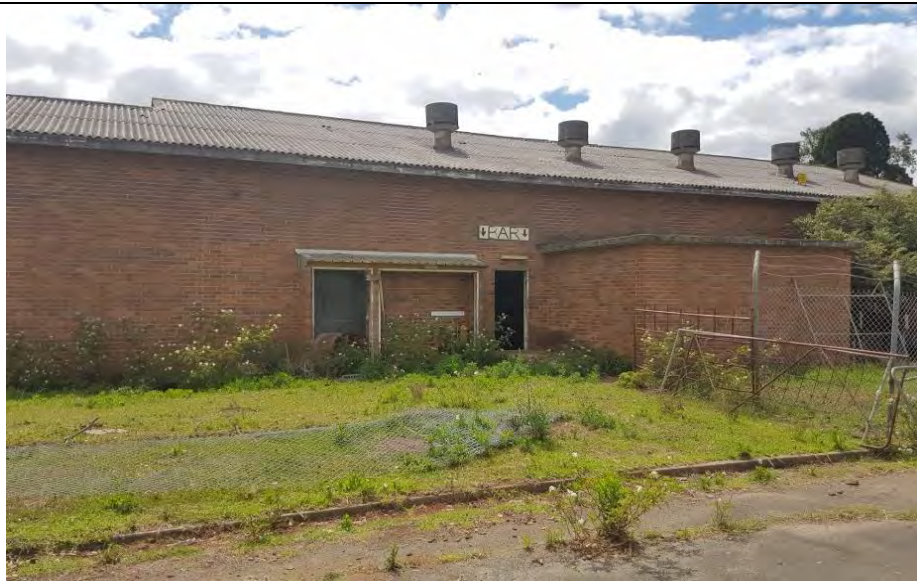
Photo 5 Former Army Compound (Building 2)
