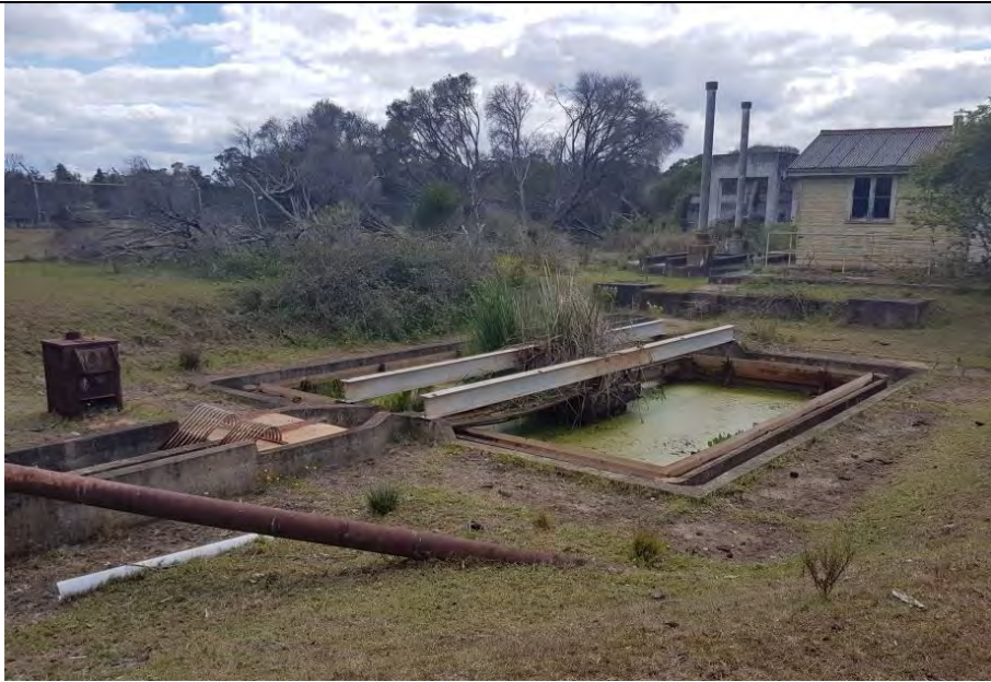
Photo 9 WWTP – Grit Chamber
