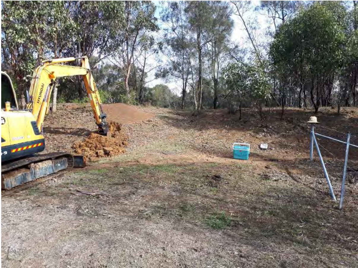
Plate 1 – DTP1 positioned in farm dam 1 wall
