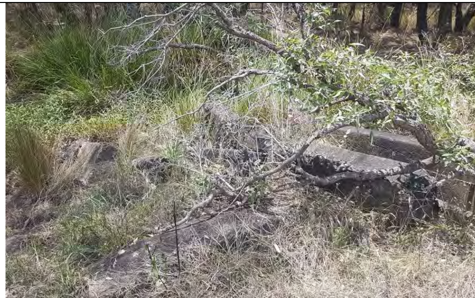
Photo 18 Pile of rubble (near the dry pond on the east of the site)
