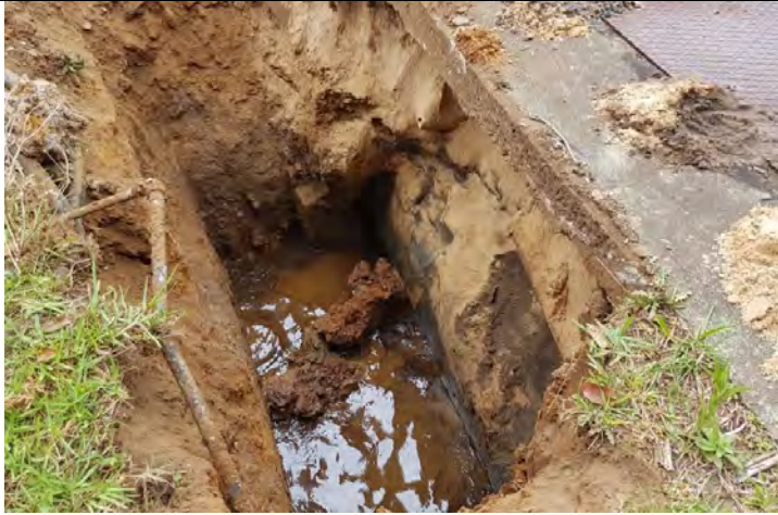
Photo 3 Former Army Compound – TP3 and UST 2
