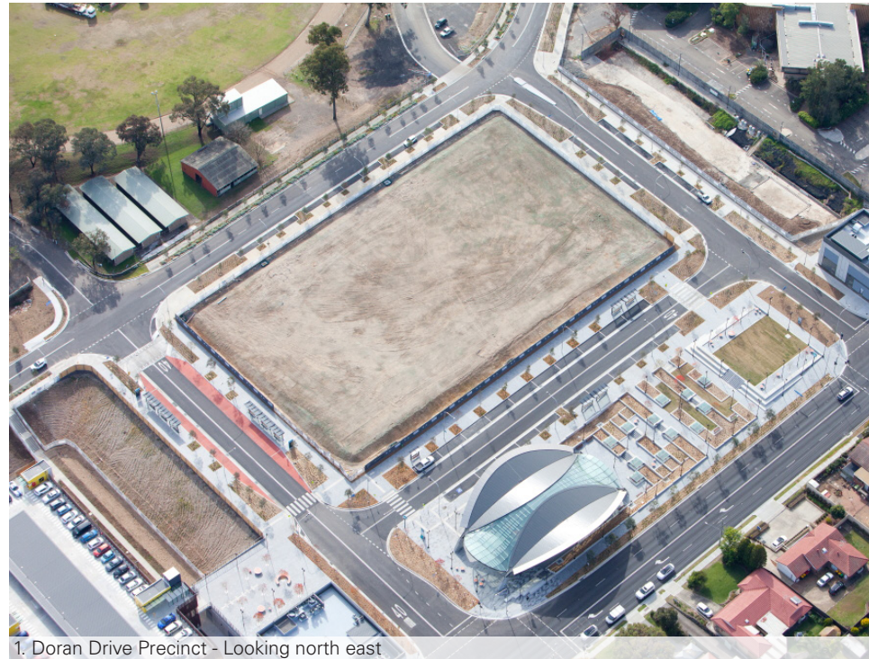
1. Doran Drive Precinct - Looking north east
