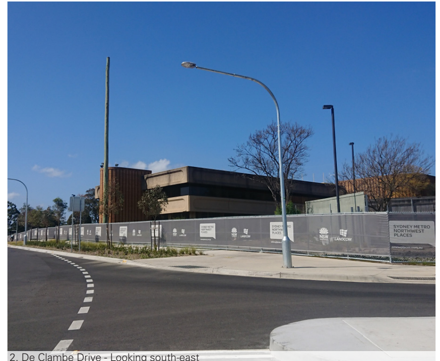
2. De Clambe Drive - Looking south-east
