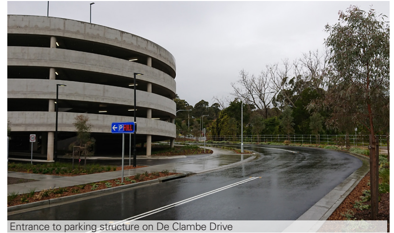
Entrance to parking structure on De Clambe Drive
