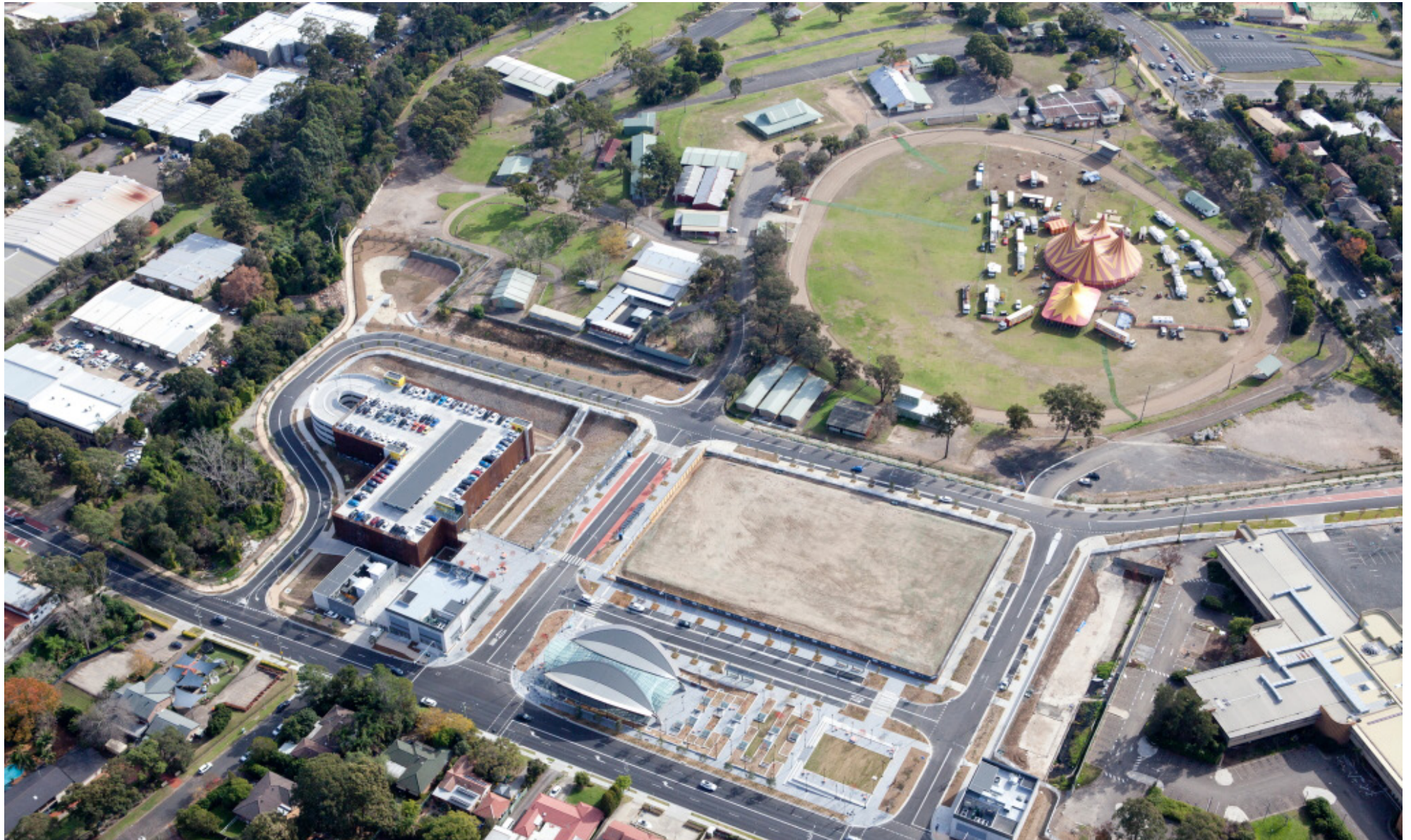
Hills Showground Station Precinct (foreground) and Castle Hill Showground (background) Aerial looking north west
