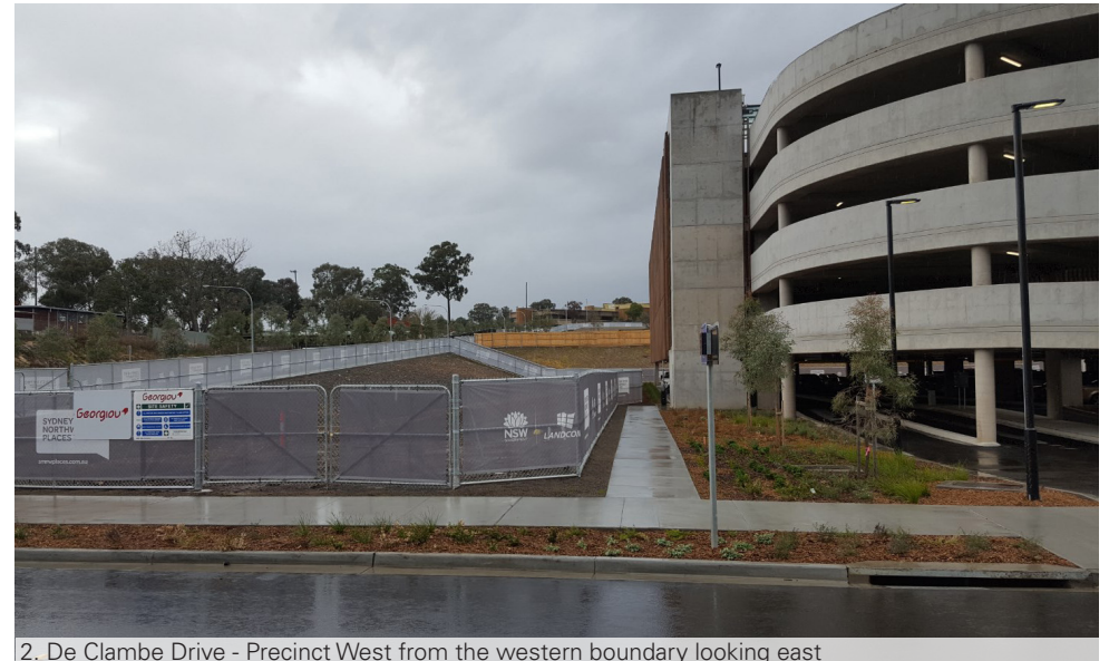
2. De Clambe Drive - Precinct West from the western boundary looking east
