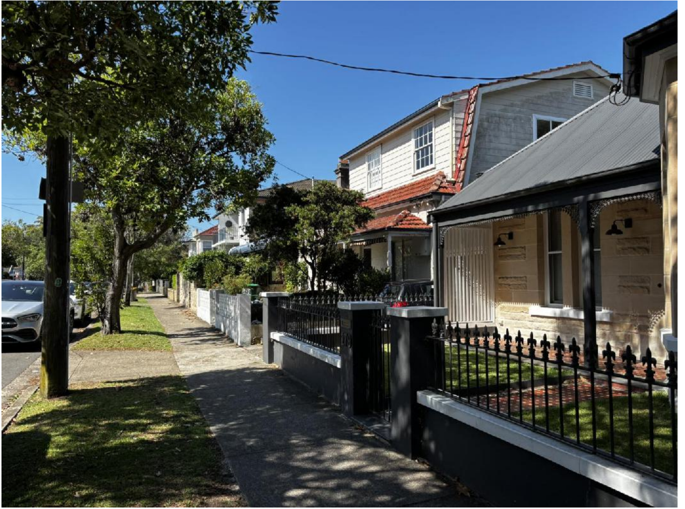
Figure 18 Development on the eastern side of West Street
