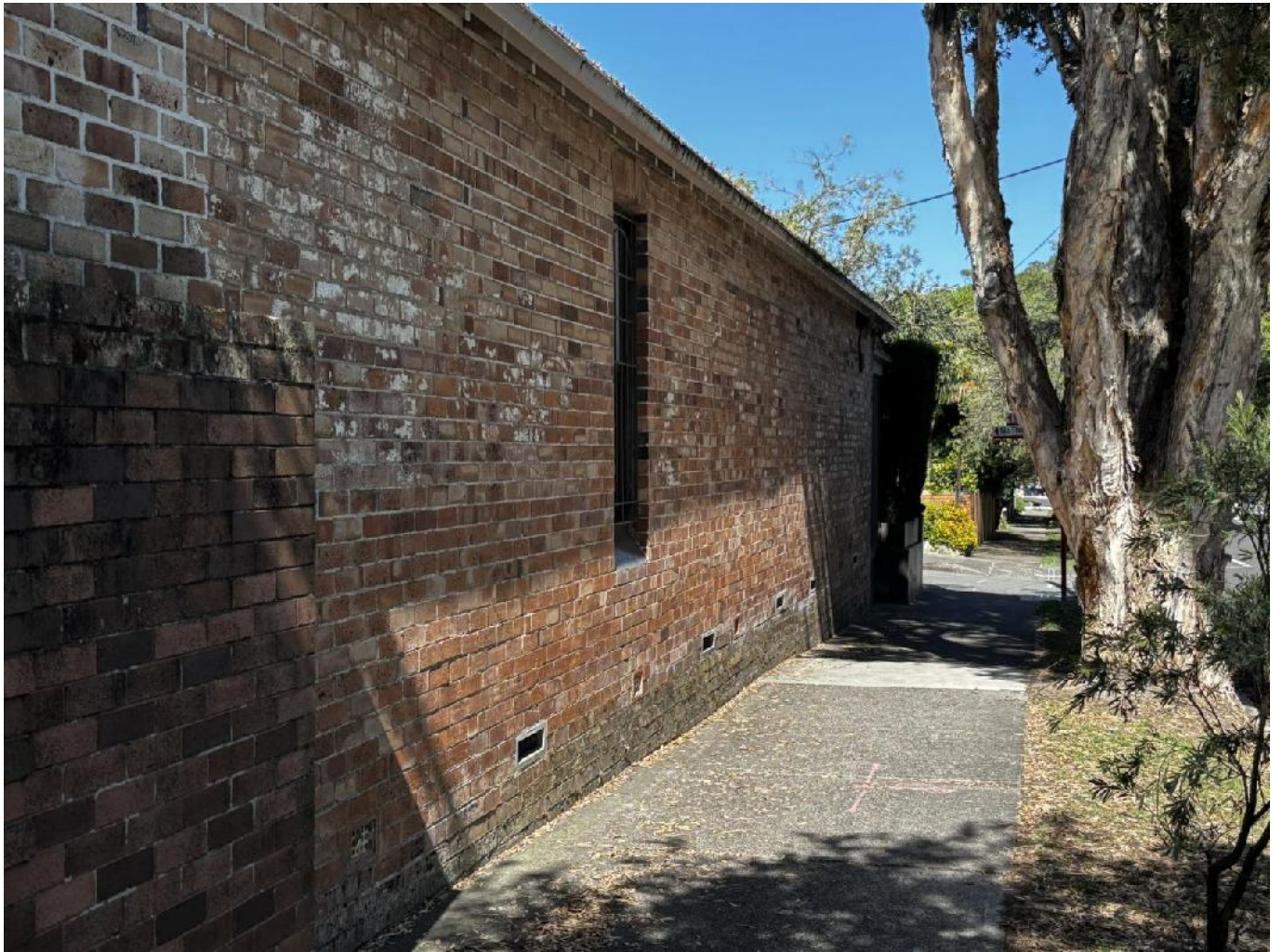
Figure 12 Development opposite the site
