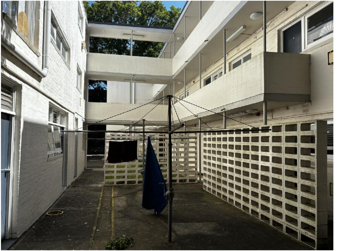
Figure 4 Space within the 'U' of a building block
