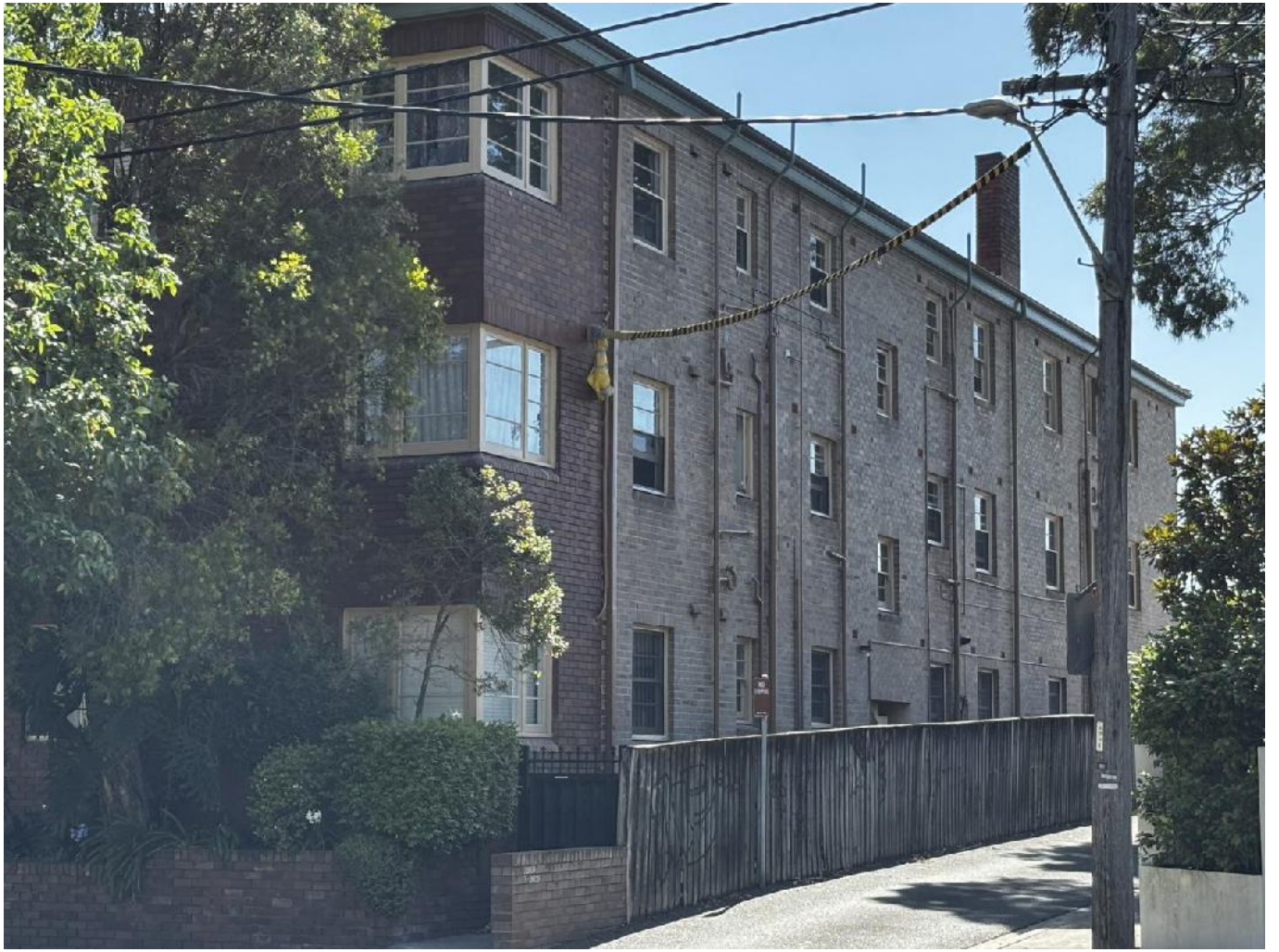
Figure 20 Residential flat building on the western side of West Street
