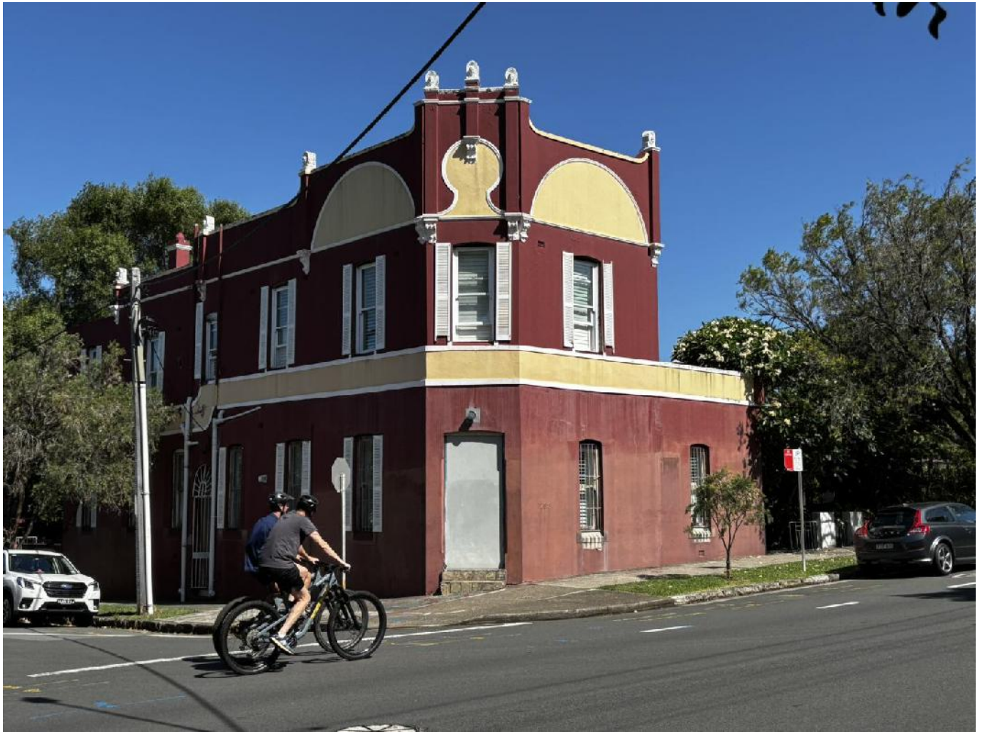
Figure 16 Development on the south-east corner of Rosalind Street and West Street
