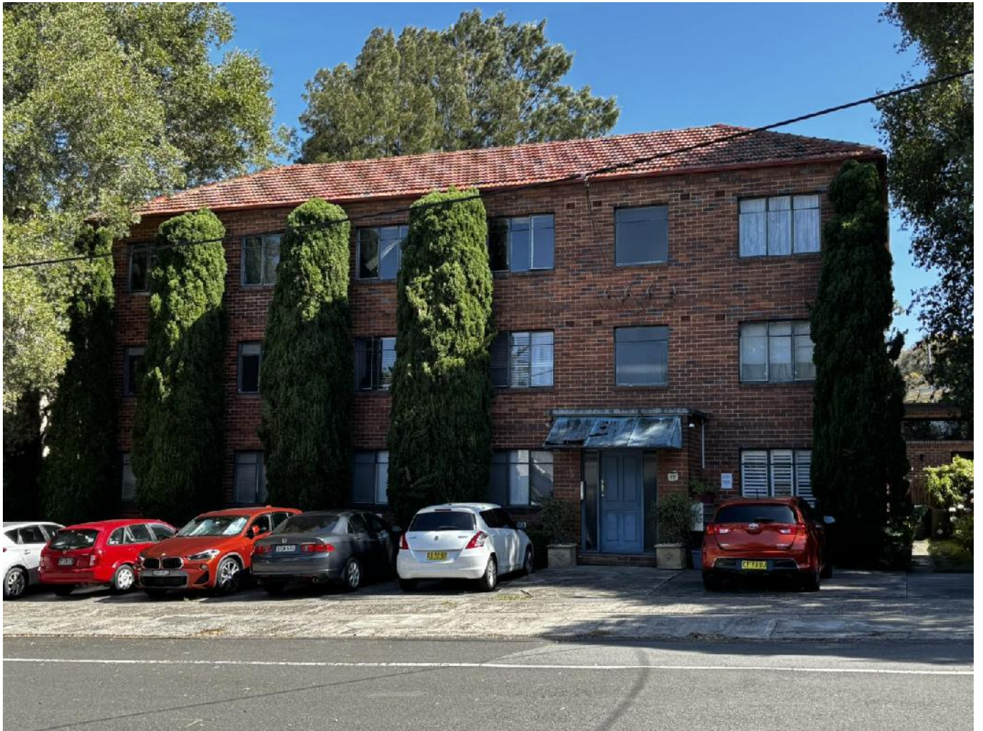
Figure 10 Adjoining development on Rosalind Street to the west
