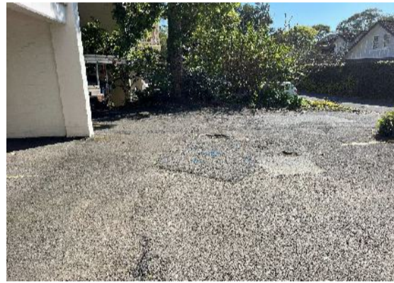
View of the driveway/carparking condition on site Looking north Inspected 02.10.2025
