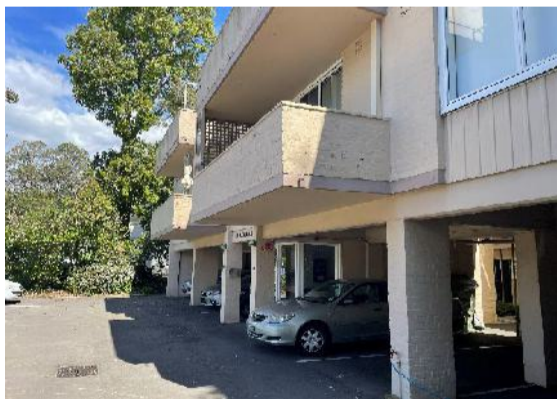
View of apartment building on No. 23 & carparking areas under the dwelling Looking south Inspected 02.10.2025
