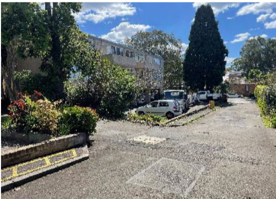
View of sealed driveway along the eastern boundary Looking north Inspected 02.10.2025
