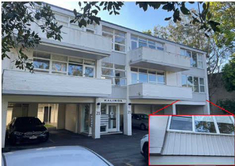
NS3: Front Facia Cladding – All buildings 19-23 Rosalind Street Exterior
