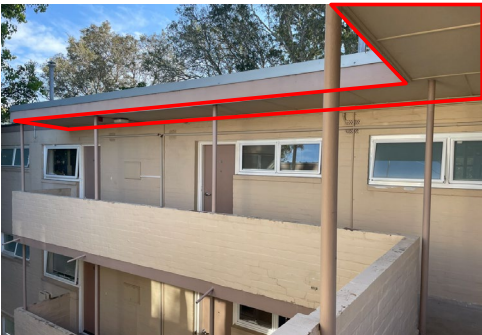
NS4: Top floor awnings – All buildings 19-23 Rosalind Street Panels
