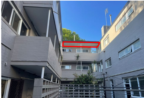
NS4: Top floor awnings – All buildings 19-23 Rosalind Street Panels
