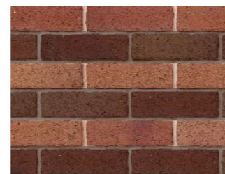
BK-02 RED BRICK TINTED MORTAR LINEAR RECESS
