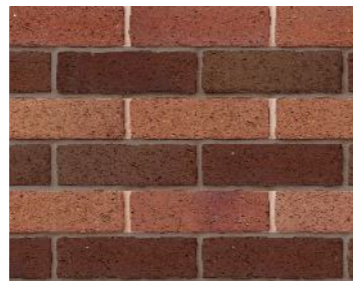
BK-02 RED BRICK TINTED MORTAR LINEAR RECESS
