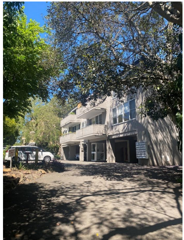
Figure 4.8: 23 Rosalind St, looking south-west
