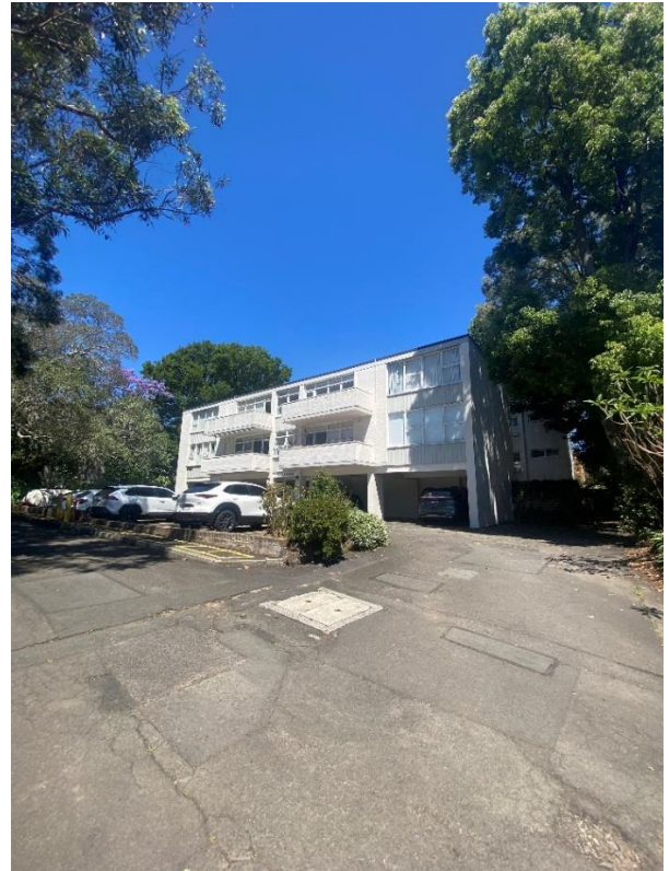
Figure 4.6: 21 Rosalind St, looking south-west
