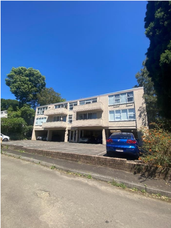
Figure 4.5: 19 Rosalind St, looking south-west
