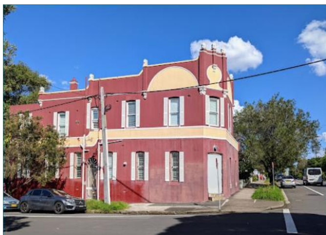
Figure 2.3: View of 205 West Street from Rosalind Street, Crows Nest. Source: Google Streetview, accessed 2025.
