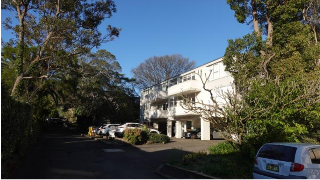
Figure 1.3 –Existing site conditions illustrating the existing 3 storey 'walkup' units and undercroft parking. There are variety of scattered trees amongst the unit blocks, most of which are undesirable species or small and insignificant trees (Photo: Arterra 28/8/25)
