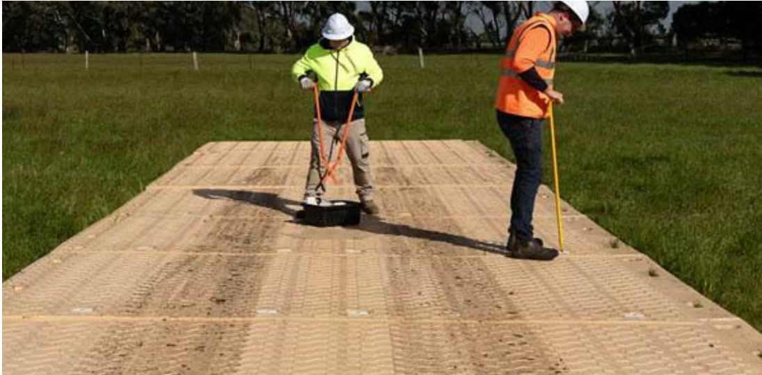
Figure 3.2 – Example of acceptable Tree Protection Area ground protection (Source: Samson/Envirex)
