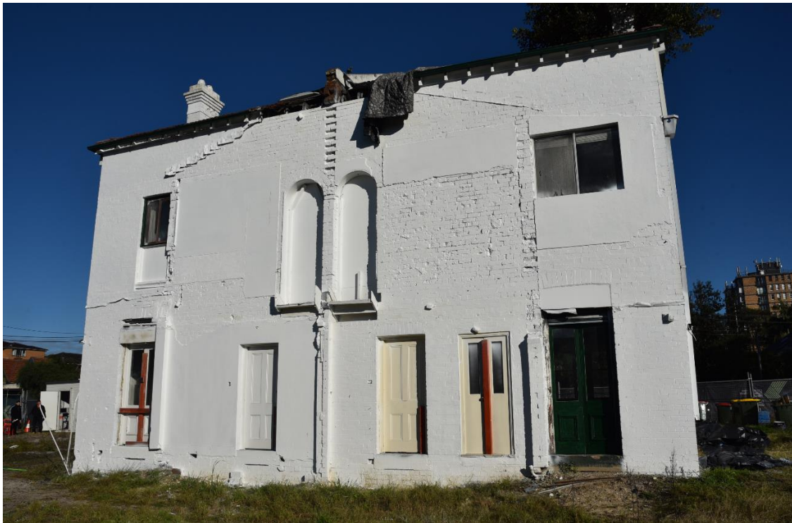
Figure 12: View towards the rear elevation of the heritage item. Note intrusive fenestration and damage from previous additions and modifications.
