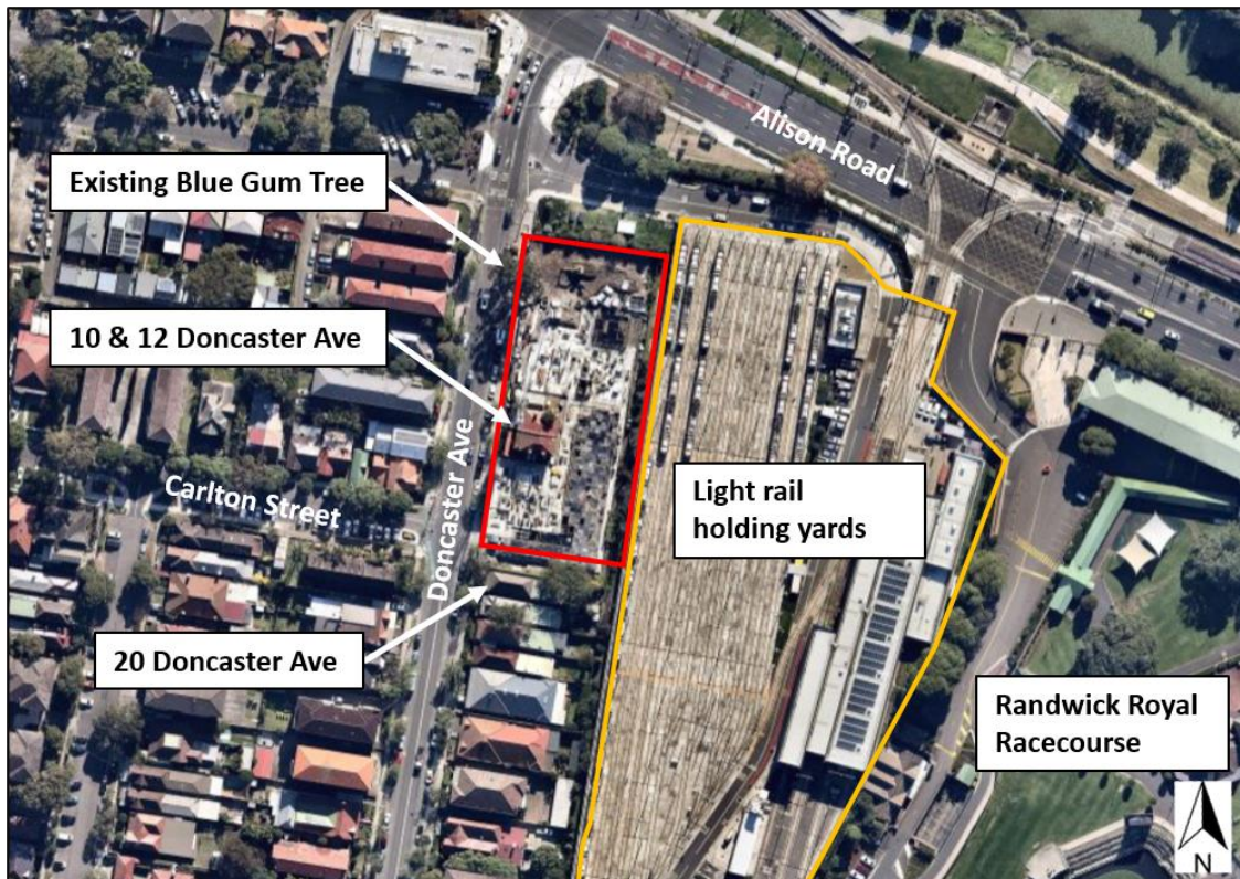
Figure 1 | Aerial view of the site and surroundings – site shown in red outline (Base source: Nearmap)
