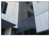
10. FRONT GLAZED GREY BODY TINT GLASS WITH SHADOW BOX SPANDREL PANEL, DULUX DURALLOY MONUMENT MATT FINISH TO FRAMES.
