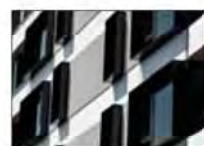
4. POWDER COATED FOLDED ALUMINIUM WITH DULUX DURALLOY SHADOW BOX SPANDEL PANEL, MONUMENT MATT FINISH.
