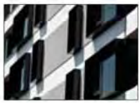
4. POWDER COATED FOLDED ALUMINIUM WITH DULUX DURALLOY MONUMENT MATT FINISH.
