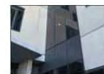
10. FRONT GLAZED GREY BODY TINT GLASS WITH SHADOW BOX SPANDEL PANEL, DULUX DURALLOY MONUMENT MATT FINISH TO FRAMES.
