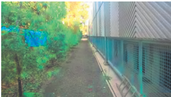
3. View to the North along TfNSW easement
