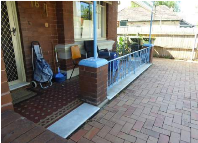
Figure 3.28 16 Doncaster Avenue, showing unsympathetic metal verandah posts and railing, non-original tiles and garden paving.
