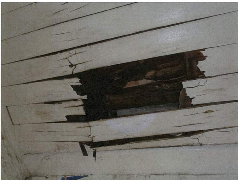
Roof and ceiling decay over entry
