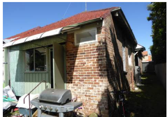
Figure 3.33 Rear of 14 Doncaster Avenue, showing changes to the brickwork and window opening, with unsympathetic cladding and aluminium framed window, showing rear details.
