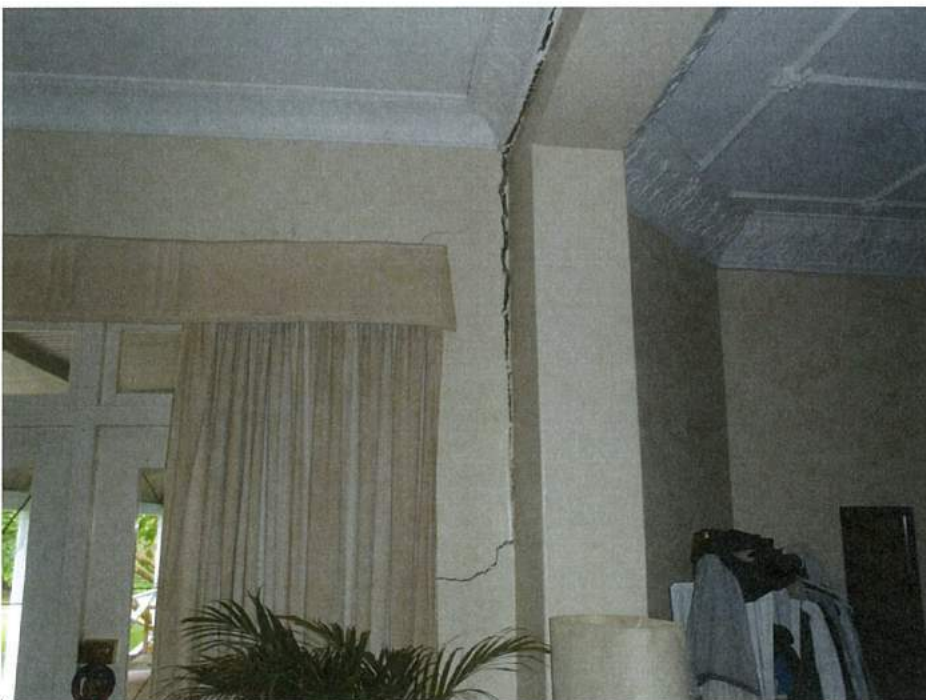
East wall of north wing showing ceiling separation at beam and severe cracking in wall
