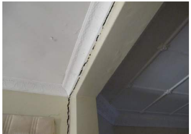
Figure 3.14 Detail of interior showing cracking and ceiling separation at beam.
