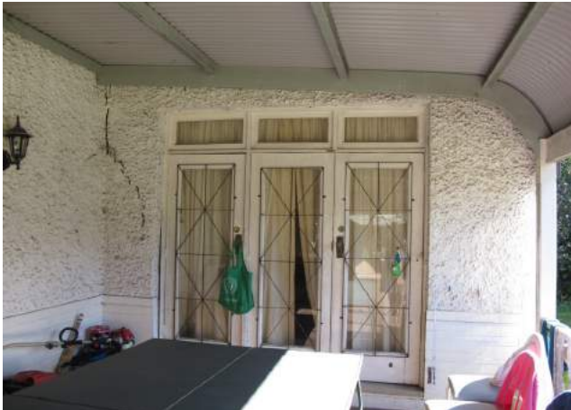
Figure 3.11 Detail showing as example of the cracking to the exterior of 4 Doncaster Avenue.
