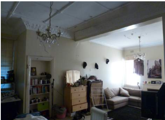
Figure 3.13 The living area within 4-8 Doncaster Avenue. Decorative plaster ceilings and cornices are visible in the foreground. A large structural beam illustrates where the dwelling was extended and associated cracking.
