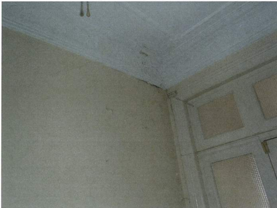
Damp penetration near entry
