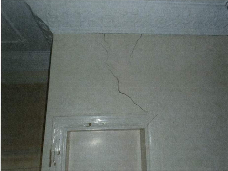
Cracking in west wall of north wing. Note also termite damage in joinery
