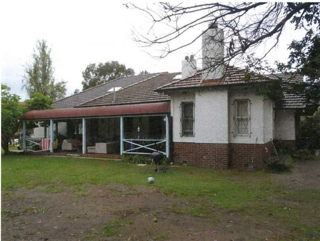
View of the building from the north. The north wing, which has rotated is on the right of the picture.
