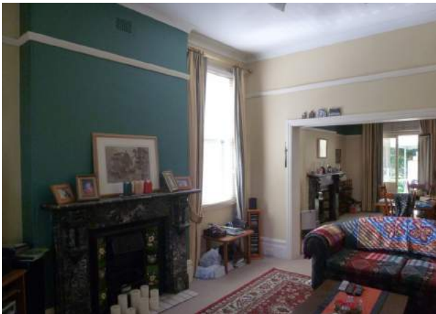
Figure 3.22 The living area in the semi detached terrace at 10 Doncaster Avenue. The fire place and its marble surround and the timber skirting are still intact. Ceilings and cornices have been replaced.
