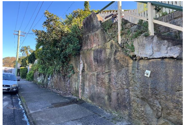
Picture 2 Rock wall along Rangers Avenue, stairs to 23 Rangers Avenue being retained.
