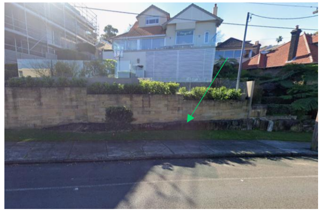
Picture 34 11 Rangers Avenue Rock Wall highlighted with green arrow.
