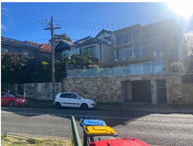
Picture 3 13 Rangers Avenue where no rock wall is present.
