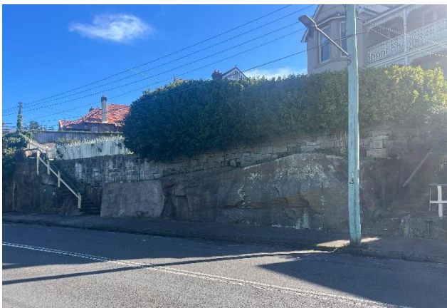
Picture 1 The significant rock wall along Rangers Avenue, 21 Rangers Avenue being retained.
