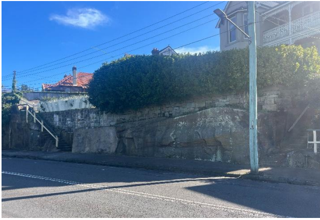
Picture 31 The significant rock wall along Rangers Avenue, 21 Rangers Avenue being retained.
