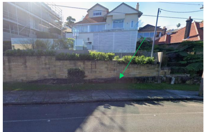
Picture 4 11 Rangers Avenue Rock Wall highlighted with green arrow.
