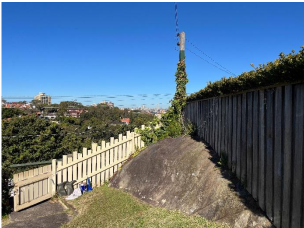
Picture 22 Rock wall in the south-west corner of 23 Rangers Avenue.
