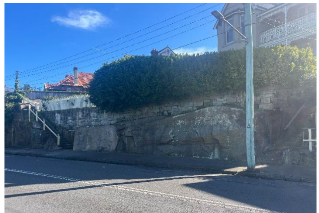
Picture 19 The significant rock wall along Rangers Avenue, 21 Rangers Avenue above.
