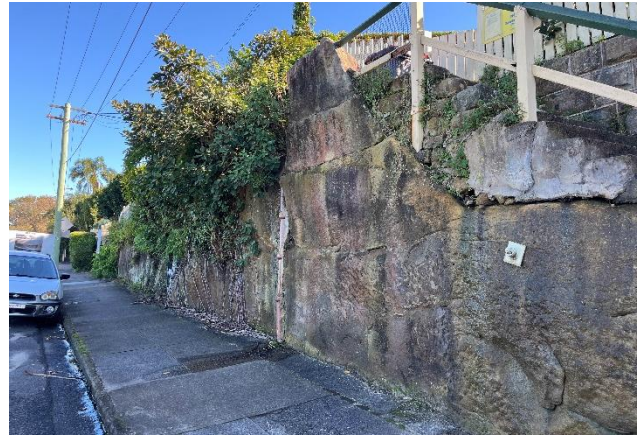
Picture 32 Rock wall along Rangers Avenue, stairs to 23 Rangers Avenue being retained.
