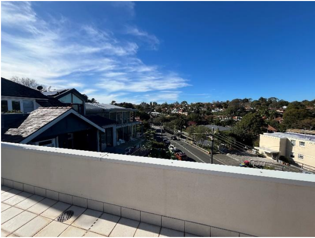
Picture 8 View to the east from the upper level of 21 Rangers Avenue.
