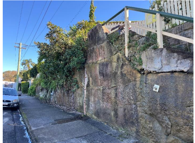
Picture 21 Rock wall along Rangers Avenue, stairs to 23 Rangers Avenue to the left.
