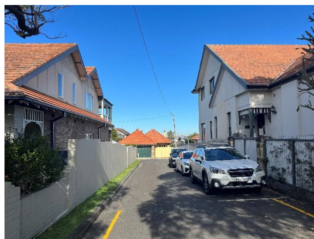
Picture 7 Looking down Bardwell Lane, example of more houses within the HCA.
