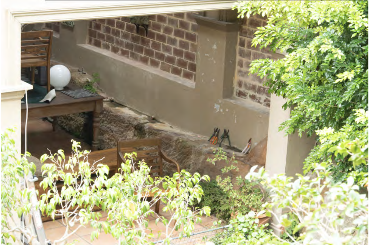
Image 9: Existing dwellings were built directly on bedrock.
