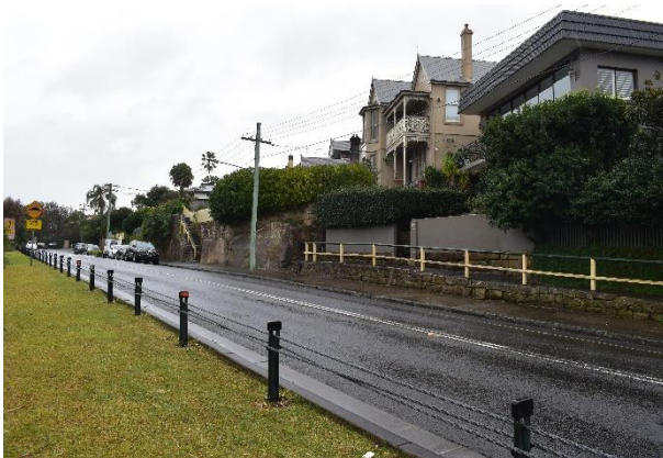
Figure 13: Slope cuts in the natural sandstone and terracing (northwest view)
