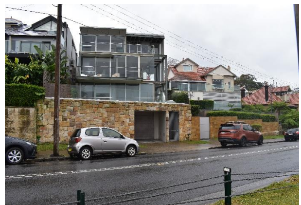
Figure 14: Slope cuts in the natural sandstone and terracing (northeast view)
