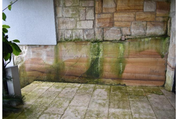
Figure 16: Natural sandstone in the front of property (No. 15) (west view)
