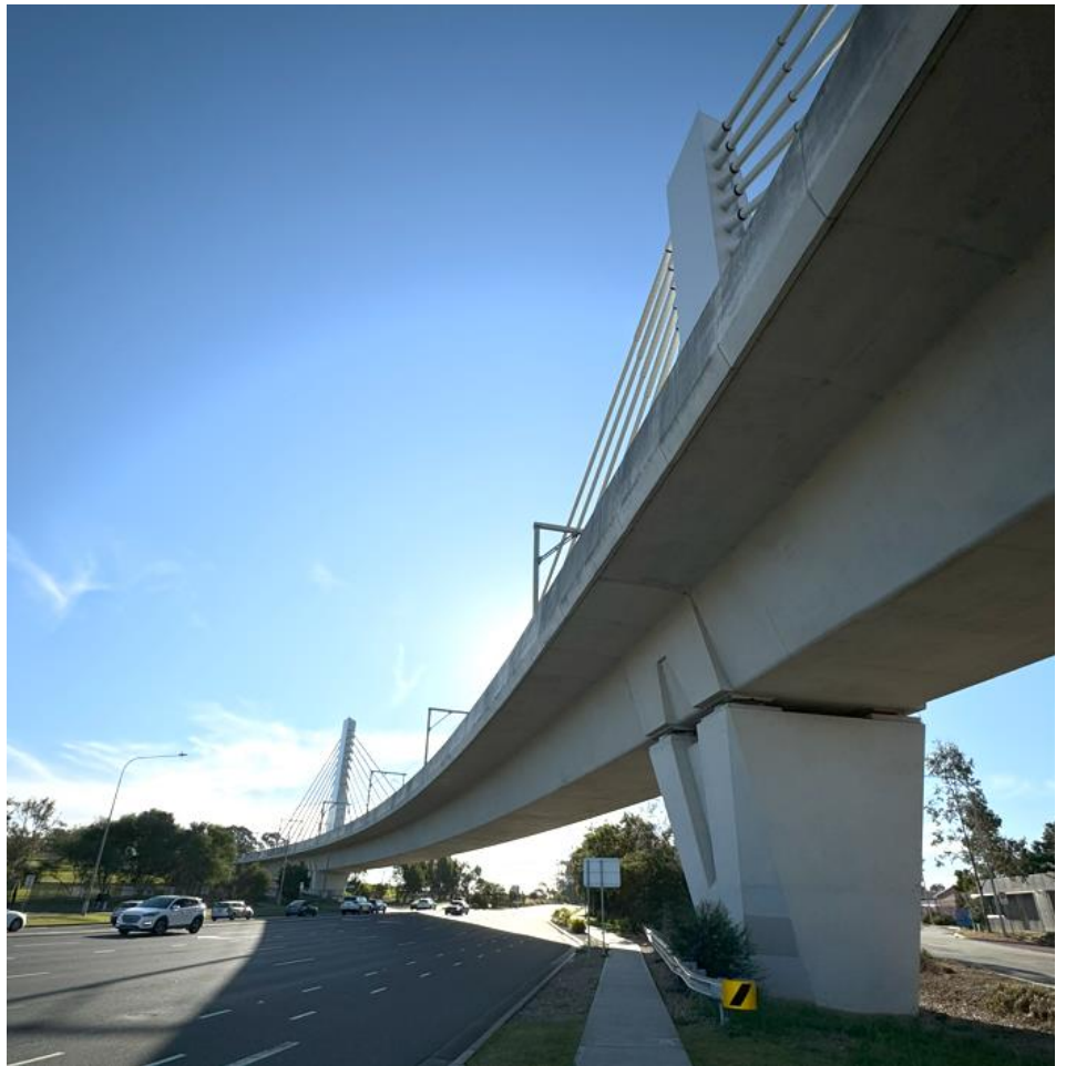
Figure 8 Adjoining development typologies – Metro bridge over Windsor Road Source: Architectus
