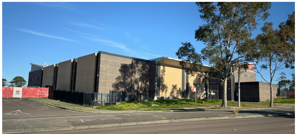
Figure 7 Adjoining development typologies – Mungerie Park zone substation Source: Architectus
