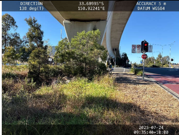
Photograph 4: Overview of the southern portion of the site, depicting the footing of the overhead Sydney Metro bridge and plant dieback noted along the edge of the bus lane to the west of the site.
