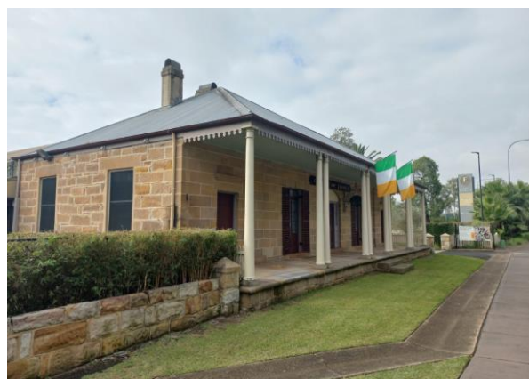
Figure 20. View to the Royal Oak Inn facing south on Windsor Road.
