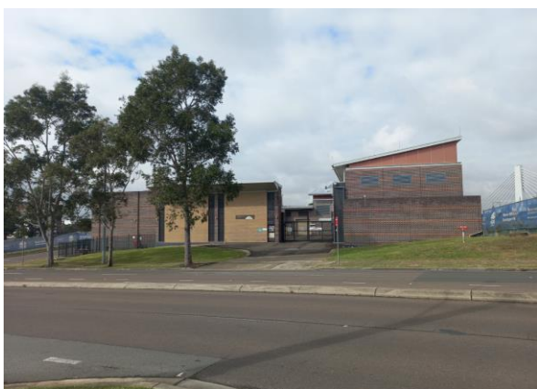
Figure 19. View to Mungerie Park Zone Substation facing south on Commercial Road.
