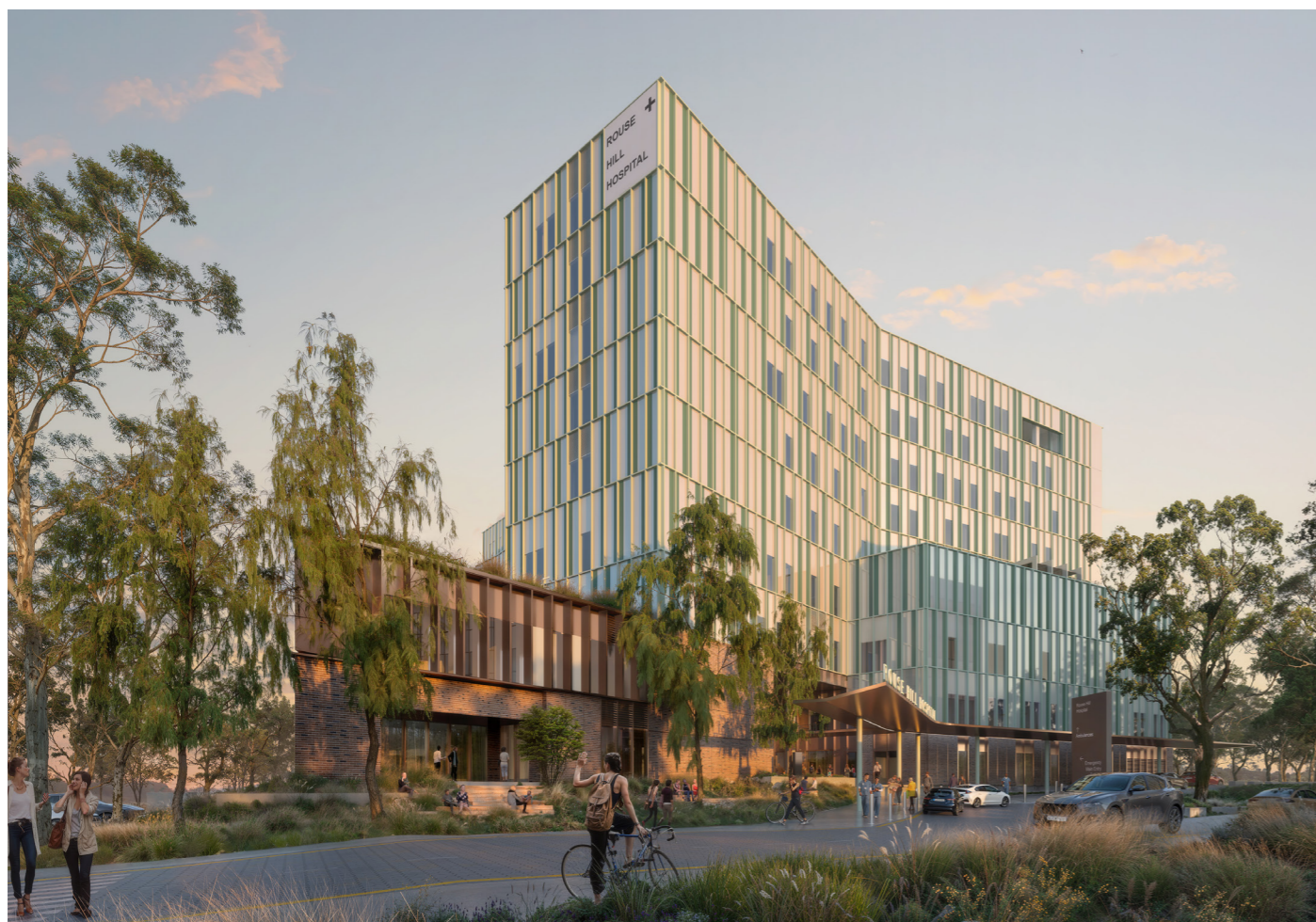
Simple uniformity of upper level facade
